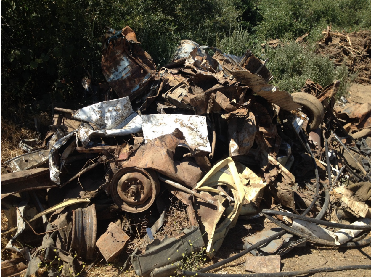
Figure 3.7-1. Debris removed during construction of the Dry Creek Habitat Enhancement Demonstration Project. June 30, 2014.
