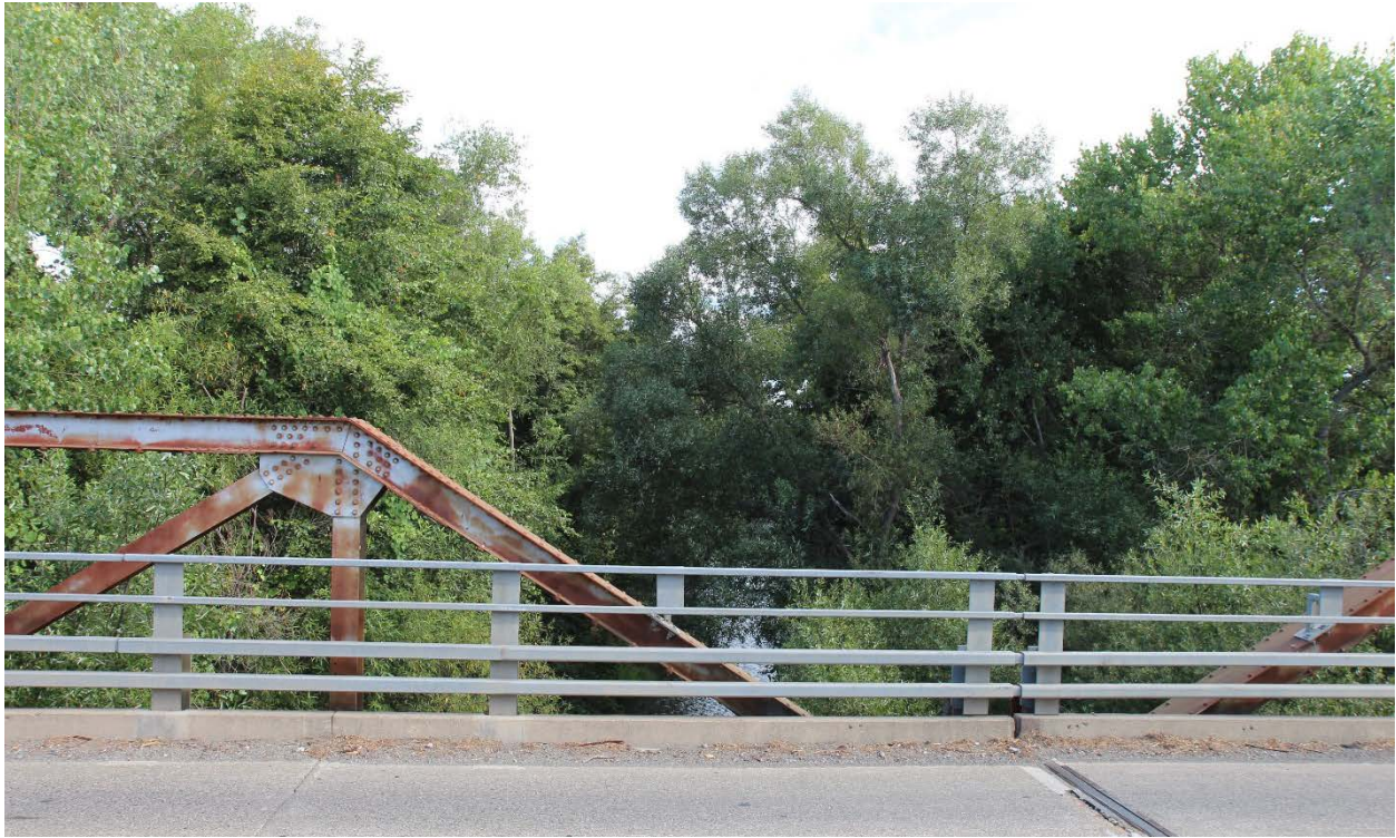
Figure 3.1.9. View of Dry Creek from Westside Bridge looking upstream. July 7, 2015.
