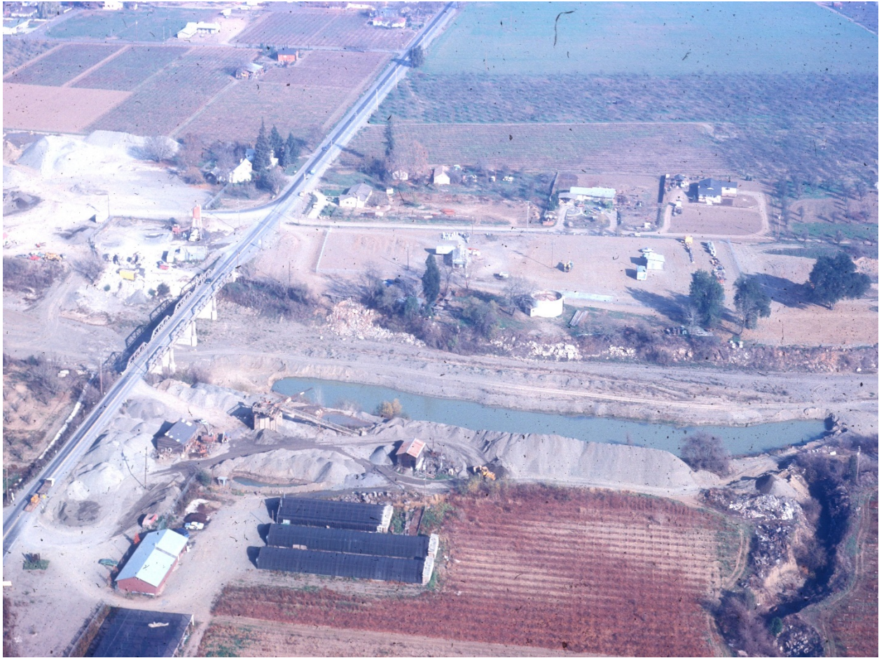
Figure 3.7-2. Dry Creek at Westside Road Bridge with areas of concrete debris visible along the upper banks. December 17, 1976.
