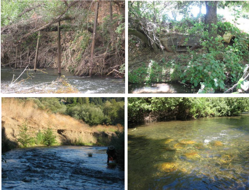
Figure 6: (upper left) Failed I-beam and chainlink fence stabilization efforts, (upper right) car bodies in the banks, (lower left) erosion along an outside bend, (lower right) a triangular boulder cluster in Dry Creek.
