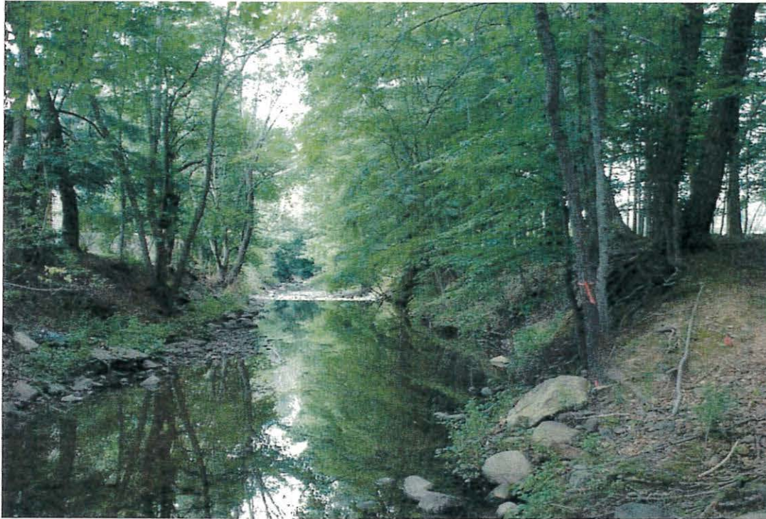
PHOTO #3 – View looking Northeast towards concrete encased sanitary sewer that crosses the Peckman River, nearest to the Verona Wastewater Treatment Plant. Photo Date: 07/12/2017.
