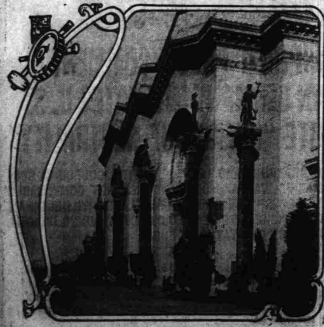
Facade of 1915 Exposition's Huge Palace of Machinery
