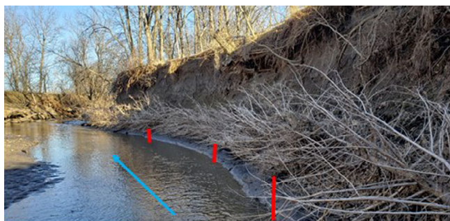
FIGURE 5 Channel bed degradation on Wolfley Creek Cedar tree revetment April 2017 (Nassar, 2019). Red lines indicate channel degradation. Blue line indicates flow direction [Color figure can be viewed at wileyonlinelibrary.com ]
