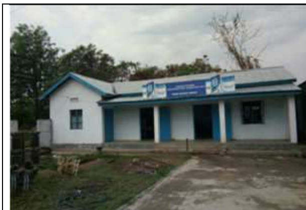
Photo 3: Existing Umrangso Substation
