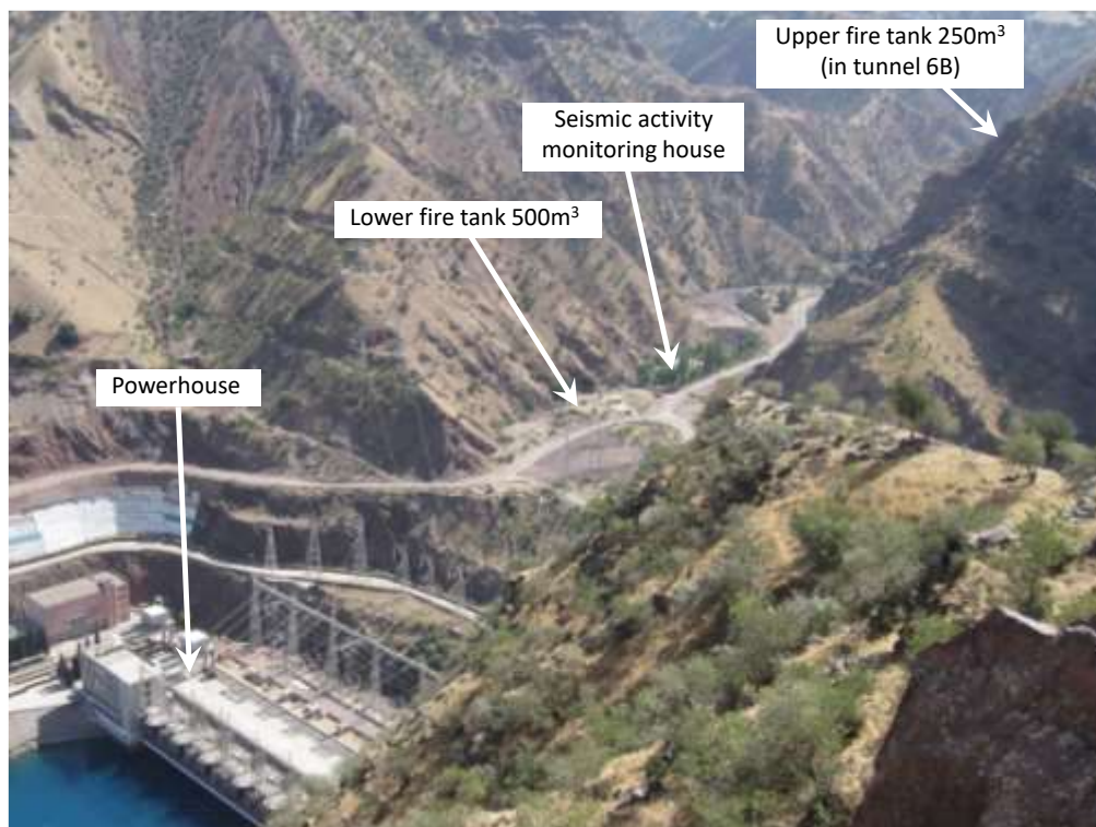
Figure 5. Nurek HPP complex (view from above powerhouse)
