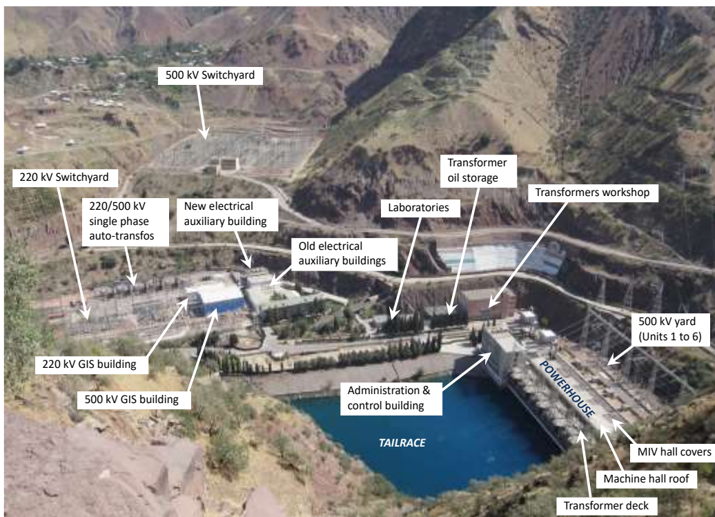
Figure 4. Nurek HPP complex (view from downstream right bank)
