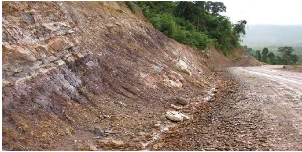
Figure 6.2 Water Drainage Channel Provided along an Elevated Unpaved Road
