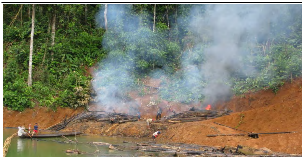
Figure 6.1 Wet Weather Affecting the Clearing Process
