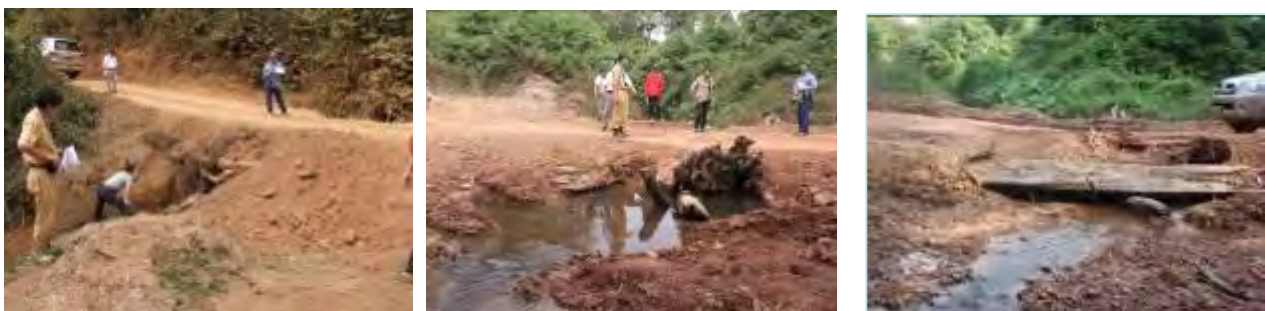
Figure-5 Small stream in dry season before the Works
