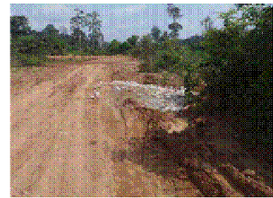
Sta. 17+200_Drainage improvement by gravel filling
