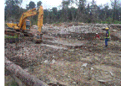
Km 16+00 Quarry Settlement pond installation
