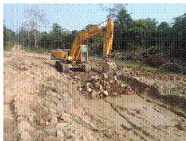
Sta. 22+200 Road improvement by gravel filling
