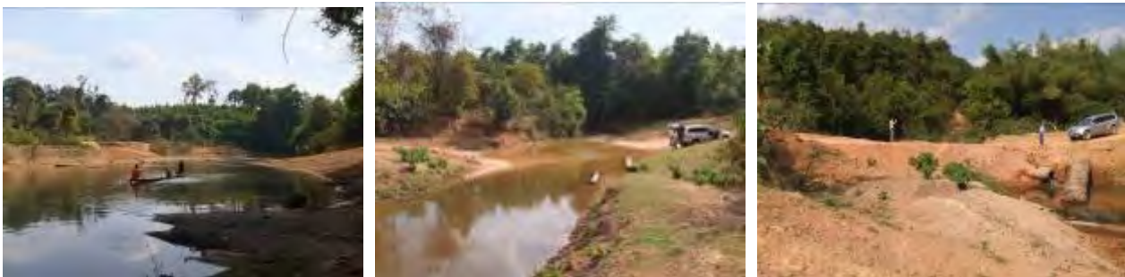
Figure-4 Nam Xao, Nam Thak and Nam Miang (from left side) before the Works
