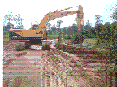
Sta. 17+200_Drainage improvement by gravel filling
