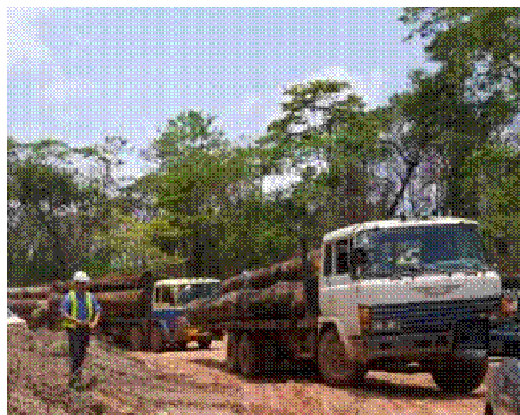
Figure-13 Timber truck on site on 22 May 2013 which is not related with road rehabilitation works of NNP1PC
