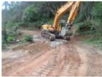
Sta. 15+200 Road improvement by Gravel filling
