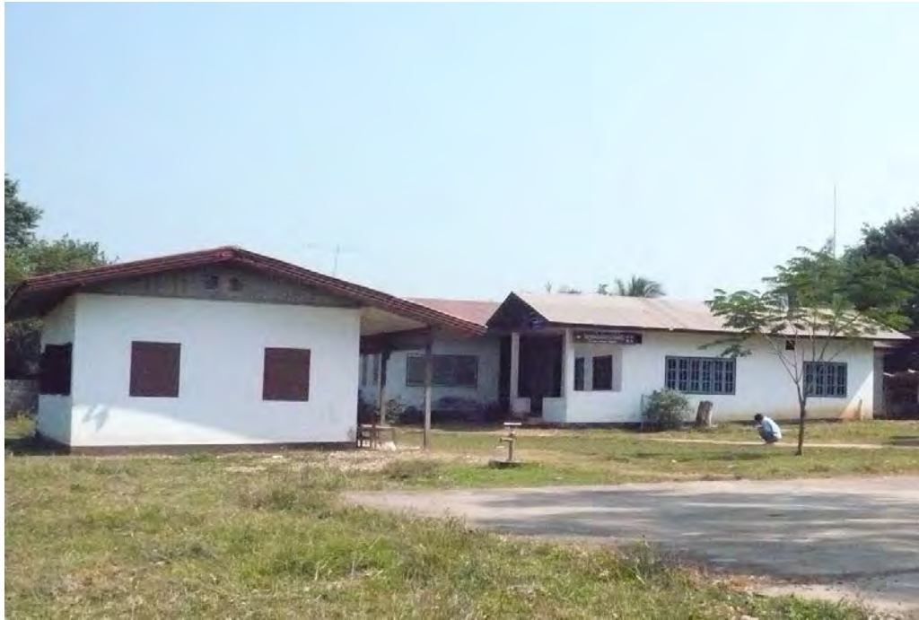
Figure 3.10 Bolikhan district hospital
