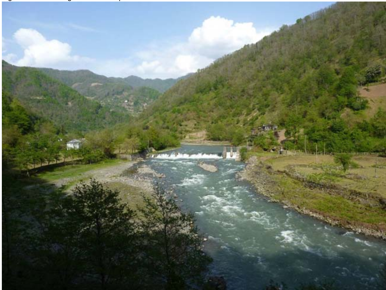
Figure 2.4: Existing Machakhlistsqali HPP Concrete Weir
