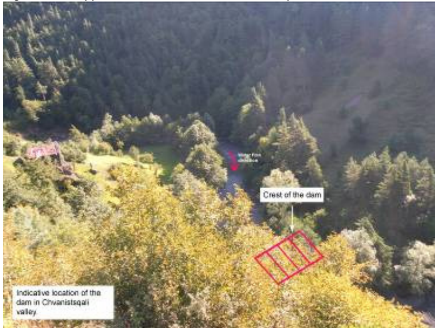
Figure 18.10: Approximate line of crest of Chvanistsqali dam
