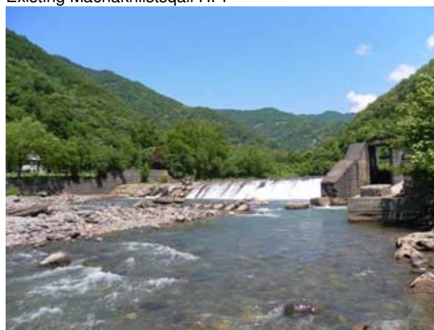
Existing Machakhlistsqali HPP
