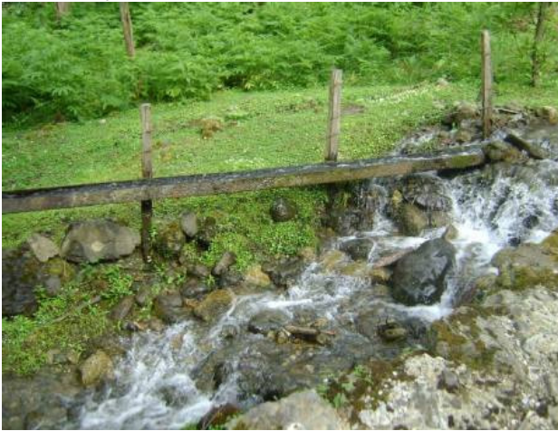
Typical Traditional Irrigation Intake Arrangements: Chvanistsqali Head
