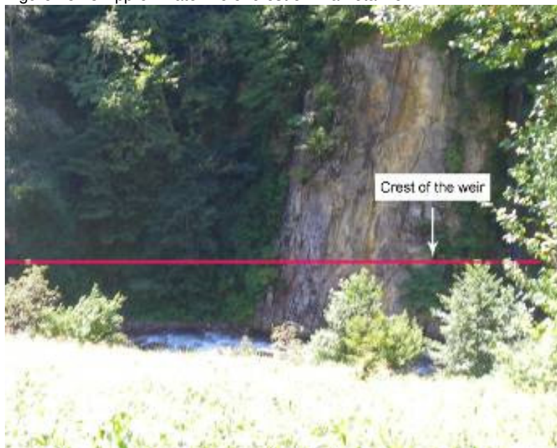
Figure 18.13: Approximate line of crest of Akavreta weir
