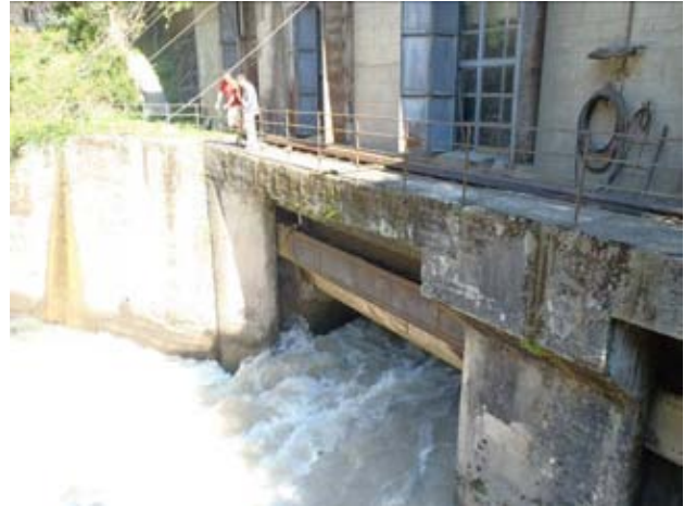
Figure 2.10: Existing Asti HPP Tailrace
