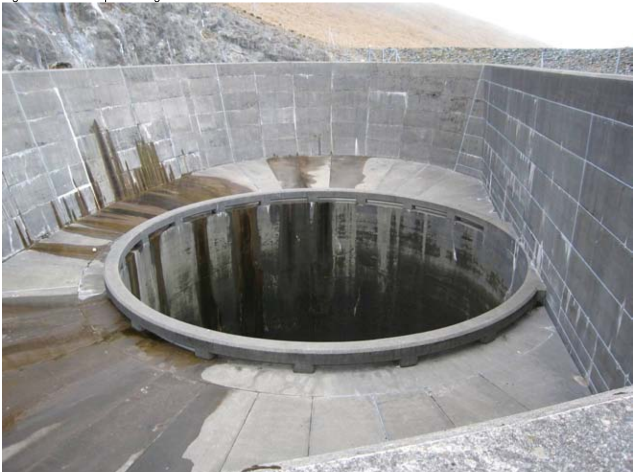
Figure 2.7: Example of surge shaft
