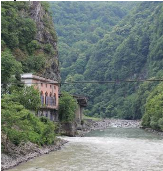
Figure 18.15:View of the existing Asti power house
