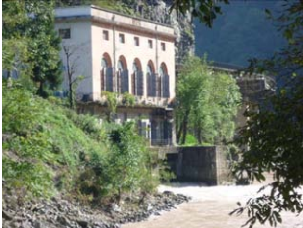
Figure 2.9: Existing Asti HPP Surface Powerhouse
