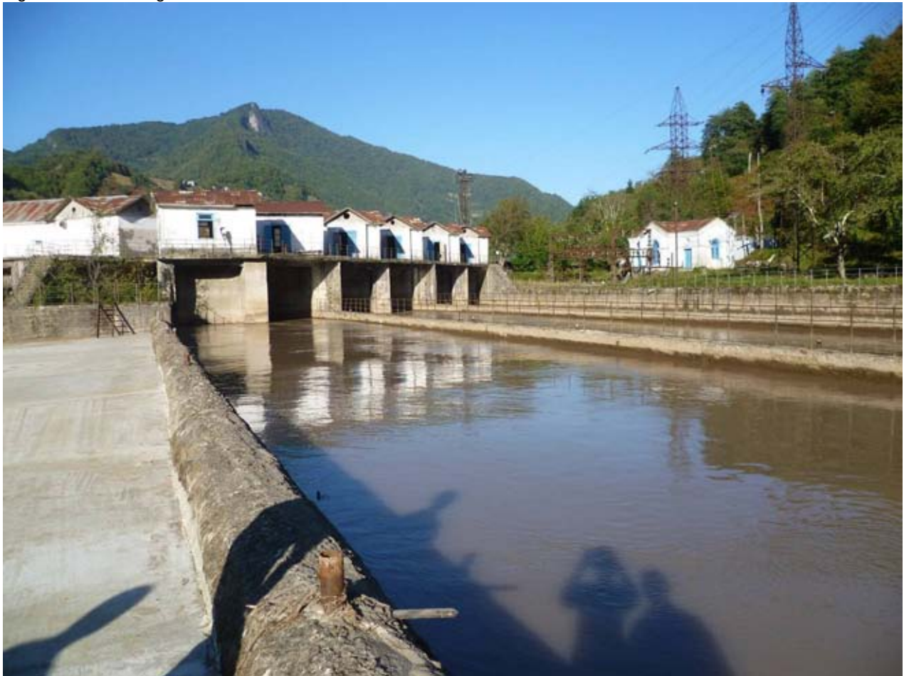
Figure 2.5: Existing Asti HPP Sediment Basin
