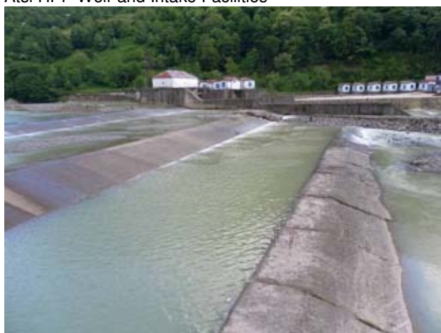
Atsi HPP Weir and Intake Facilities
