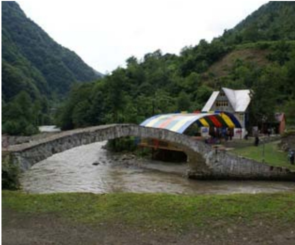
MM4 Bridge near Tskhemlara village
