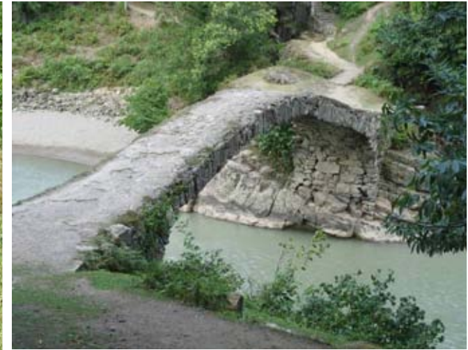
MM35 Bridge in Makhuntseti village
