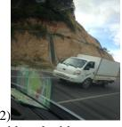
After the construction, the road was widened with two separated motorbike lanes along the two roadsides, and road surface is in good condition (1). The roadside slopes were reshaped and the horizontal and vertical drainage ditches were constructed (2). The stepped concrete embankment was constructed to stabilize the areas where landslide used to be often occurred at km 108th (3). One rest stop is provided in the area that is opposite the constructed embankment (4)
