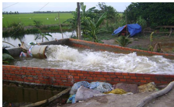
Figure 24: Pumping water from diked areas to canals in flood reason
