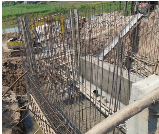
Figure 55: The construction area of culvert in the subproject
