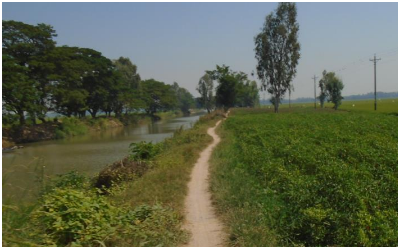
Figure 53: The existing embankment is also the trail in along Vinh Hau canal
