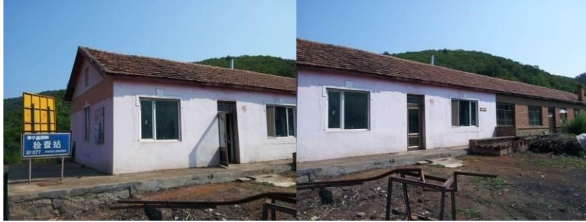
Fig.3.2-1 Site Photos of Renovated Conservation Station——Qianying Conservation Station
