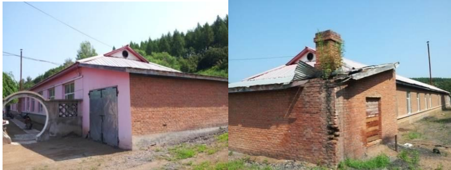
Fig.3.2-2 Site Photos of Renovated Conservation Station——Huichuan Conservation Station
