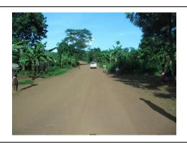
Figure 5-4: Pronounced rutting, loss of camber and lack of side drainage system
