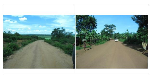
Figure 3-3: Fair condition of carriageway but side drains and bridge insufficiently maintained
