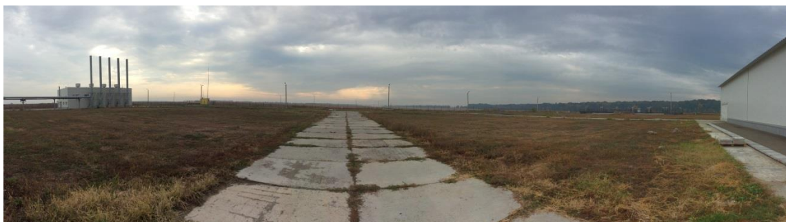
Figure 2.5 Hatchery, site for third line
