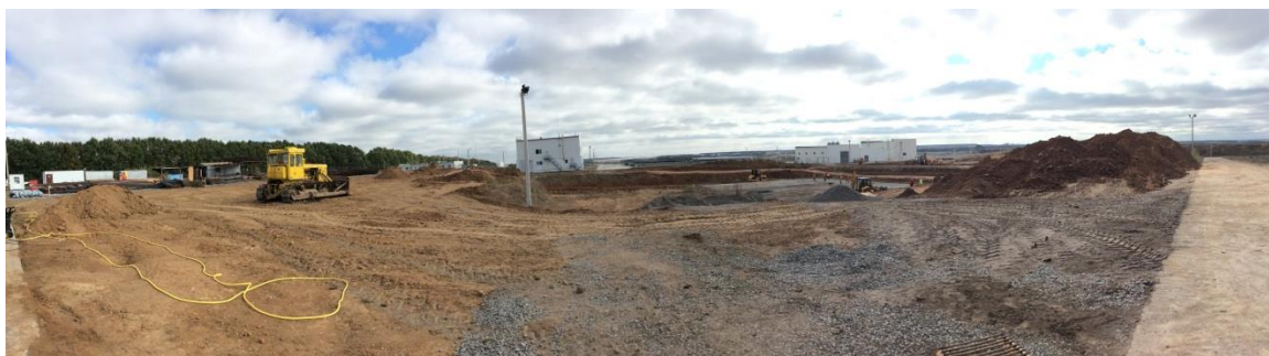
Figure 2.9 WWTP, second line (foundation-laying stage)
