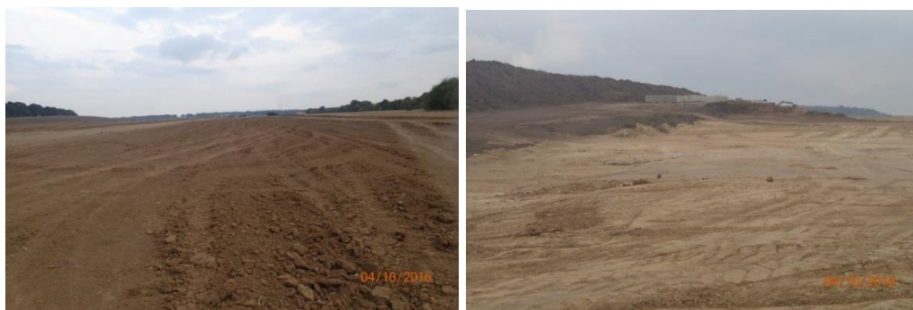
Figure 6.10 Excavation of 30 ha brigade site and topsoil stockpile berm
