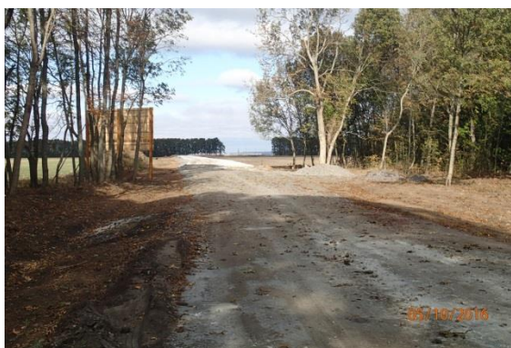
Figure 6.9 Clearing of vegetation and tress for the access road construction
