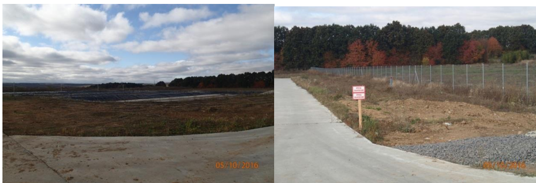
Figure 6.2 WWTP Lined sludge lagoons and groundwater monitoring well
