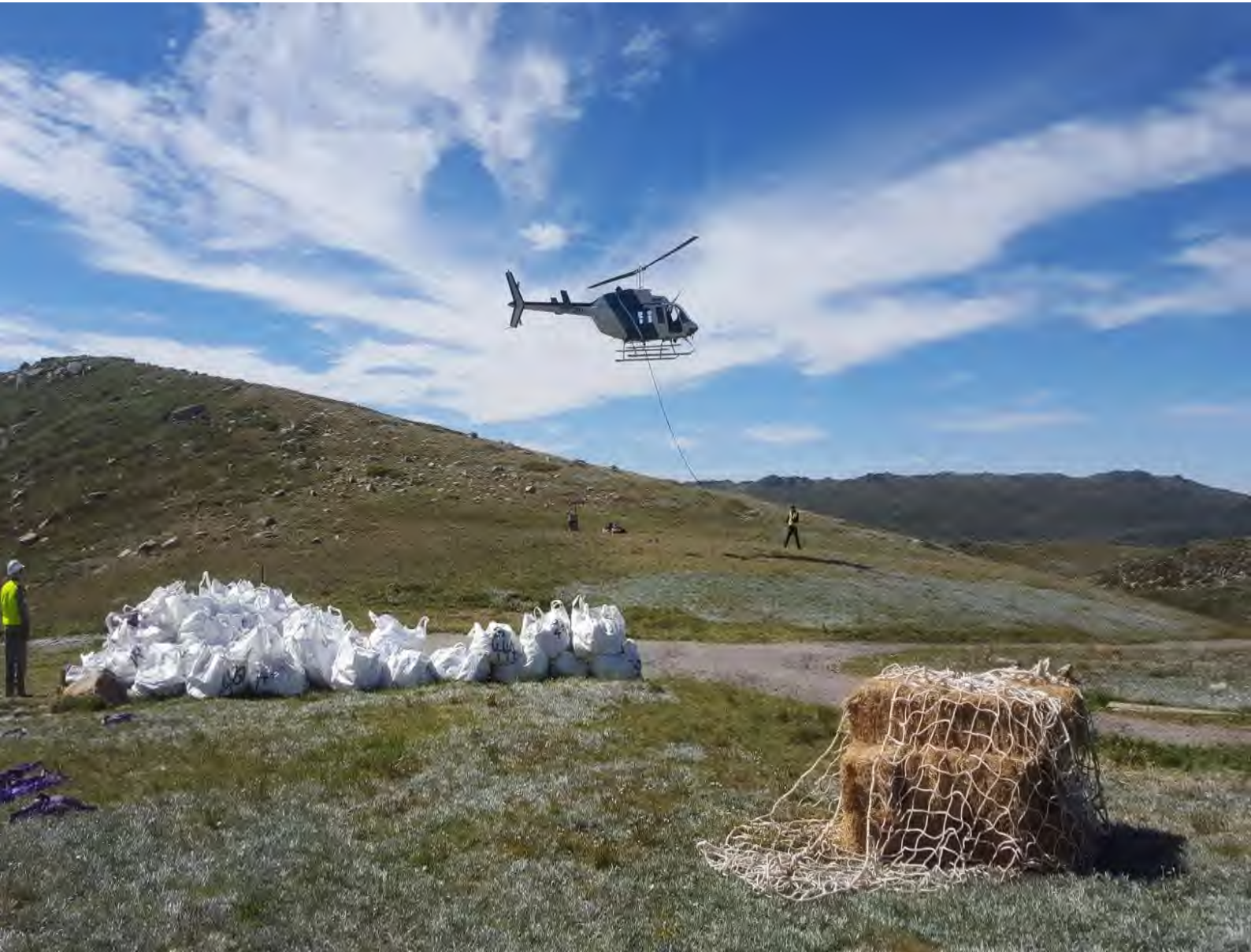
Image of Alpine trail construction (Natural Trails)
