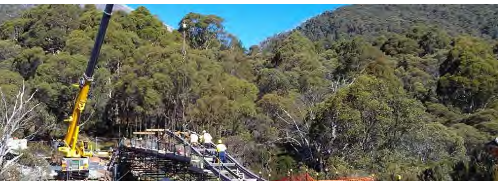
Image construction of a bridge on the Thredbo Valley Trail (Natural Trails)
