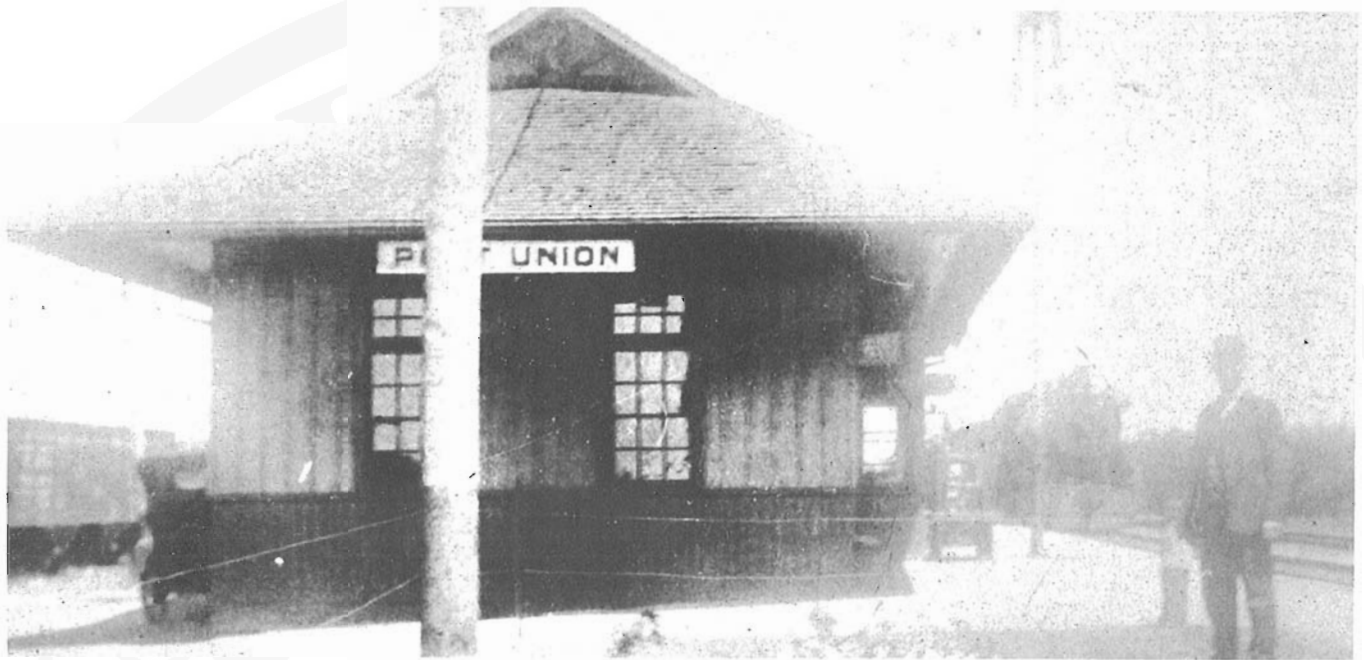
Photo Four – Port Union Station – Side View. Points of interest: a 10-Wheeler; the GTR hopper car and Model 'T' in back of the station; the semaphore position; bay window; a four-wheeled dolly. Note particularly the double track which would have been only three or four years old. The GTR began double tracking in 1887 from Montreal to Toronto. Except for a single track section of 46 miles between Port Union and Port Hope (which included Darlington – Photo 1), double tracking was not completed until 1917. My grandfather is in the foreground wearing his Grand Trunk Station Master hat. Even when it became CNR, he kept the GTR on his cap.
