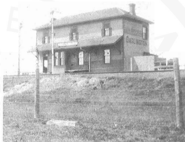
Photo One – Darlington Station – Front View. Note the two storey wooden frame construction; painted block side lettering; the semaphore signal position; a three-wheeled dolly and, single track. (Burnet Collection).
