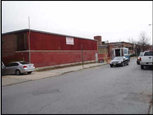
Photograph Nos. 7 and 8 – Fill port and vent pipes for gasoline and fuel oil USTs were observed off the southwestern and southern walls of the building.
