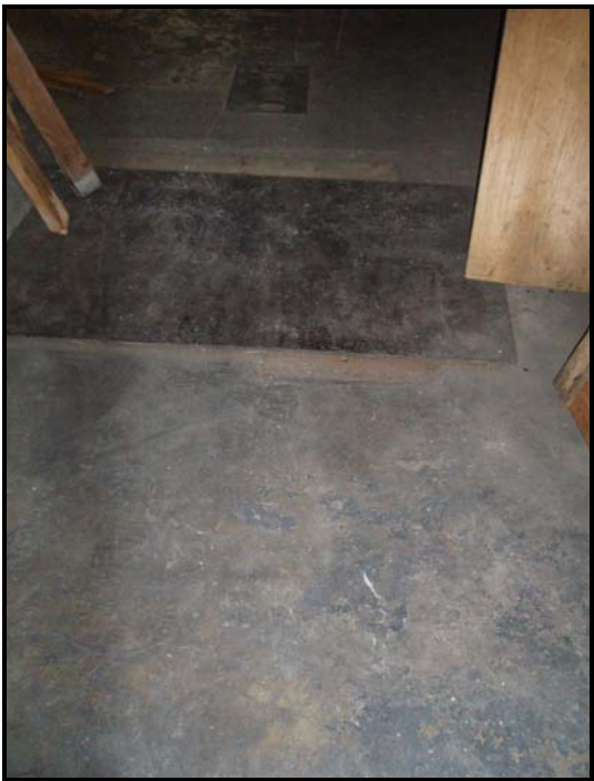
Photograph No. 9 – Steel plate within first floor of the building.
