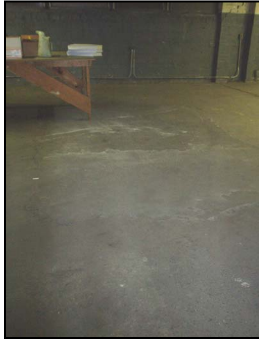
Photograph No. 10 – Concrete patch within first floor.
