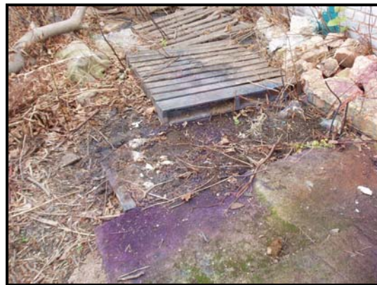
Photograph No. 11 – Staining of concrete and soil within exterior courtyard.
