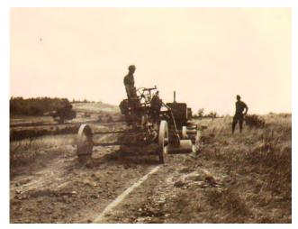
This photo was taken on July 29, 1936, of a grader being pulled by a tractor working on truck trail 202-1 by a crew out of S-123. This truck trail is still in use today, and is now the northern end of Maple Lane, and S-123 was the CCC camp located on Pine Creek Rd. Two sections of this road were relocated by the CCC, the remainder following old town road.
