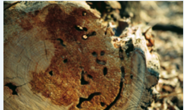
Carpenter ant damage (Joseph O' Brien, USDA Forest Service, Bugwood.org)
