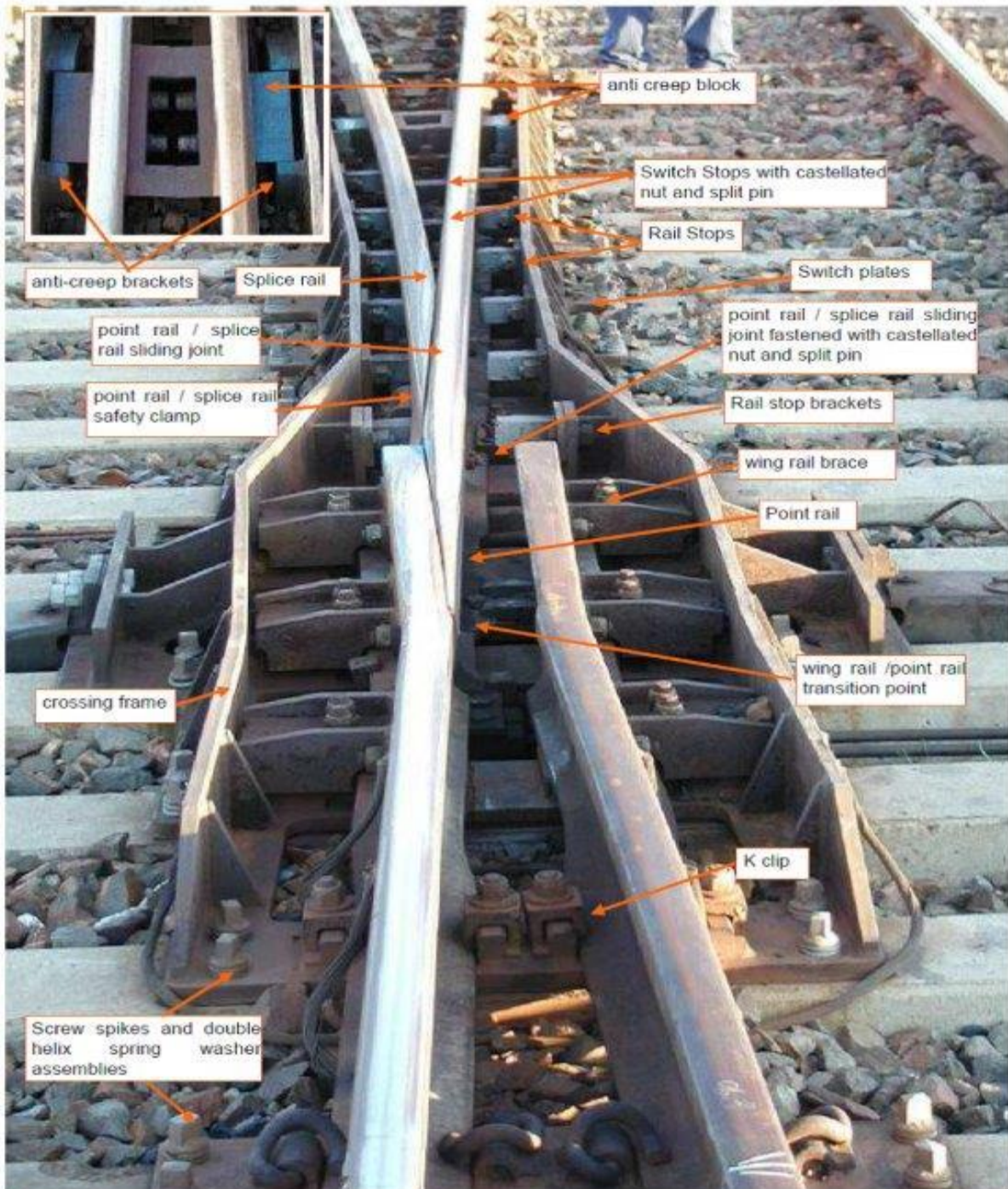
Photo 8 Typical VAE Swingnose Crossing
