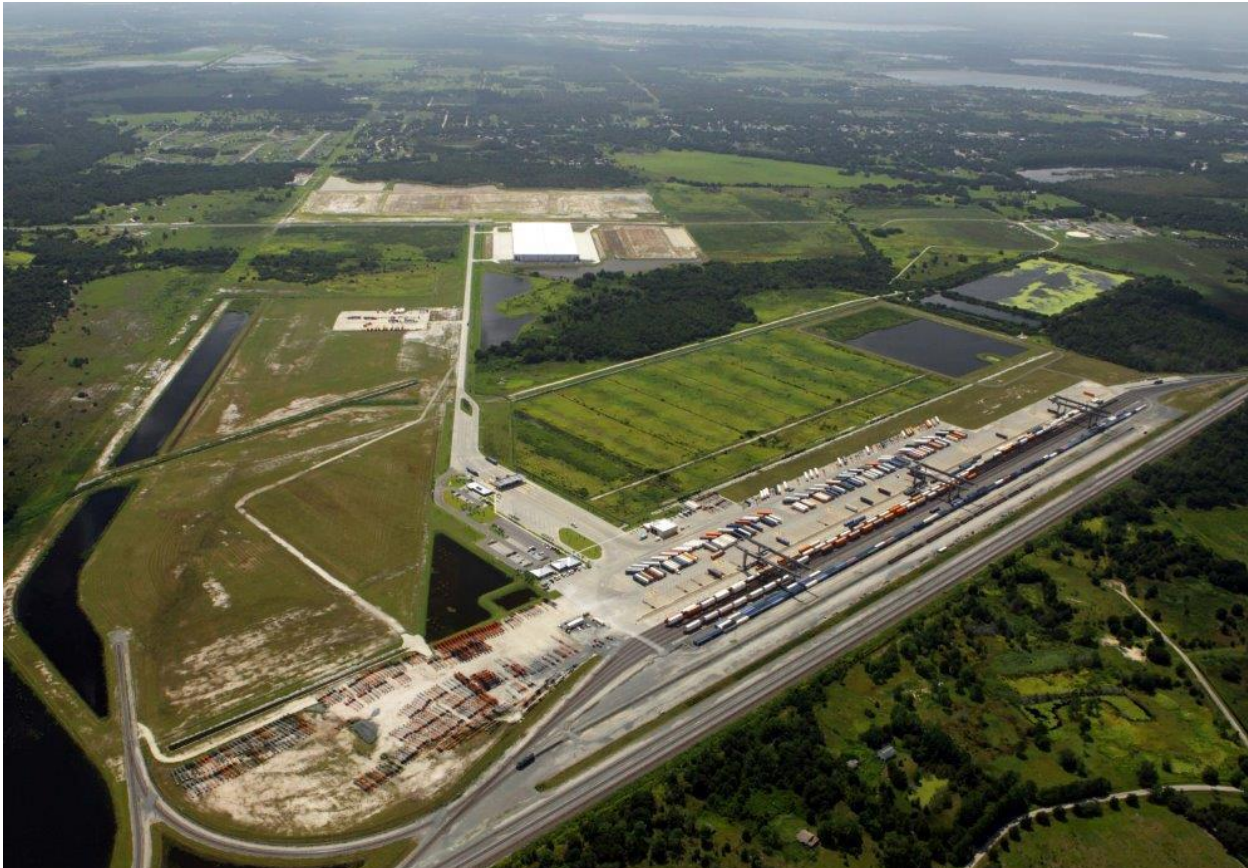
Figure 2-33 | CSX – Winter Haven ILC aerial view
