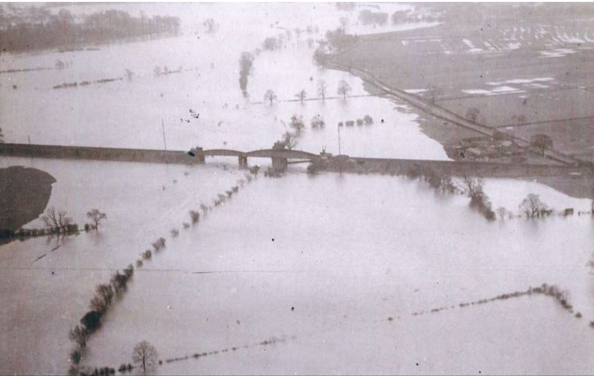
Naburn Swing Bridge 1947
