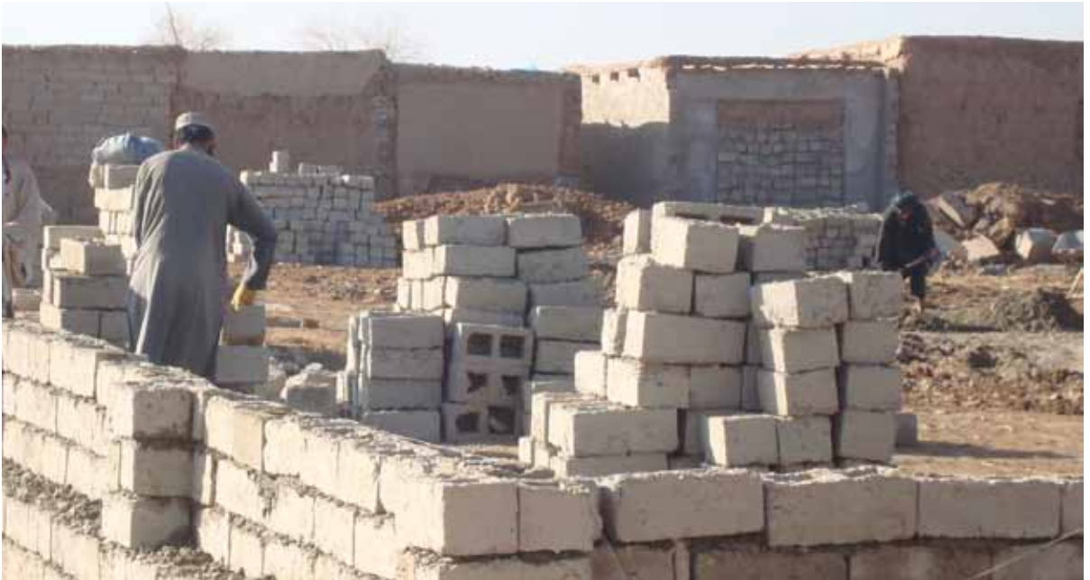
Construction of new mosque at Nad-e Ali
