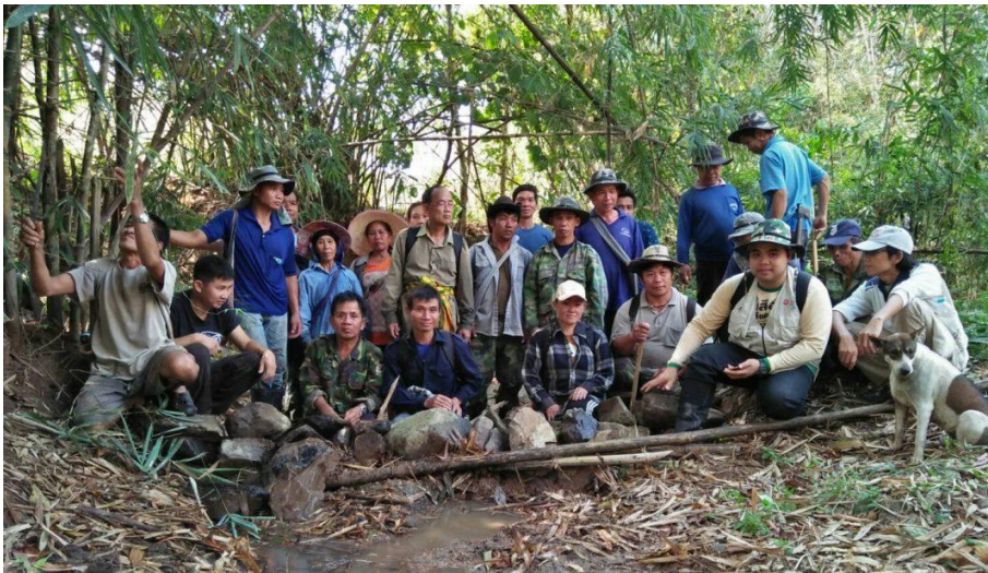
Figure 3.9 SCG Lampang and villagers building check dam
