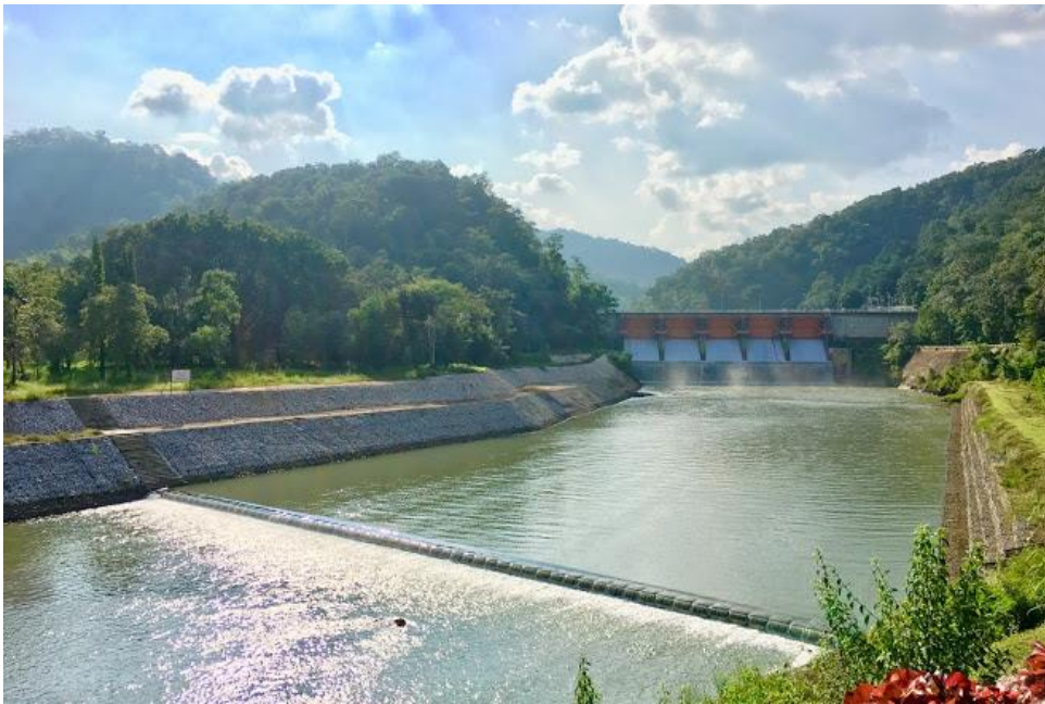
Figure 1.11 – Kiew Lom Dam, Lampang Province
