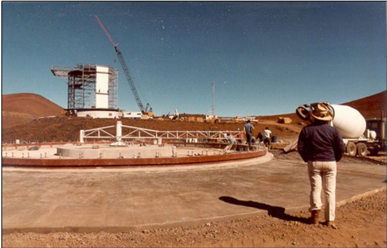
Figure 2-8 Photograph of Foundation During Construction
