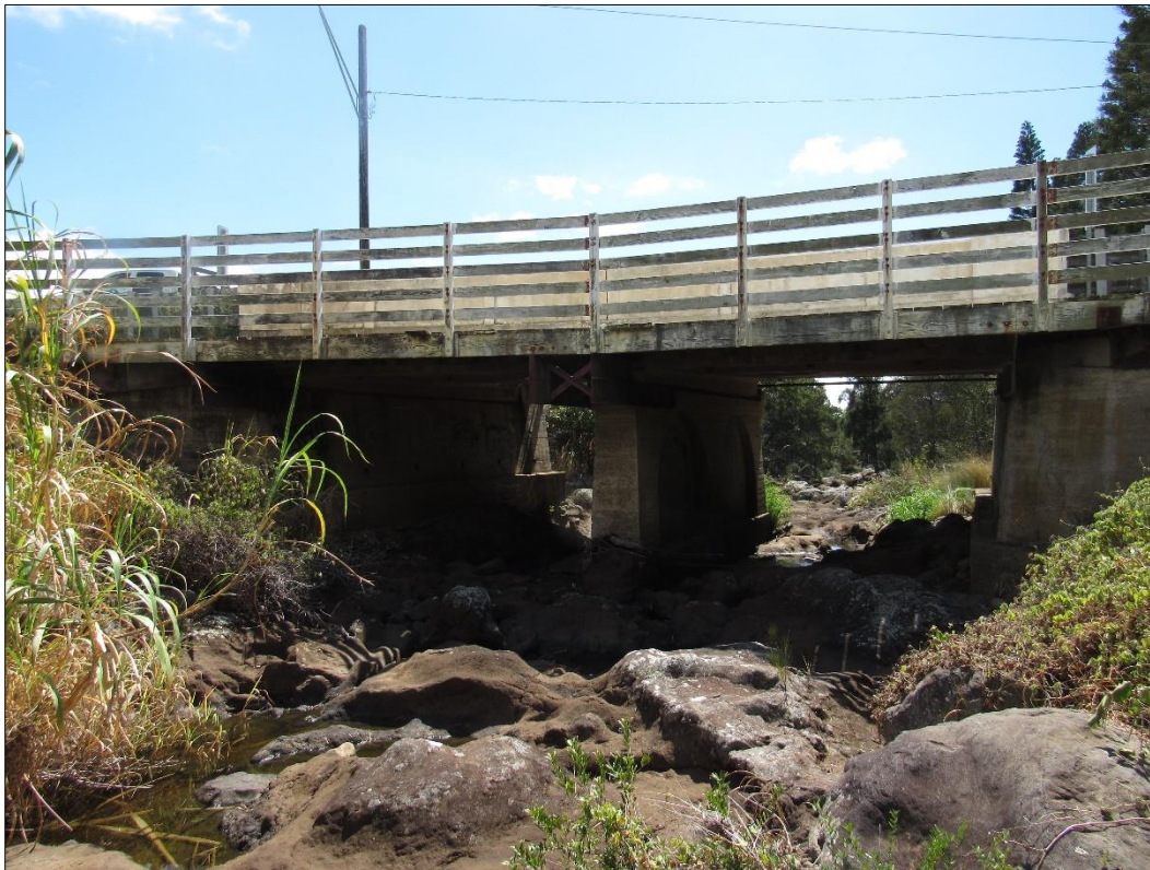
Figure 4. Waiaka Bridge, view to the southwest.
