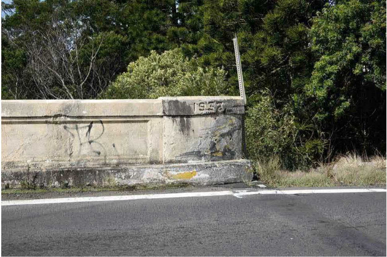
Waiaka Stream Bridge – Abutment
