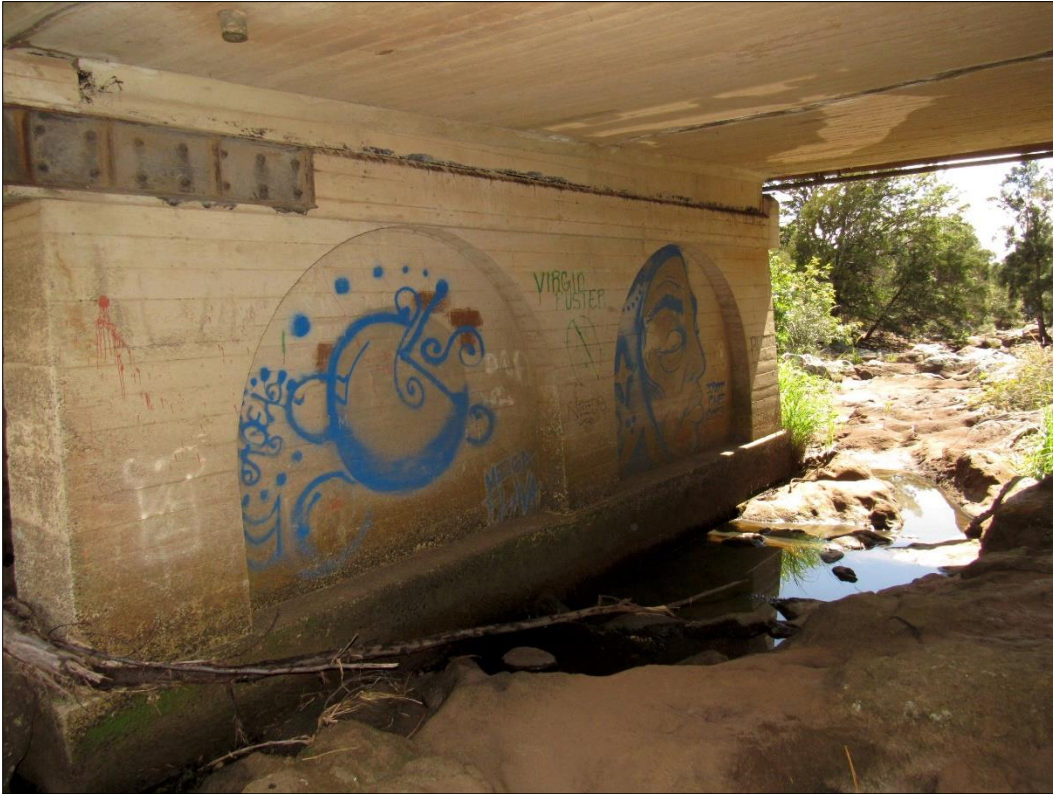
Figure 30. Site 29221 Waiaka Bridge wall pier, view to the southeast.
