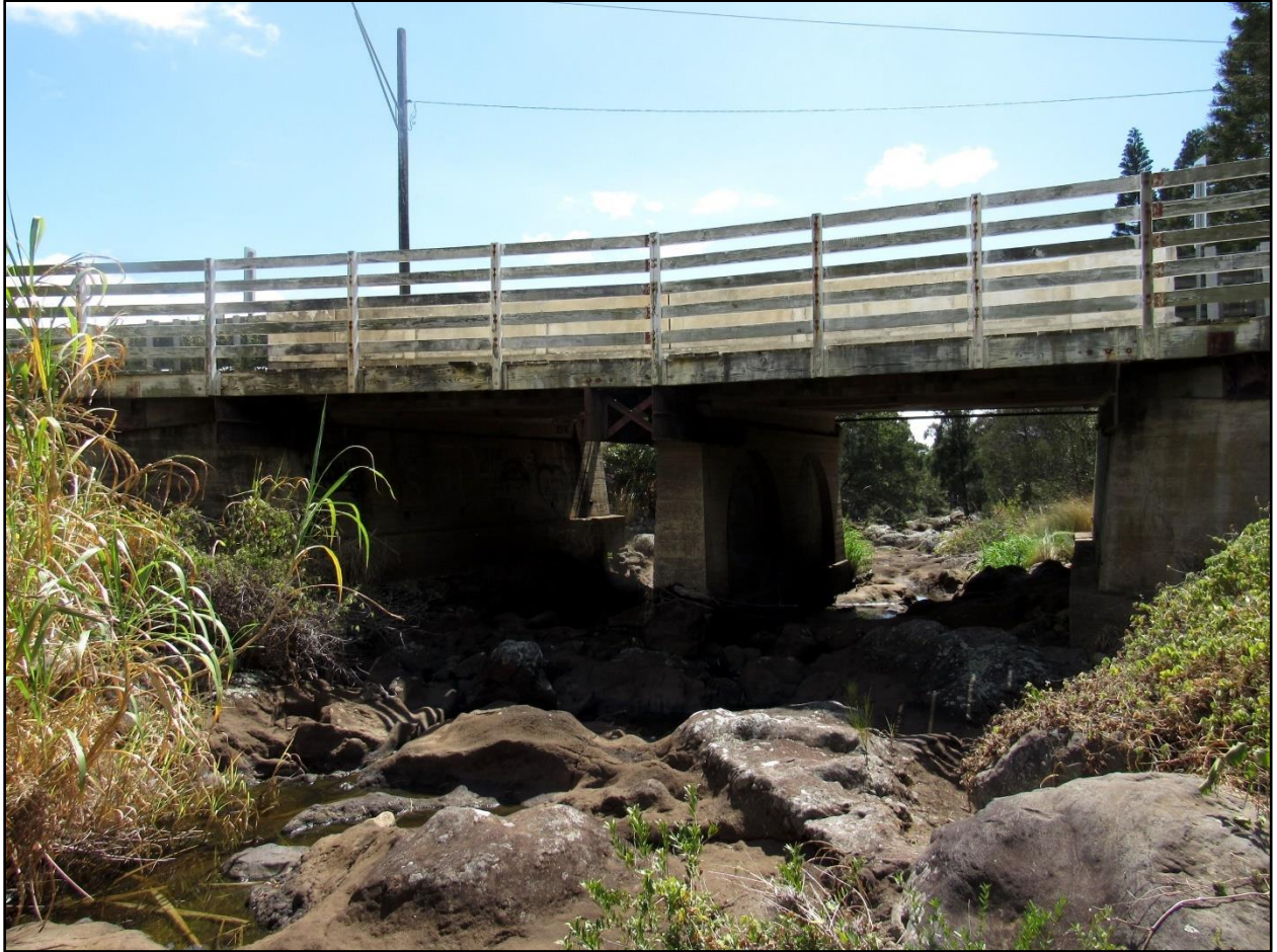
Figure 27. Site 29221 the Waiaka Bridge, north elevation.
