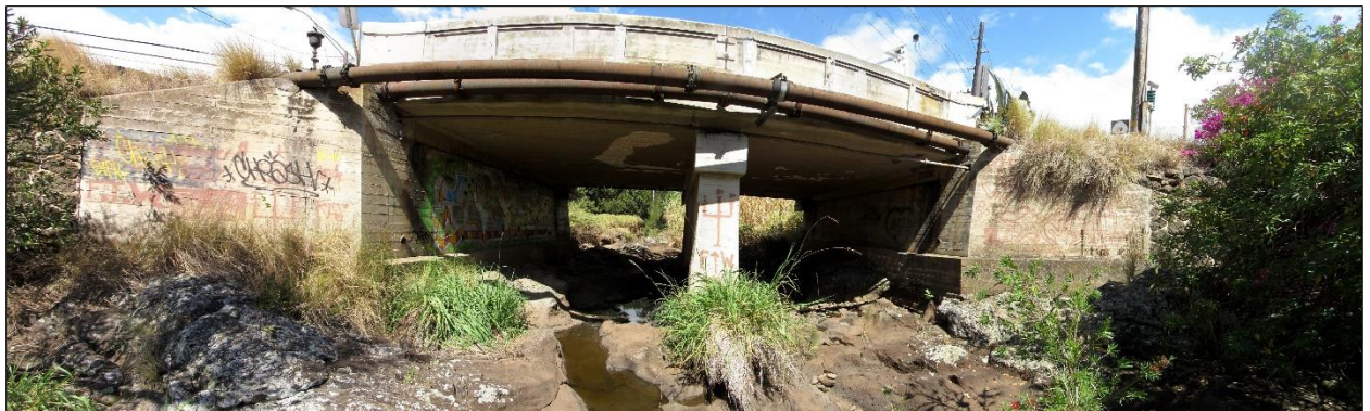
Figure 28. Site 29221 the Waiaka Bridge, south elevation.
