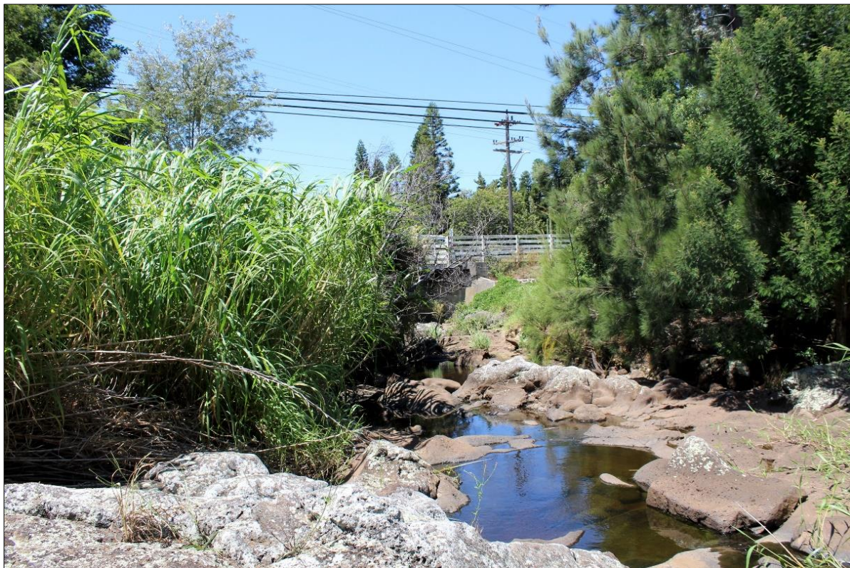
Figure 8. Keanu'i'omanō Stream looking downstream toward Waiaka Bridge, view to the southwest.
