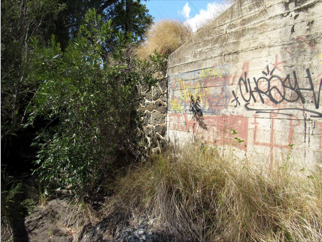
Figure 32. Site 29221 Waiaka Bridge detail of concrete and masonry abutment wing walls, view to the northwest.
