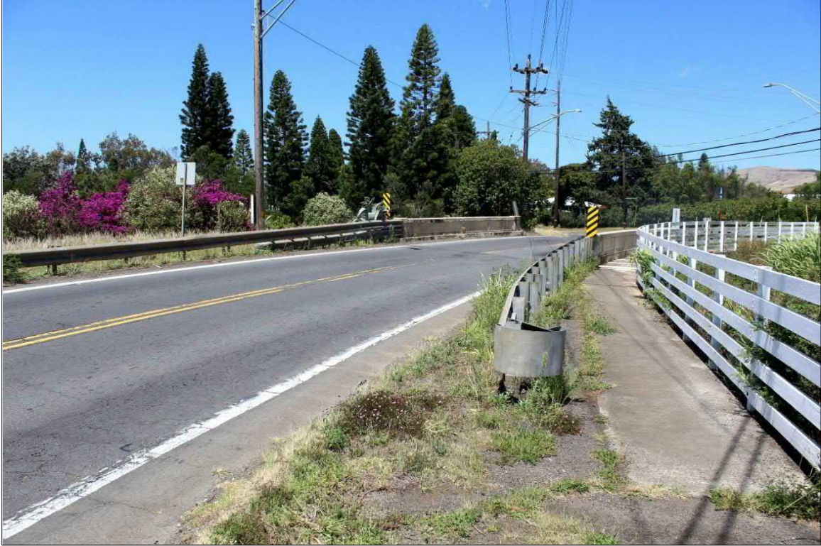
Figure 8. Waiaka Bridge, view to the northwest.
