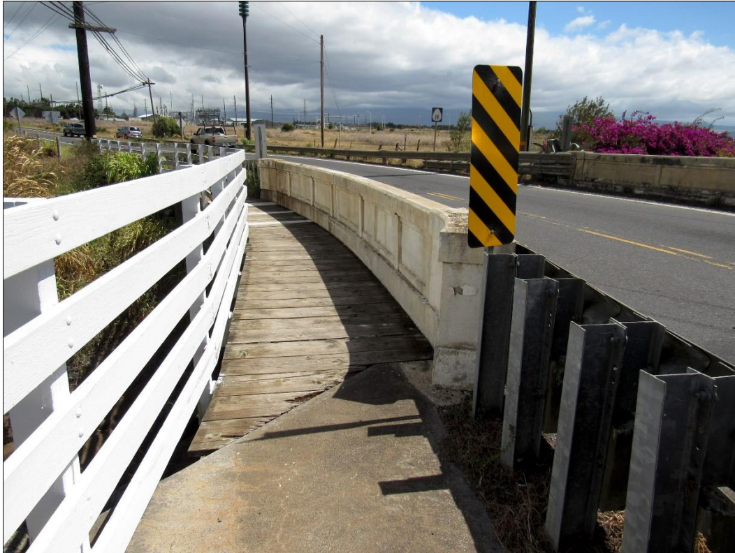
Figure 34. Site 29221 Waiaka Bridge wooden foot bridge, view to the east.
