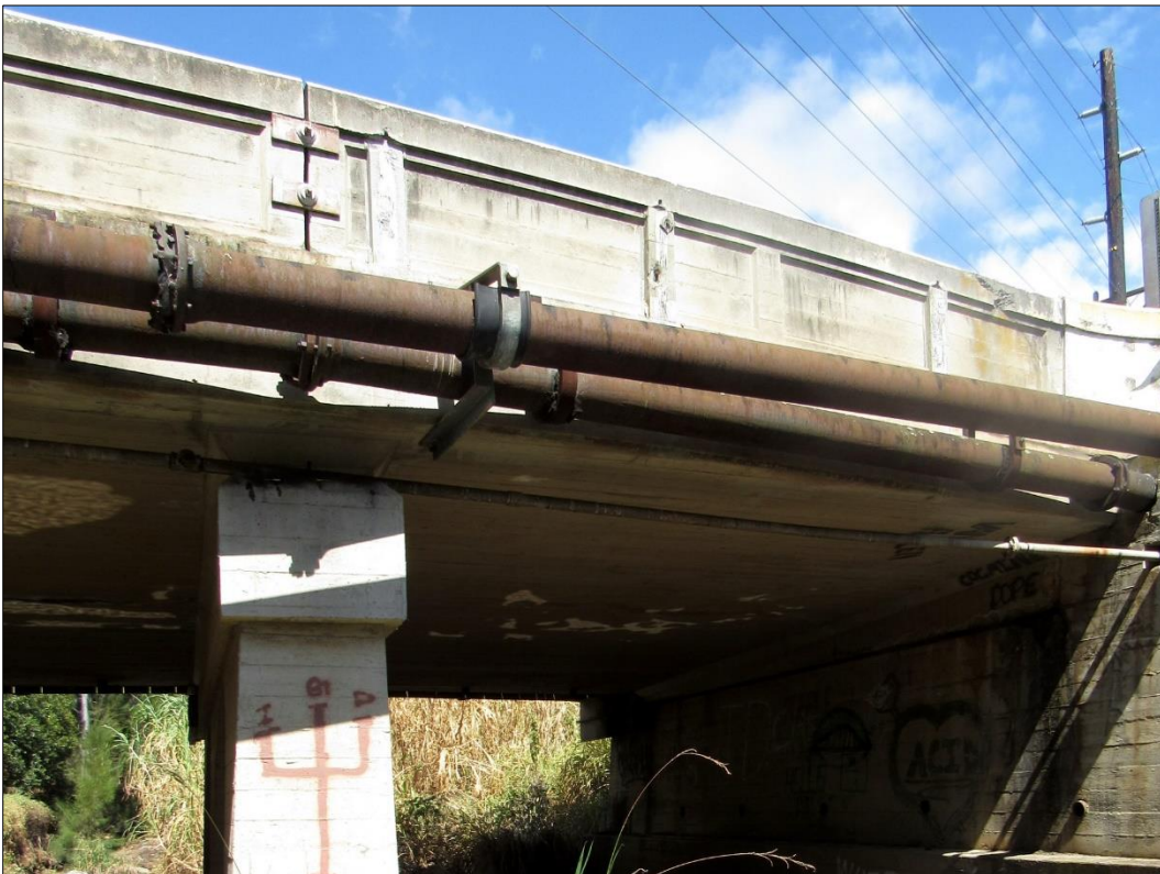
Figure 33. Site 29221 Waiaka Bridge detail of parapet, view to the northeast.
