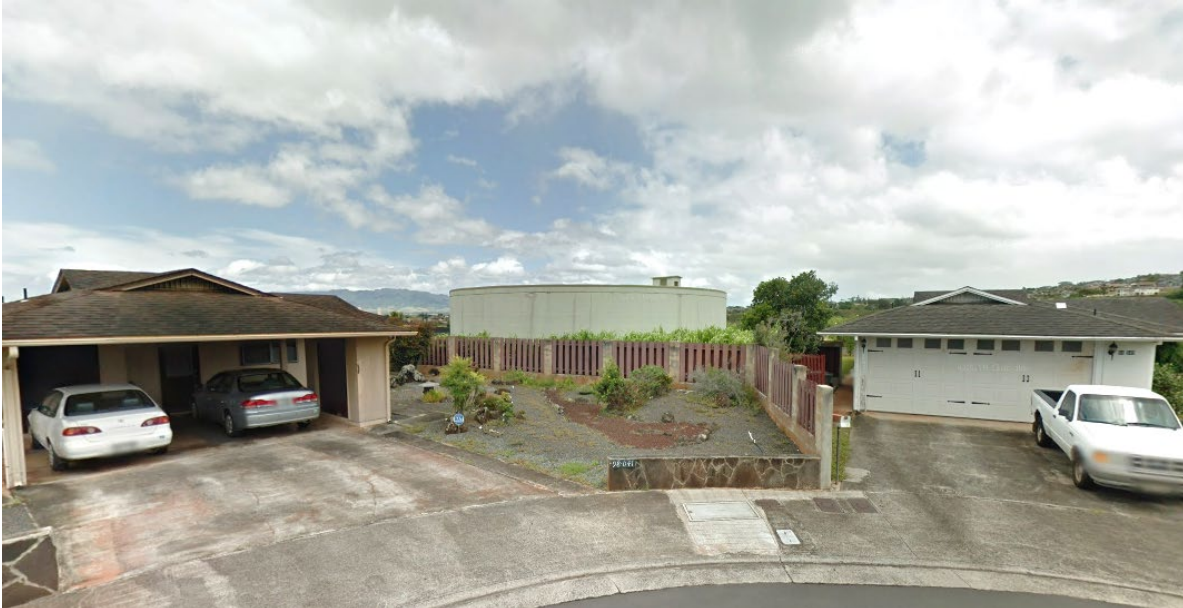
Photo #8. View along Puaalii Way from Google Street View (July 2011). The Waimalu 217' Reservoir is visible as an urban form that is behind and between two single-family homes along the Puaalii Way cul-de-sac.
