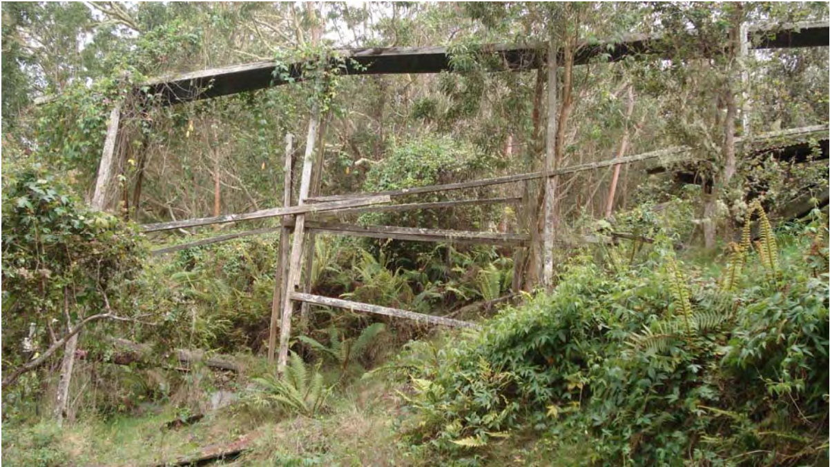
Figure 16. Flumes used to transport water to wooden tanks.
