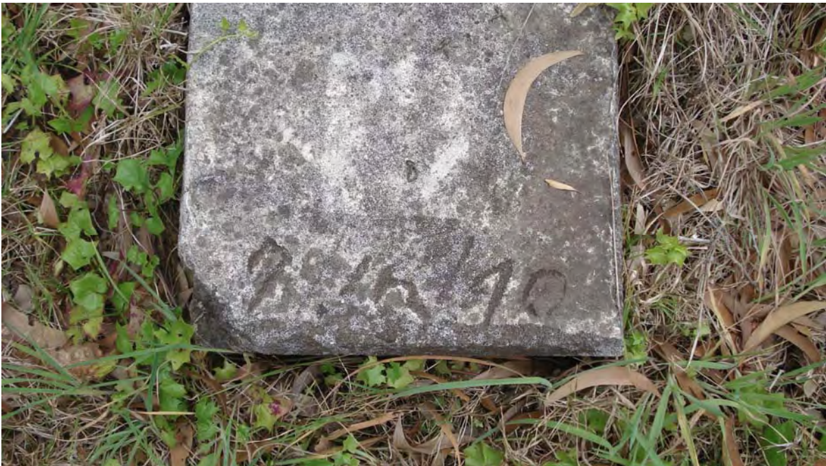
Figure 19. The year 1940 etched in a remaining concrete tank foundation.
