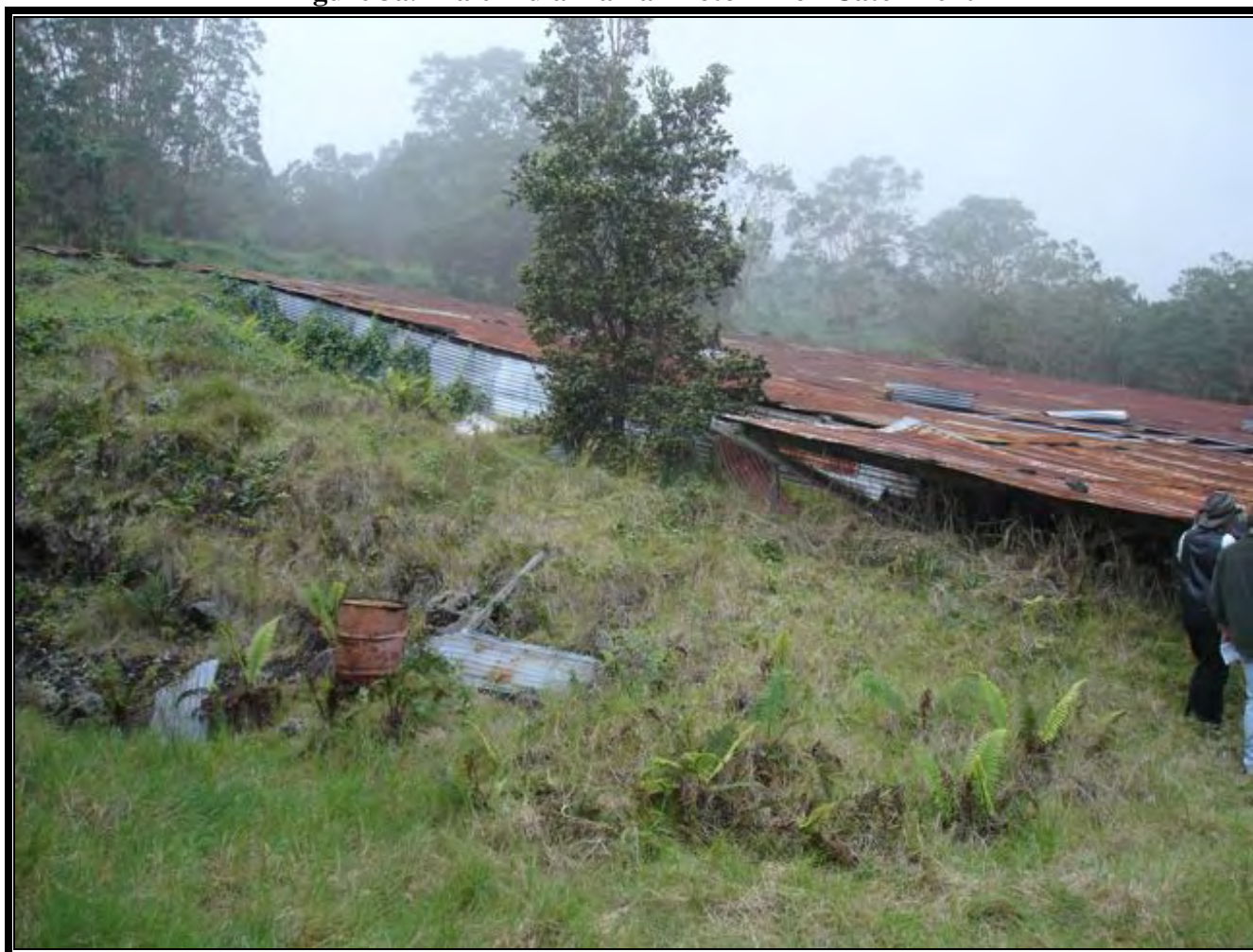
Figure 3a. Hale Piula Haina Photo – Iron Catchment
