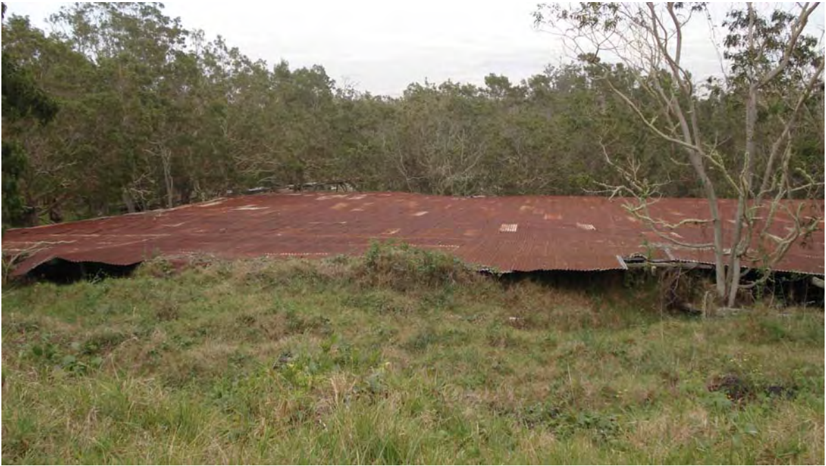
Figure 14. Corrugated roofing structure located at Hale Piula , view to the north.
