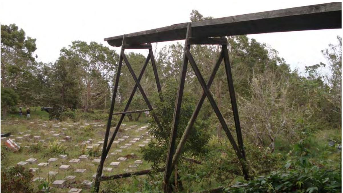
Figure 17. The end of the water flume where water would drop into large tanks.
