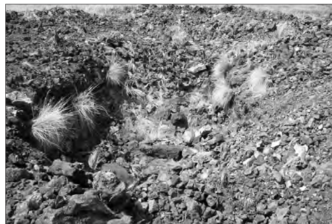
Figure 9. Opening # 6 filled with bulldozed rubble (View West)
