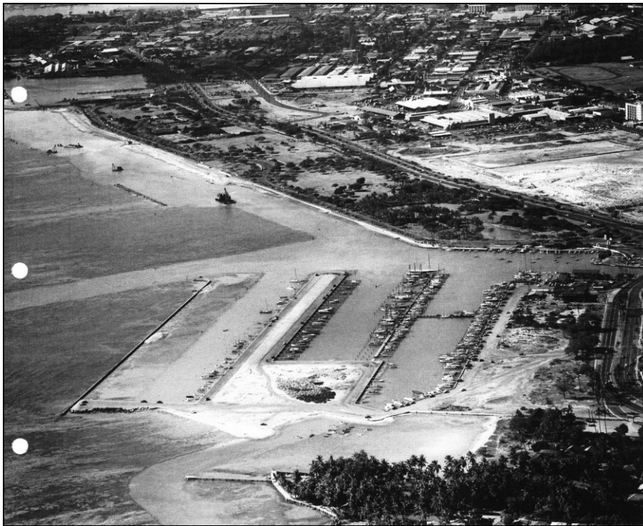
Figure 27. 1950s photograph of dredge boats between Ala Wai Yacht Club (right foreground) and Kewalo Basin (left background); also note coral fill (white) area on land where the future Ala Moana Shopping Center will be built (Hawai'i State Archives)
