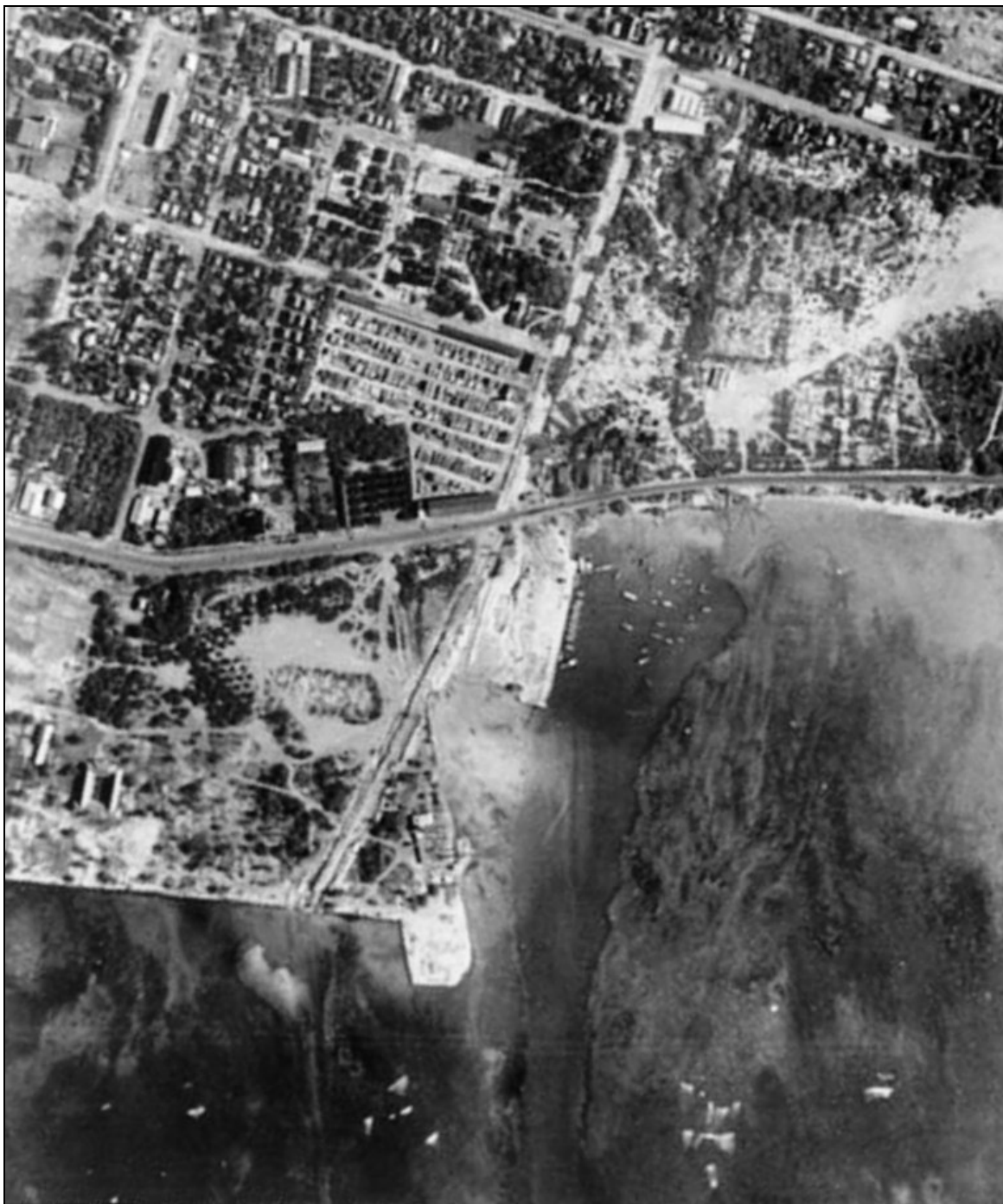
Figure 23. 1927 aerial photograph showing the natural deep pocket in the reef (just prior to dredging) and the brand new and in-progress land fill on the west side; A very narrow strip of sand is shown between the narrow beach road and the reef (Hawai'i State Archives)
