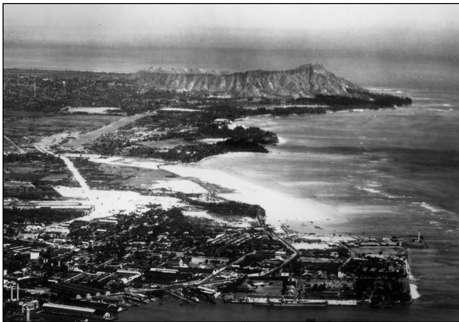
Figure 25. 1931 aerial photograph, showing dredged materials (white crushed coral) used in the construction of Kapi'olani Boulevard and used for fill in marshy areas of Honolulu and Waikīkī (Hawai'i State Archives)
