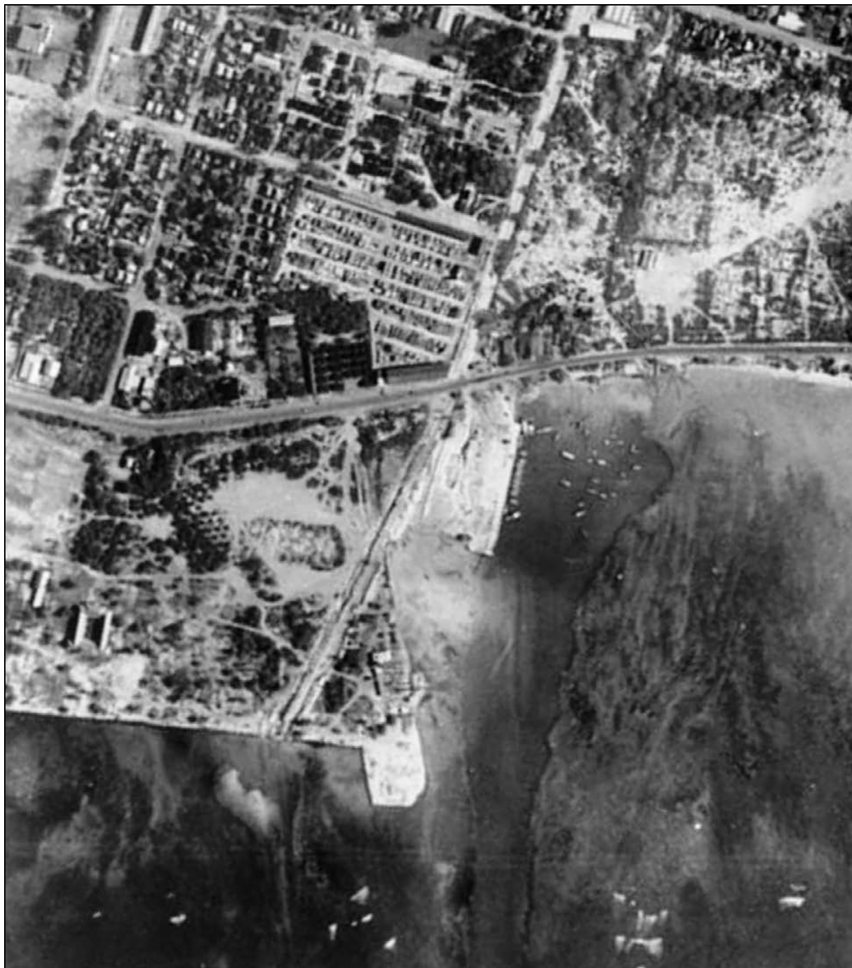
Figure 21. 1927 aerial photograph showing the natural deep pocket in the reef (just prior to dredging) and the brand new and in-progress land fill on the west side (note: a very narrow strip of sand is shown between the narrow beach road and the sea most, or all, of which is believed to have been covered by seaward widening of Ala Moana Blvd.)
