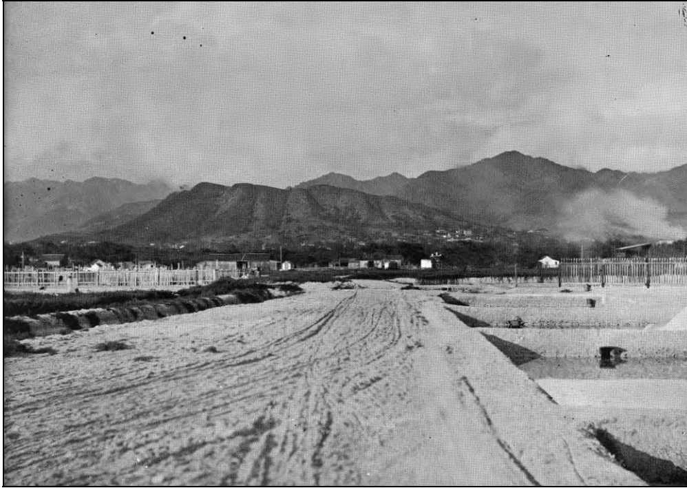
Figure 15. 1902 photograph of Kewalo Brine Basins; the Kaka'ako salt works may have extended back to pre-Contact times and are shown here going strong in 1902 (Scott 1968:579)
