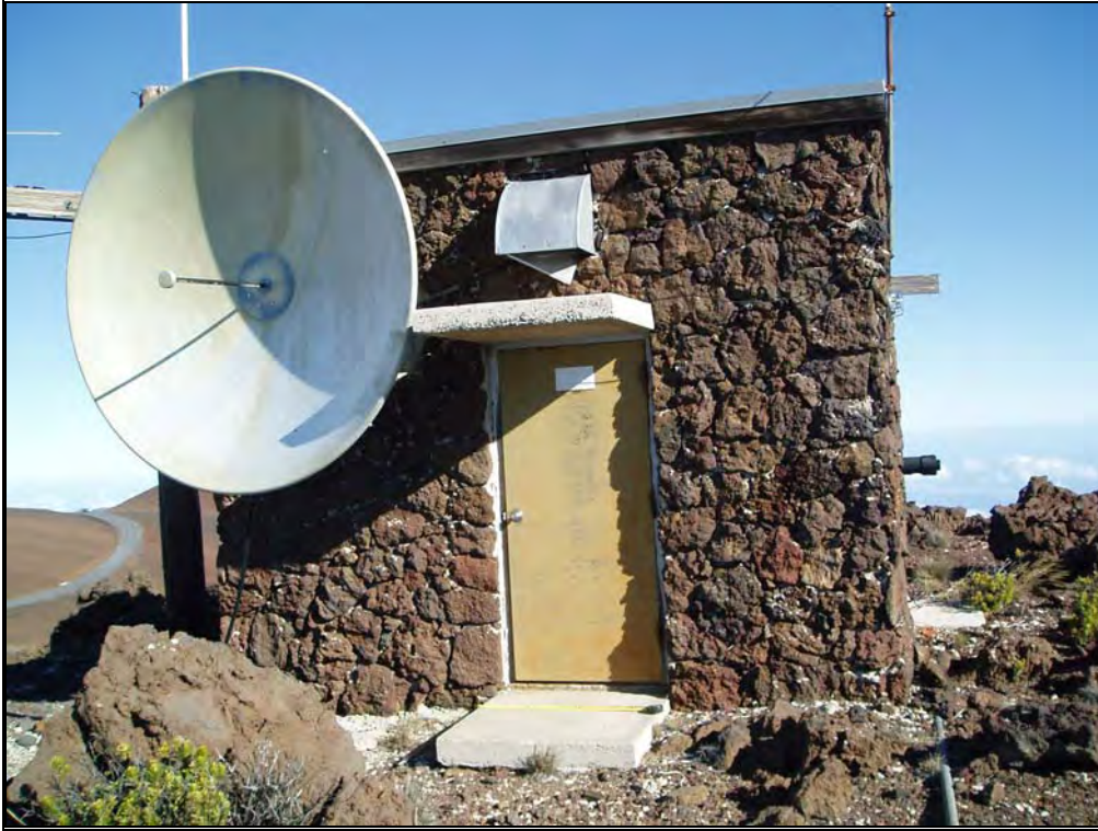
Photograph 6: General view to the north of Reber Circle of an older mid-1960s antenna building (see Figure 3 for location of this structure).
