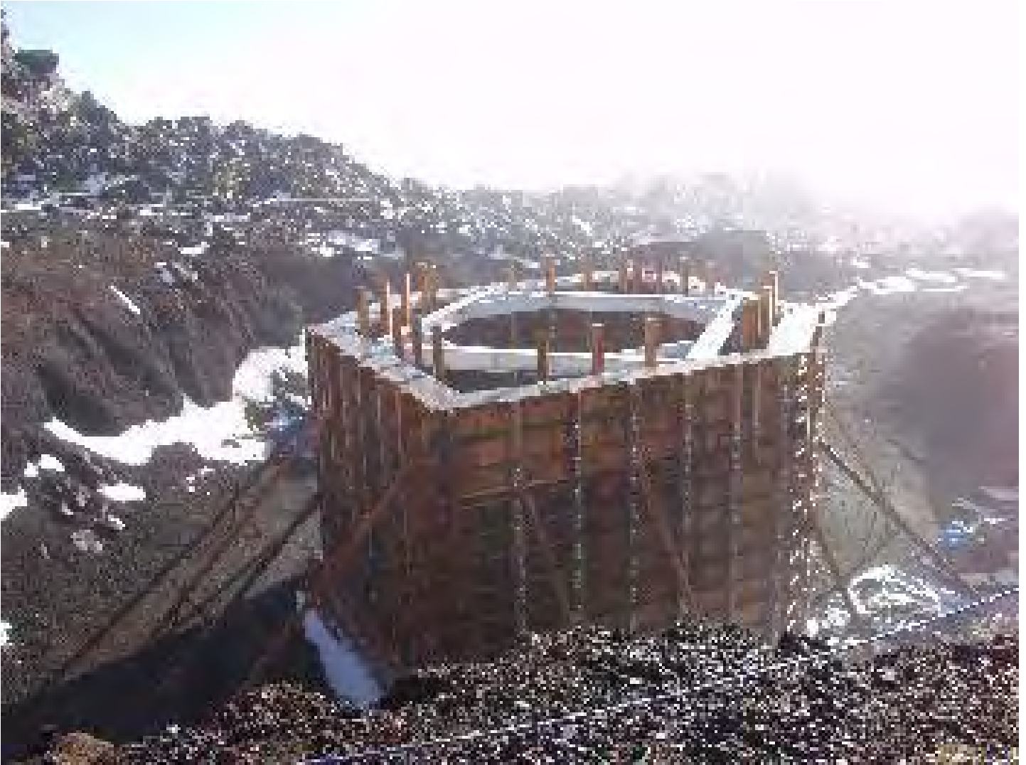
Shows structure with snow.
