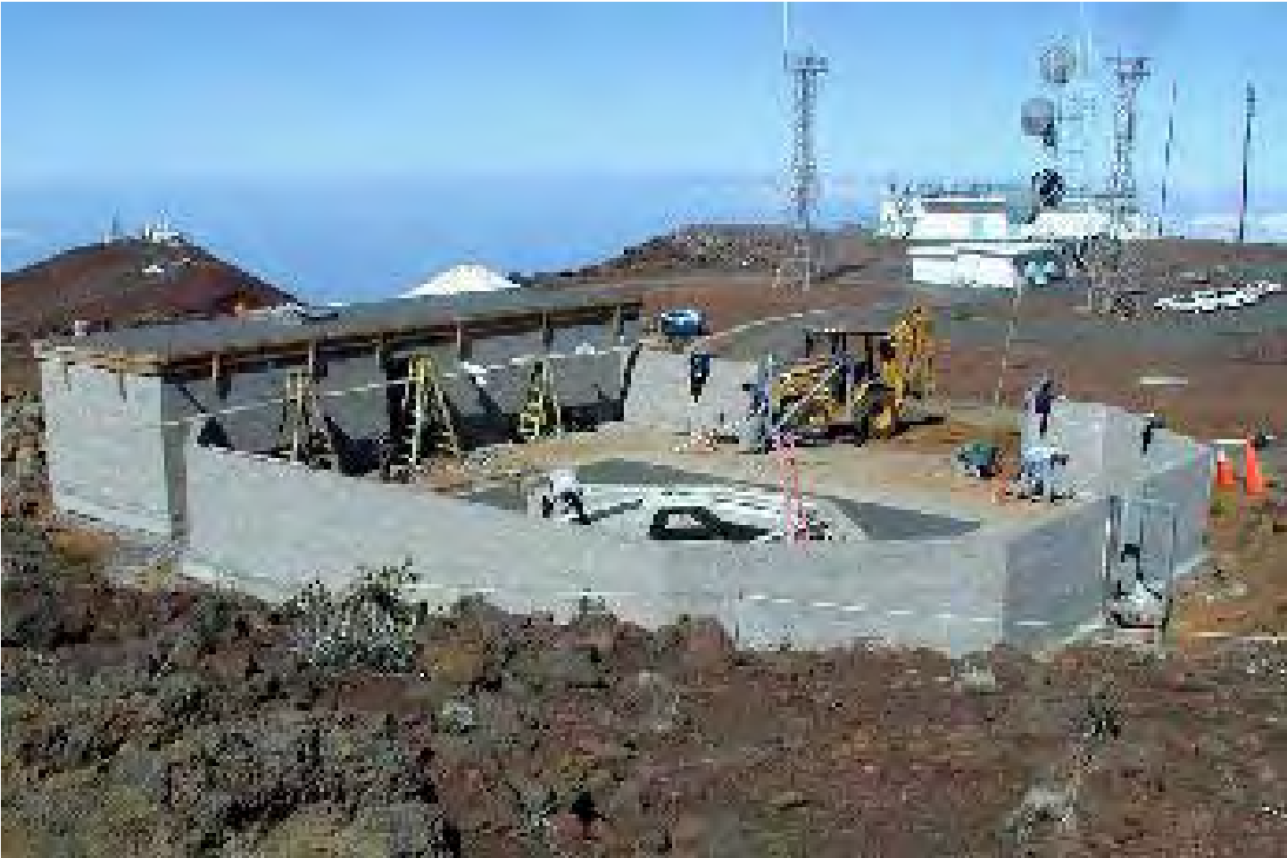
Concrete enclosure of Faulkes Telescope.
