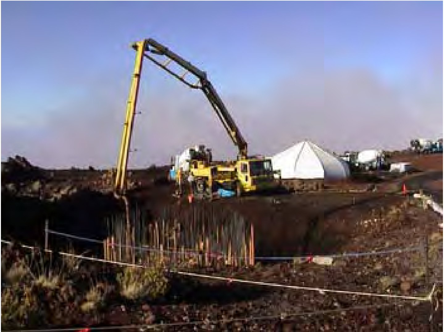
Shows boom truck pouring concrete into form of platform.
