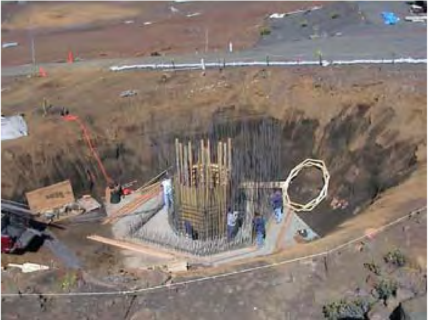
Shows the entire pit dug for the foundation.
