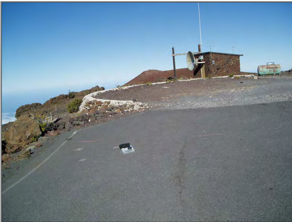
Photograph 3: General view to the north across Reber Circle—Site 5443.
