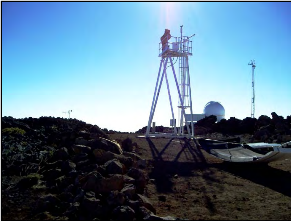
Photograph 4: View to the southwest of the data tower and weather tower (right), note push pile at left and construction materials at right; Mees Observatory is in the background.
