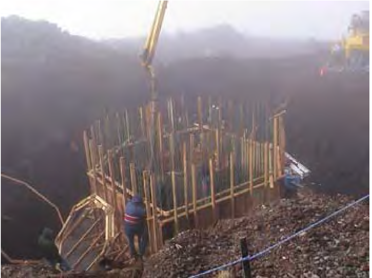
Construction of the foundation.
