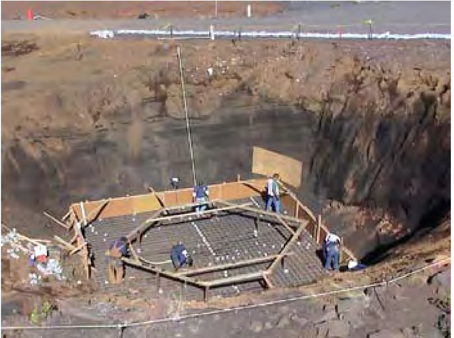
Workers constructing base of telescope in “pit”.
