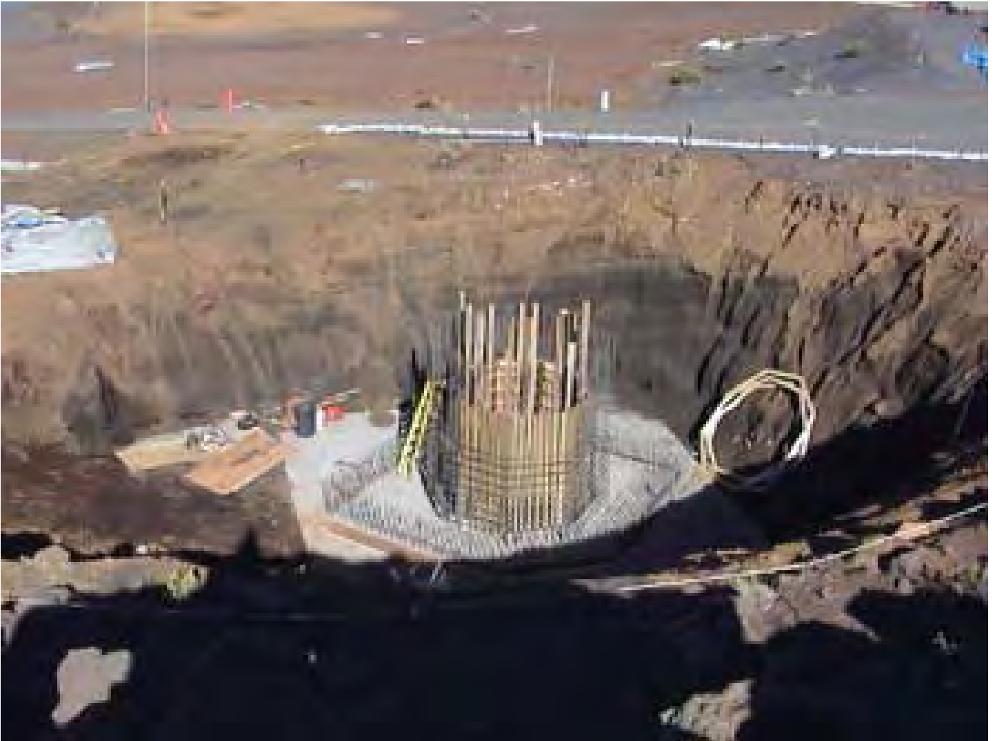
Concrete foundation, Faulkes Telescope
