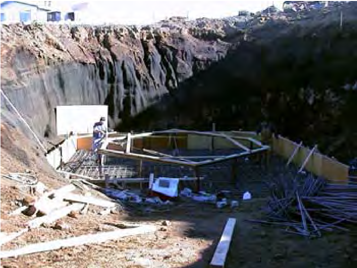
Shows excavation for Faulkes telescope foundation.
