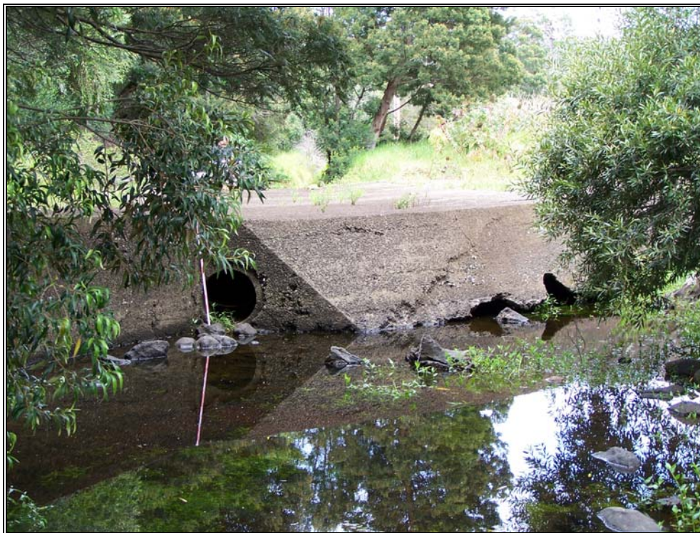
Figure 33. Western side of SIHP# 26873 showing culvert, view to east
