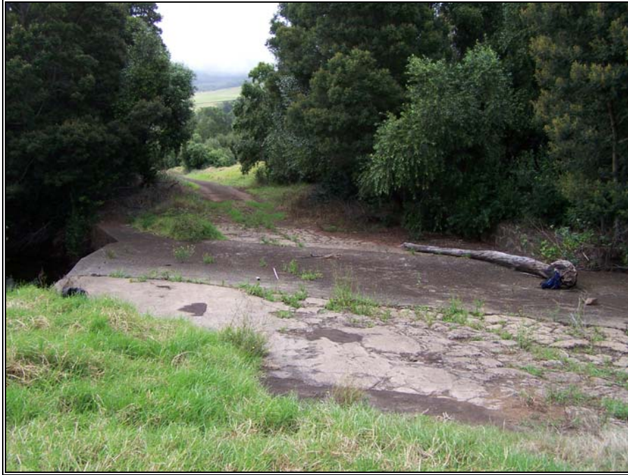
Figure 30. SIHP# 26873 ford and associated roadway, view to northwest
