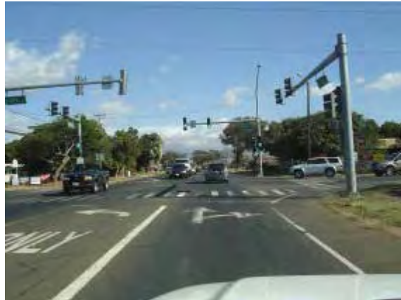
Figure 3.9-7. Representative Two-lane Highway—Hāna Highway at Dairy Road
