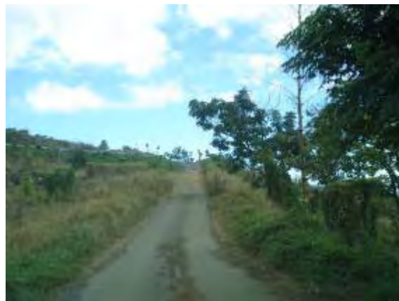
Figure 3.9-10. Representative Unpaved Pastoral Road: Pāpaka Road, Eastern Portion
