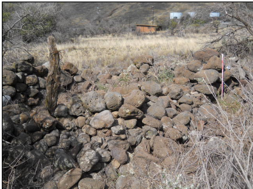
Figure 16. Photo showing SIHP # 50-10-22-29224 exterior eastern wall; view to the northwest
