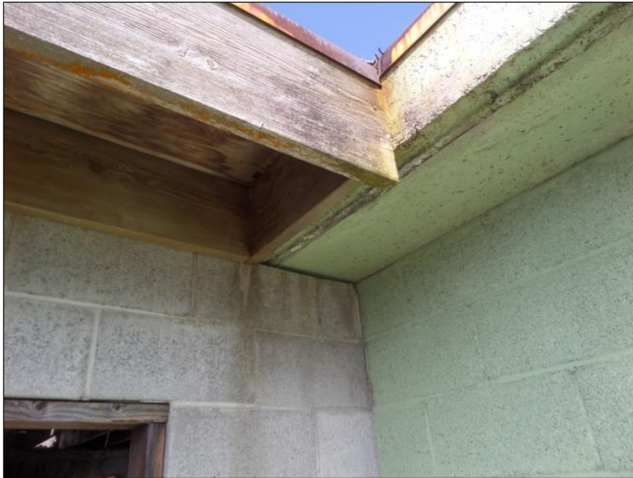
Figure 81. Close-up of addition walls and eaves.
