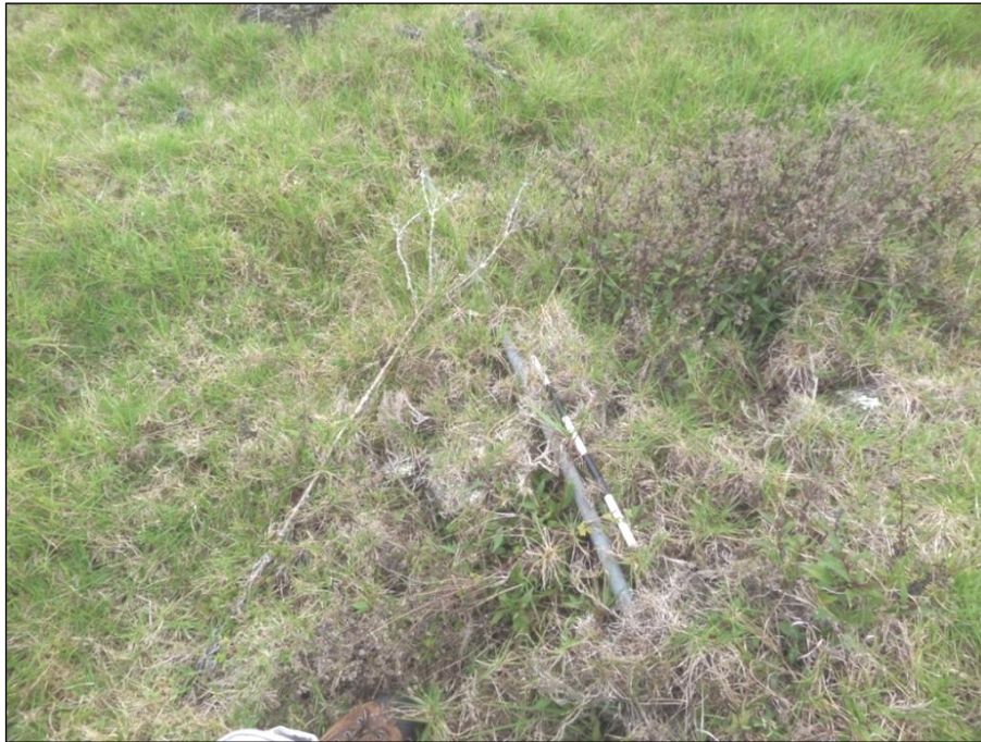
Figure 21. Three quarter inch galvanized irrigation pipe running through Waiho 1 Waimea Paddock.
