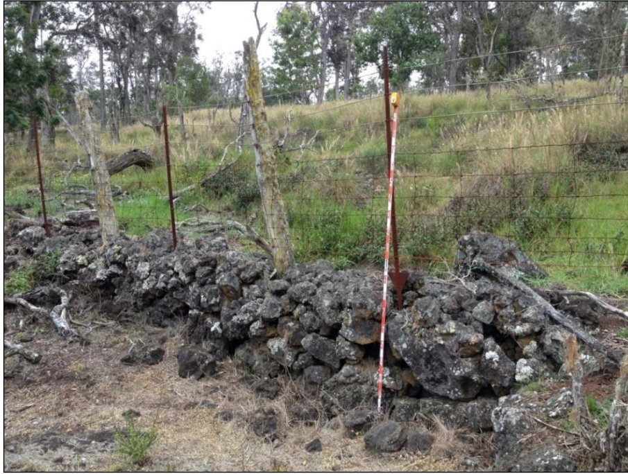
Figure 31. Substantial cobble chinking at base of Fence 4. View to northeast.
