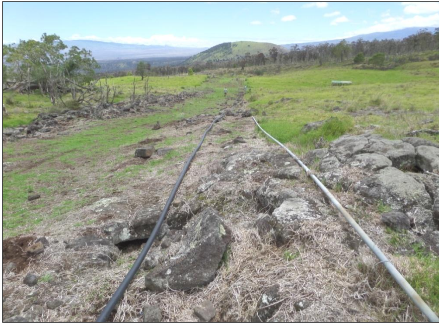
Figure 19. Irrigation lines running toward Henahena Unit along mauka side of fire break.
