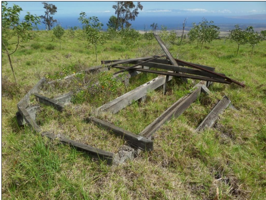
Figure 124. Site 30397, wooden beam support structure, facing northwest.
