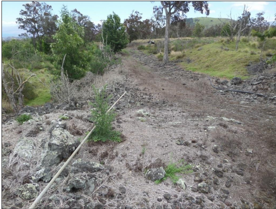
Figure 26. Remnant pipe along Henahena Unit corridor, Section 1. Modern polyethylene pipe visible at far right.
