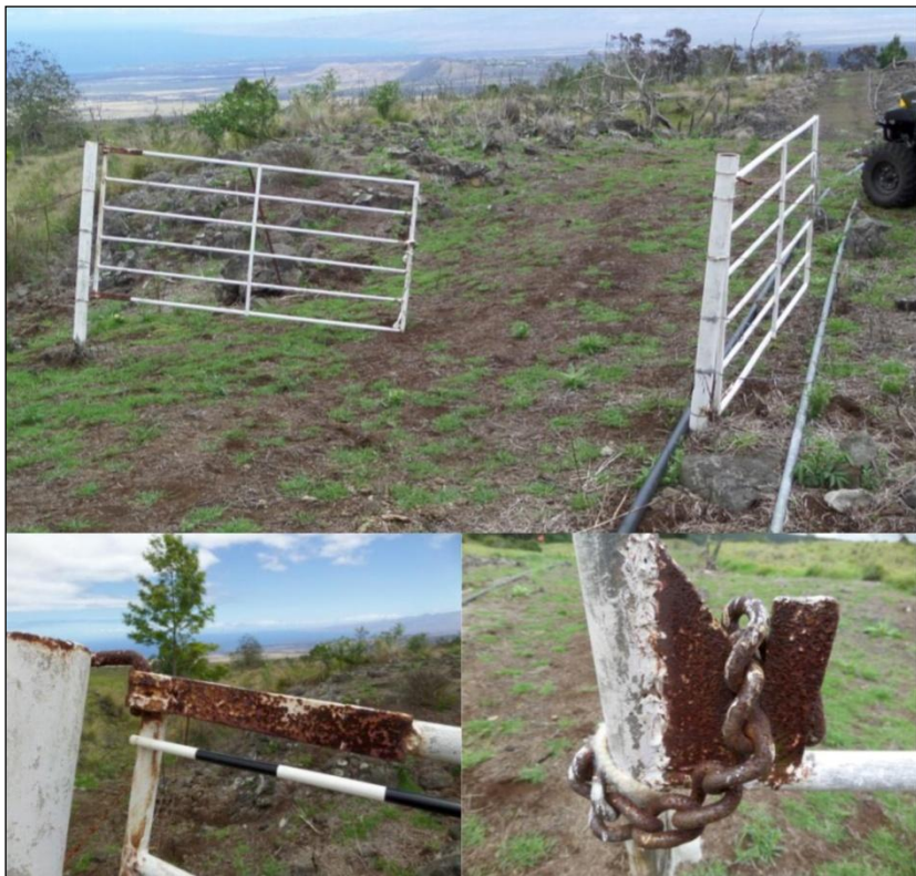
Figure 25. Steel gate in Waiho 1 Waimea Paddock. Detail: custom fabricated gate hardware.
