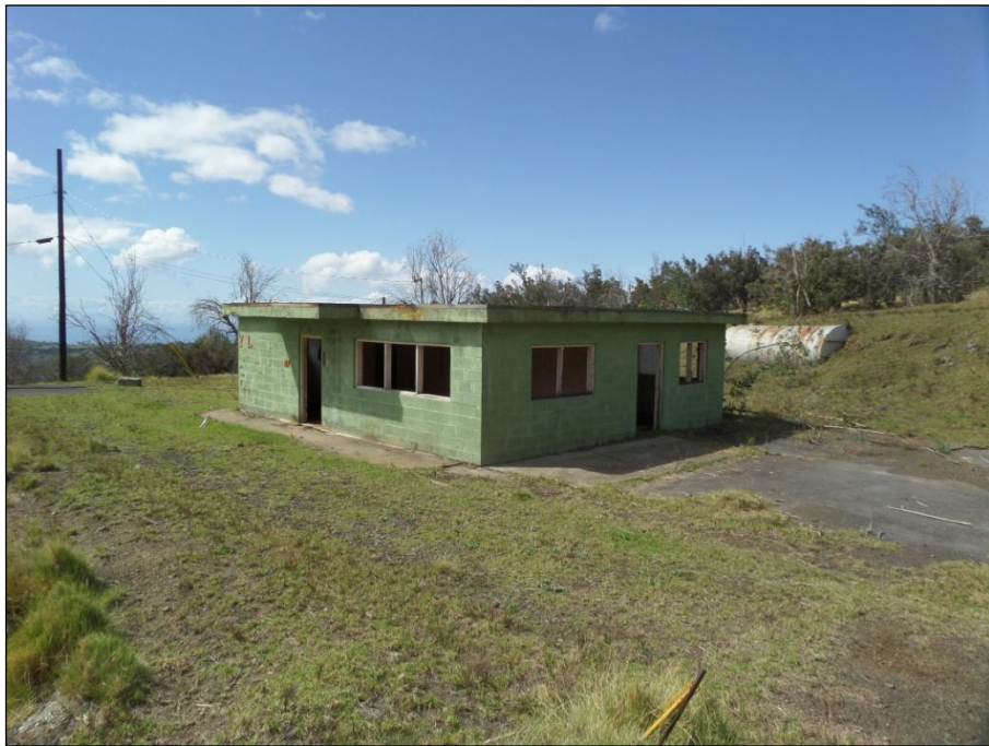
Figure 77. Quarry office, facing northeast.
