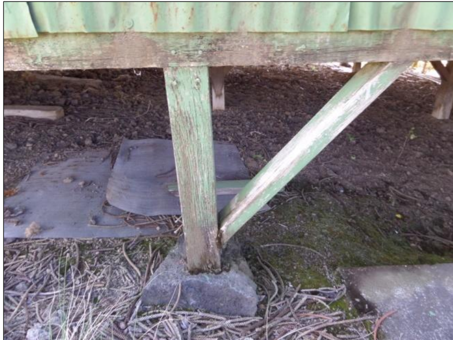
Figure 75. Close-up of wooden support post and rock pier, facing southwest.
