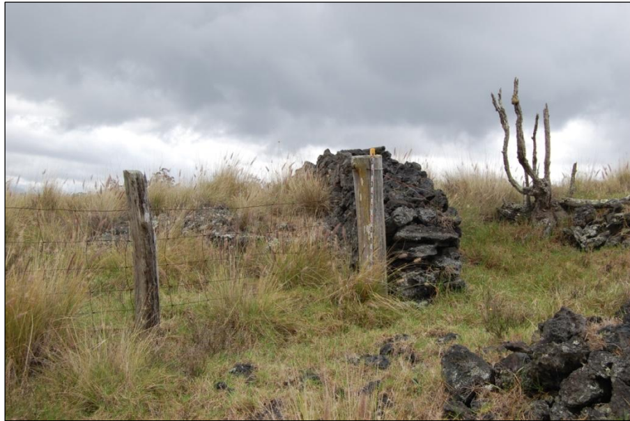
Figure 106. End of wire fence at rock wall (Site 30310), facing southeast.
