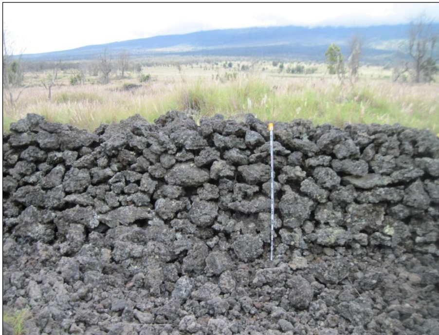
Figure 117. Site 30310 rock wall, facing southwest.
