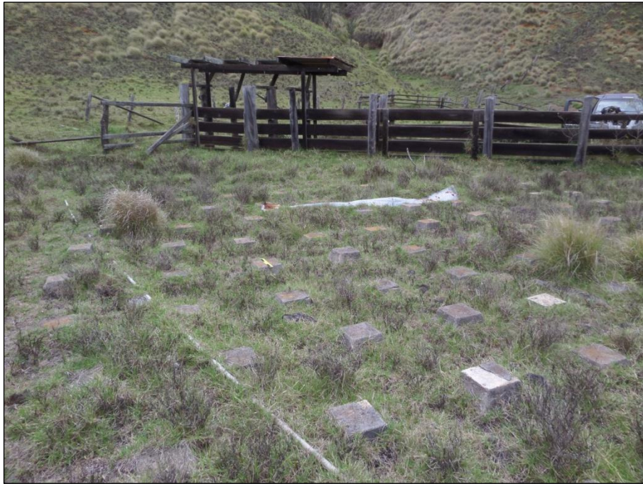
Figure 104. Galvanized waterline running from the foundations to the northeast.
