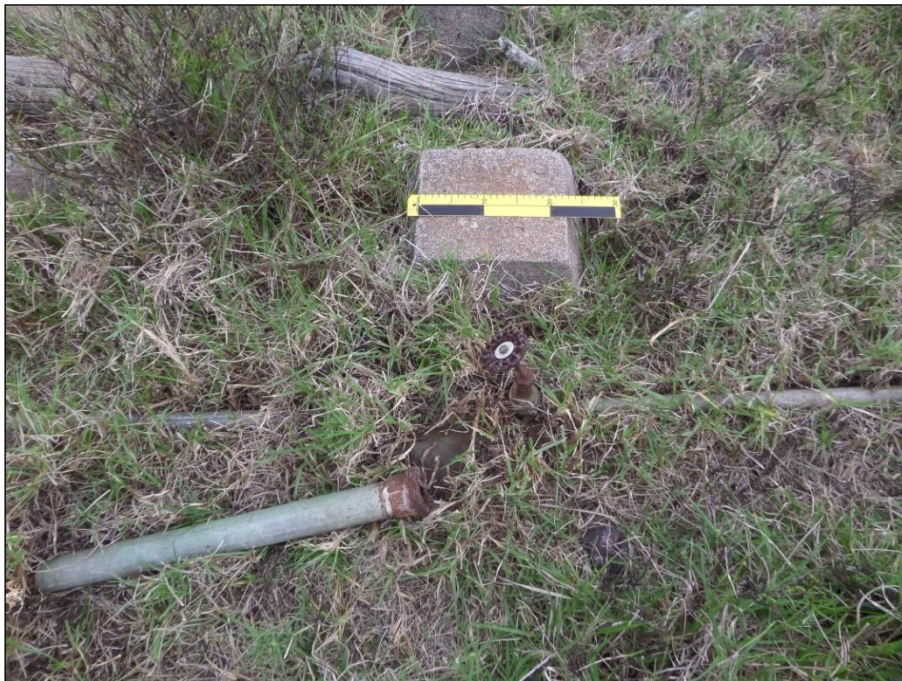
Figure 103. Close-up of one of the concrete footings, waterline, and a valve.
