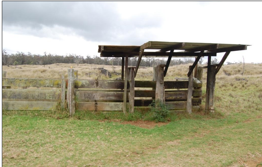
Figure 99. sheltered section of the chute, facing southeast.
