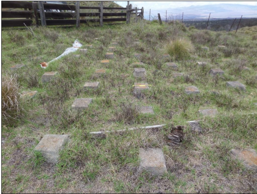
Figure 102. Concrete footings laid out in rows, facing north.
