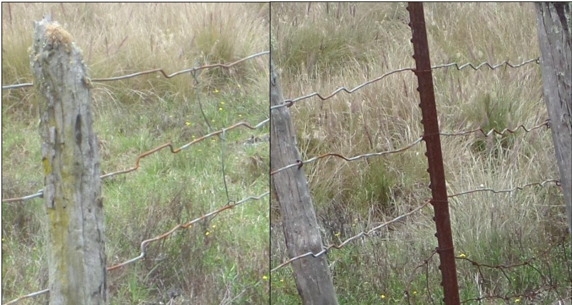
Figure 28. Example of line crimping to correct sagging in heavy gauge wire.
