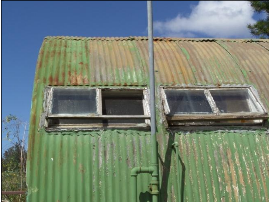
Figure 73. Close-up of corrugated metal roof and wood-framed windows, facing northeast.
