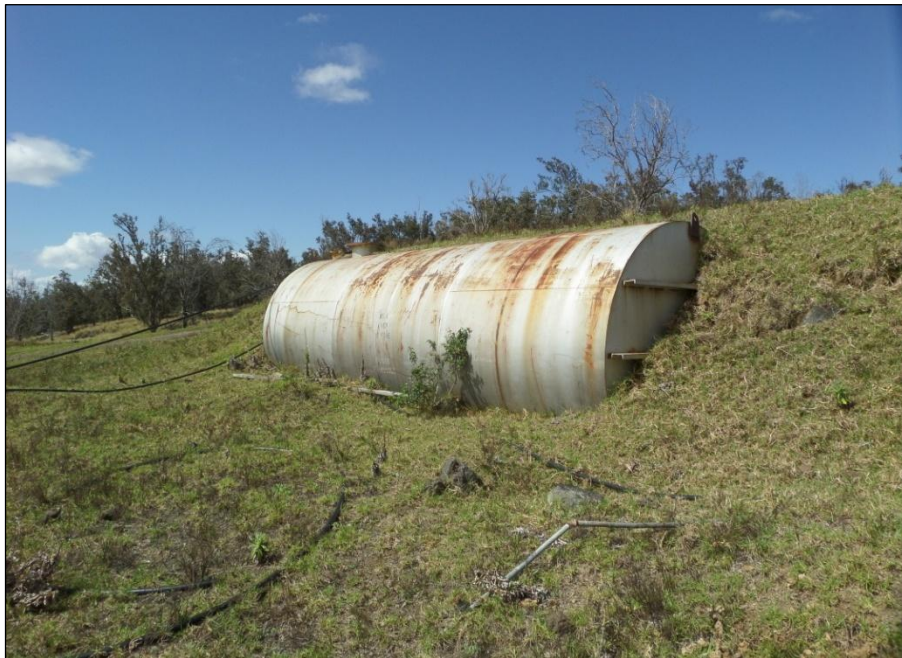
Figure 83. Partially buried tank northeast of quarry office, facing northeast.
