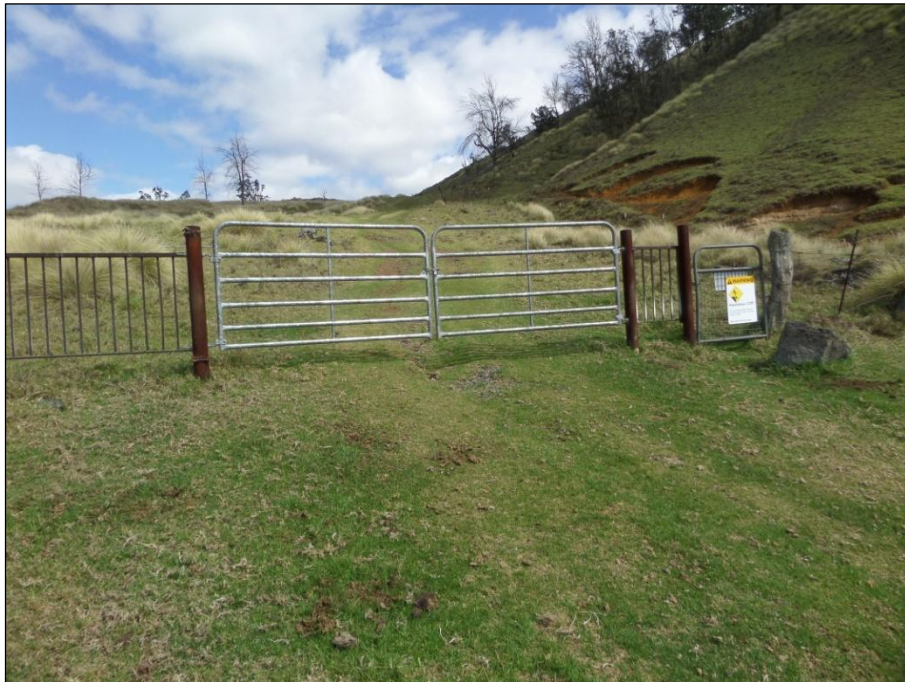
Figure 55. Metal gate in Fence 8 along the quarry boundary, facing southeast.
