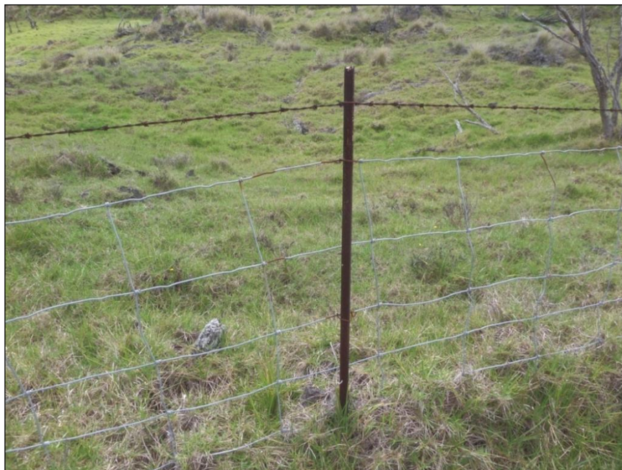
Figure 9. Aiea Unit Fence 1, t-post hung with woven wire and a single top-strand of four-point barbed wire.
