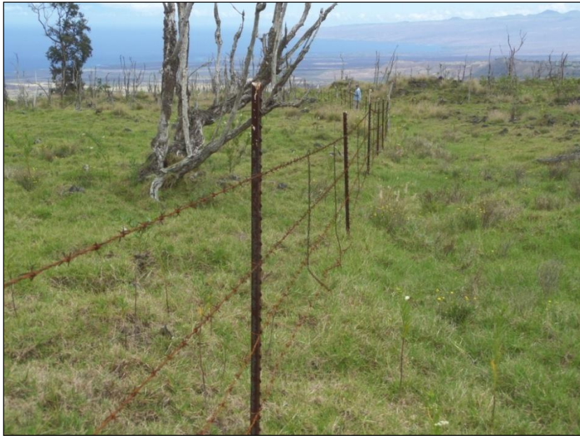
Figure 11. Aiea Unit Fence 2; t-posts hung with four strands of barbed wire. Interior paddock subdivision fence within Waiho 1 Waimea Paddock.
