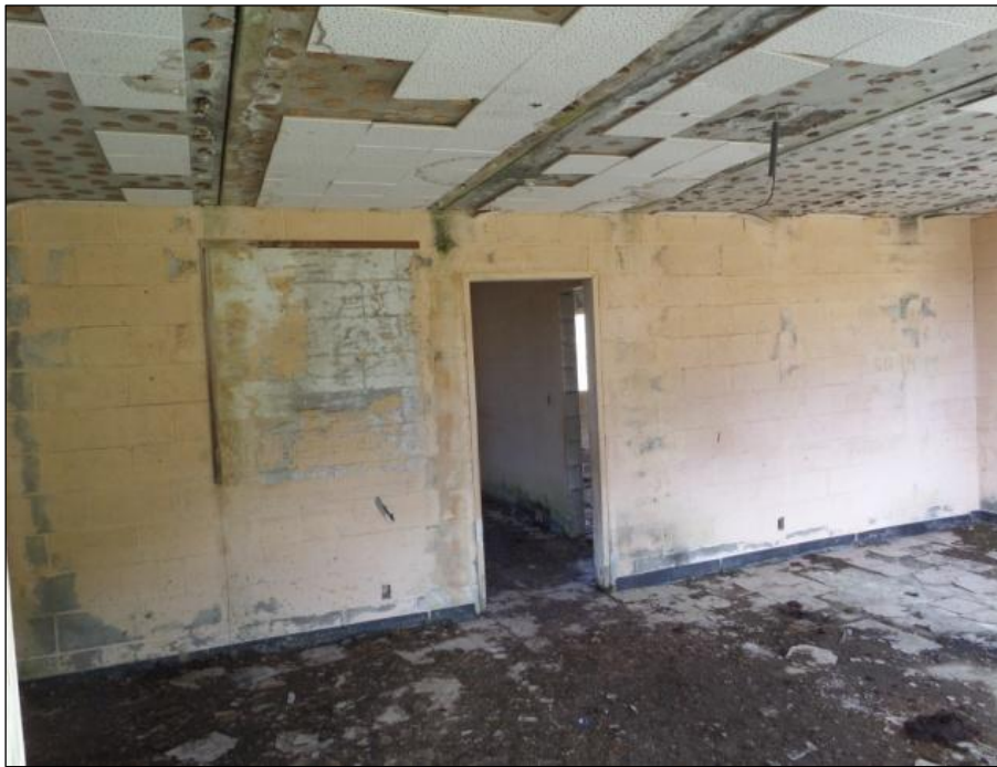
Figure 82. Main room of quarry office.
