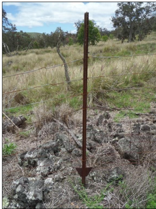
Figure 30. Complete view of older t-post type, including base plate.
