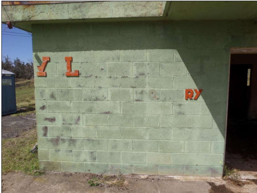
Figure 79. Wooden letters attached to wall of office near entrance, facing northeast.
