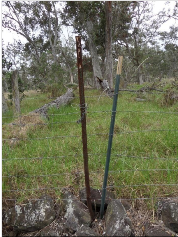
Figure 40. Two types of t-post on Fence 5. Older style on left, newer style on right.
