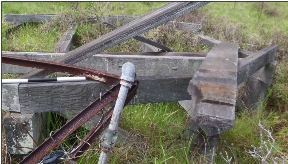
Figure 126. Close-up of galvanized pipe associated with support structure.
