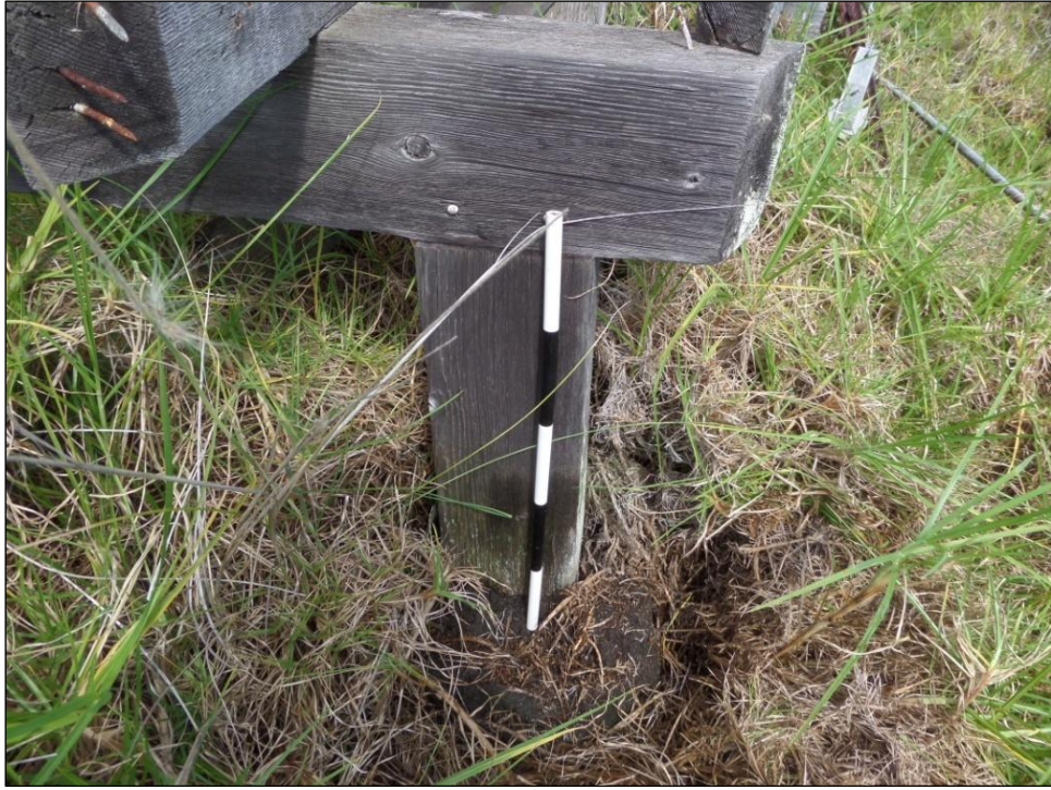
Figure 125. Close-up view of support pier with showing beam resting on rock.
