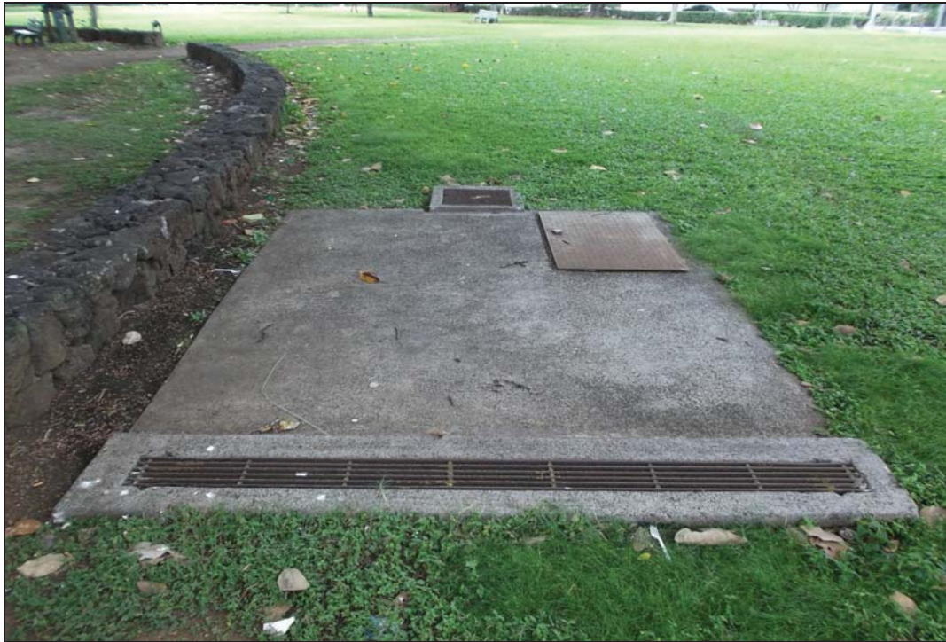
Figure 23: Photograph of the Fountain Pump. View to Southwest.
