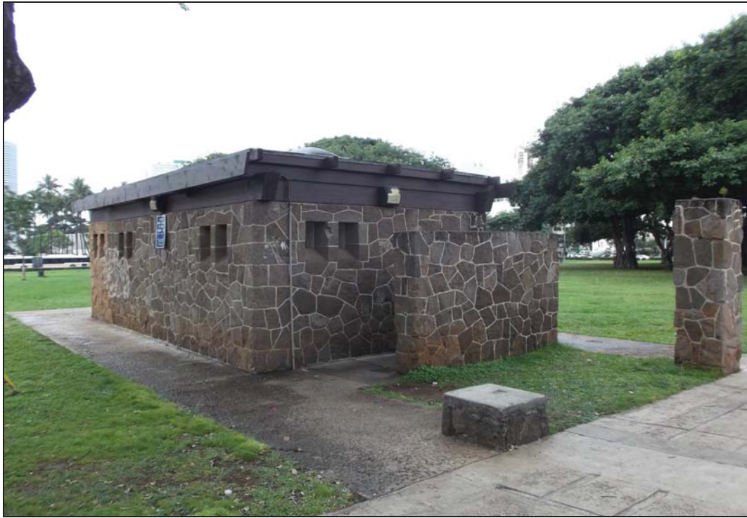
Figure 12: Photograph of Basalt Block, Wood, and Cement Bathroom. View to Southwest.
