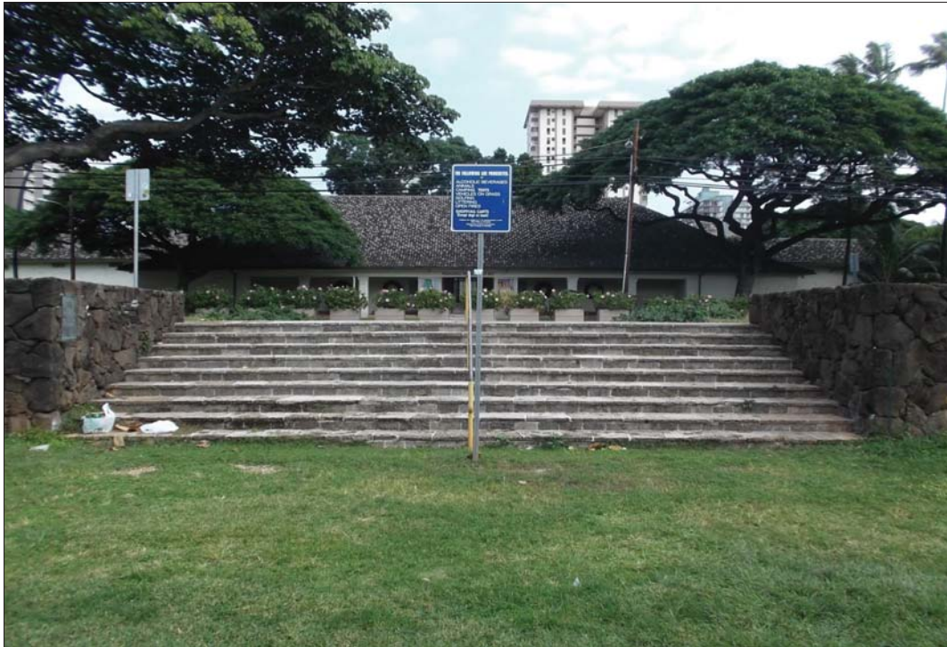
Figure 20: Photograph of the Cut-Limestone Block Staircase. View to Northeast.
