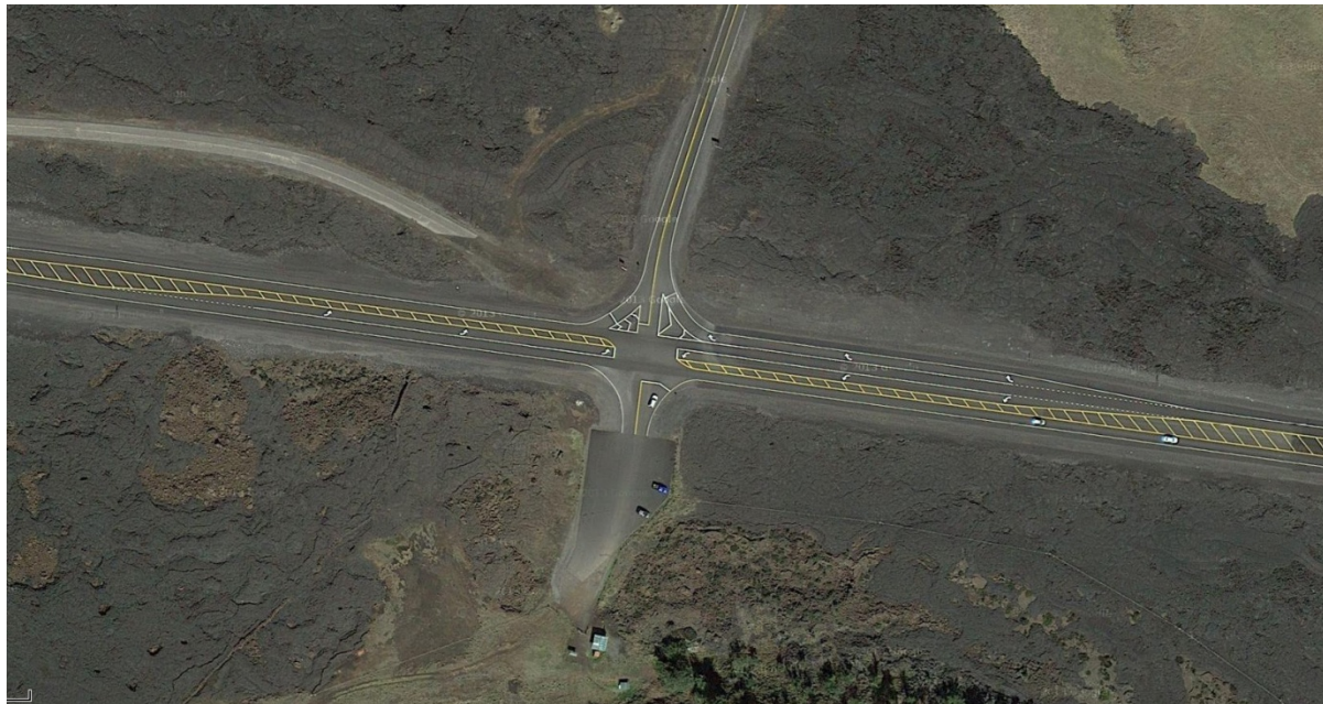
Figure 3-19: Intersection of Mauna Kea Access Road with Daniel K. Inouye Highway
