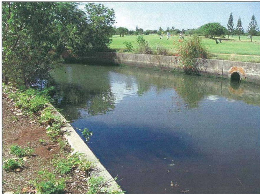
Figure 21. Photograph of concrete lined drainage canal, taken from northwestern portion of project area, view to south
