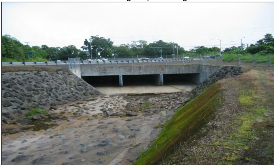
Figure 18. Waiakea Stream looking upstream at Waiakea-Uka channel from Station 18+00 Note scour damage repair on right bank.
