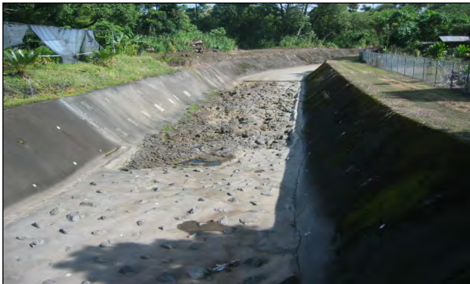
Figure 16. Waiakea Stream looking downstream at the upstream face of the T. Shiroma Bridge Note channel restriction
