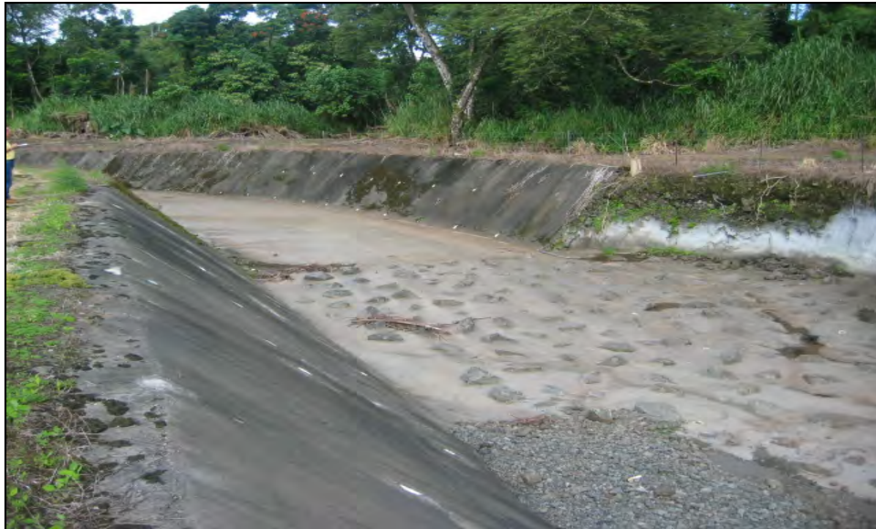
Figure 18. Waiakea Stream looking upstream at Waiakea-Uka channel from Station 18+00 Note scour damage repair on right bank.
