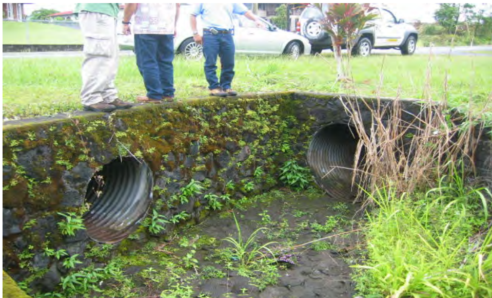
Figure 29. Palai stream looking at HaiHai St culvert
