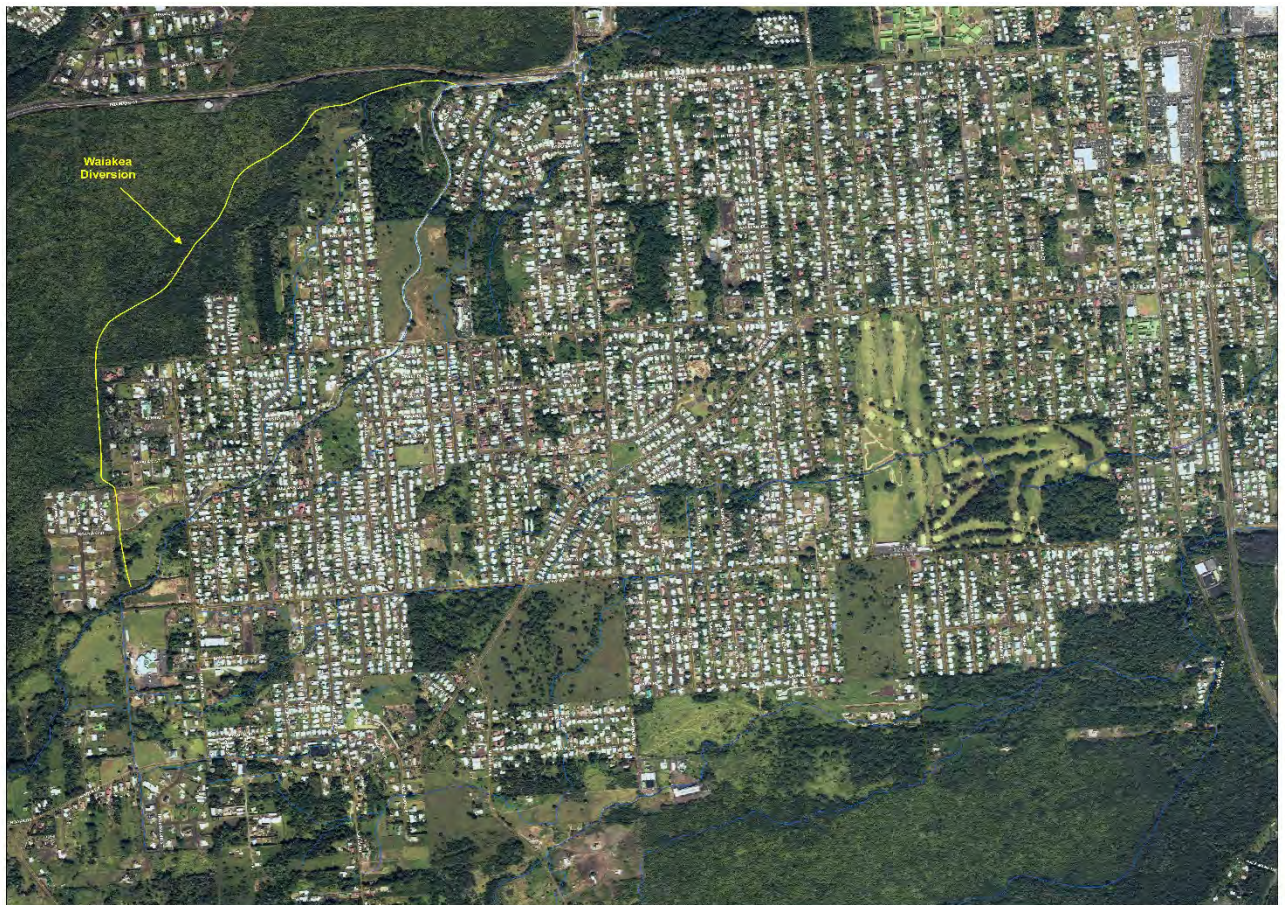
Figure 50. Location of Waiakea Stream Diversion Channel
