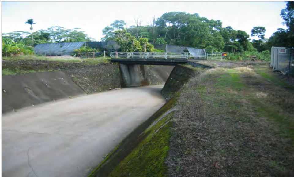
Figure 16. Waiakea Stream looking downstream at the upstream face of the T. Shiroma Bridge Note channel restriction
