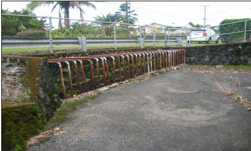
Figure 26. Palai Stream C looking at stormwater ditch inlet along HaiHai St.
