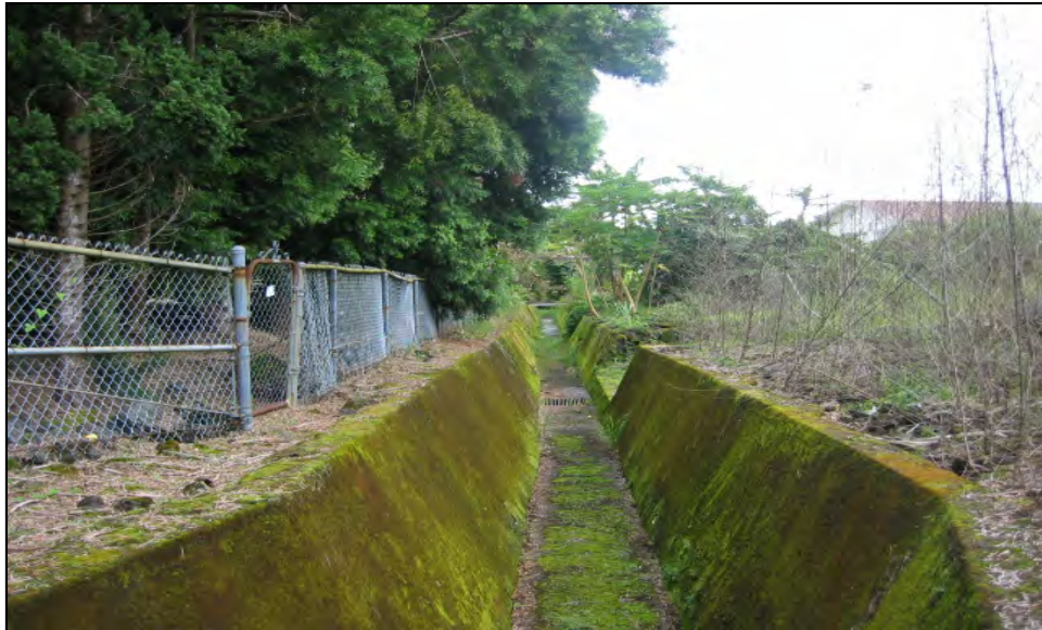
Figure 24. Palai Stream C looking upstream at drainage ditch from Station XX
