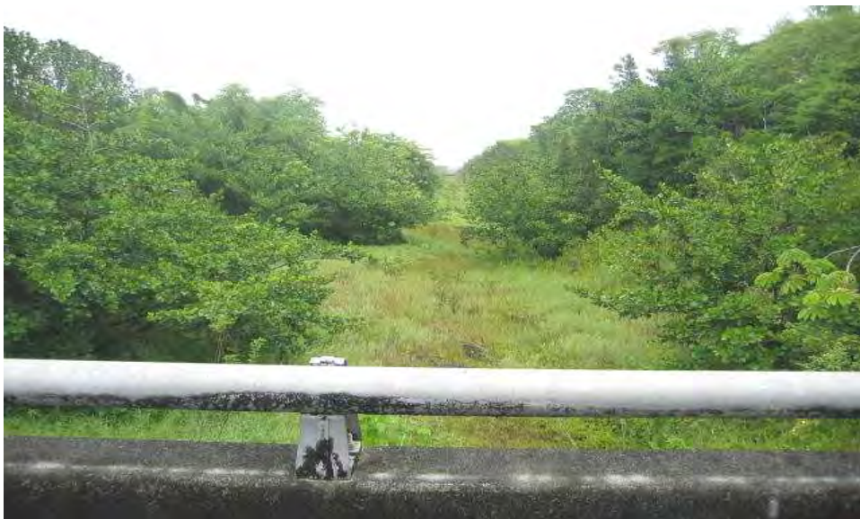
Figure 36. Four Mile Creek looking downstream from Awa St Bridge
