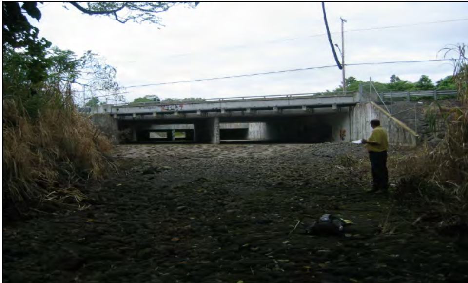
Figure 20. Waiakea Stream looking at downstream face of Komohana St Bridge
