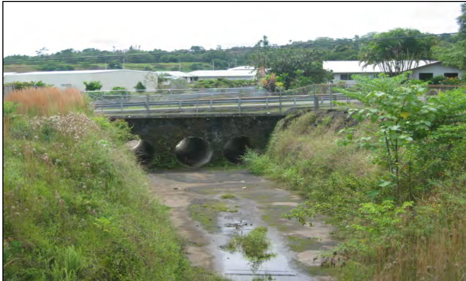
Figure 21. Kupulau Ditch looking upstream at downstream face of Ainaola Dr.
