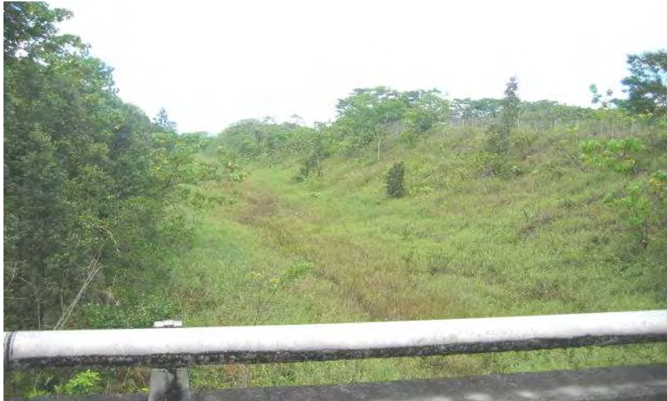
Figure 37. Four Mile Creek looking upstream from Railroad Ave Bridge
