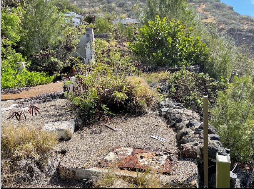
Figure 18. Mortared rock wall on the cliff line, facing northeast.
