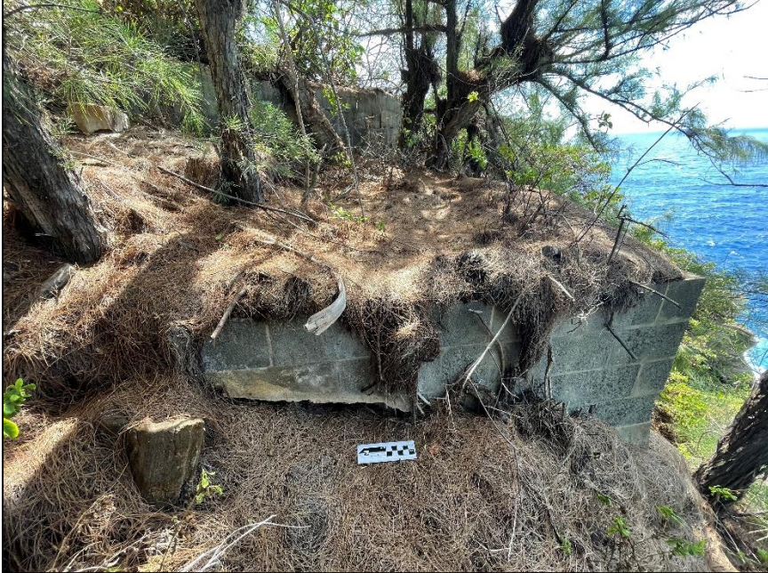
Figure 20. Structural remains on the southeastern slope of the property, facing east.
