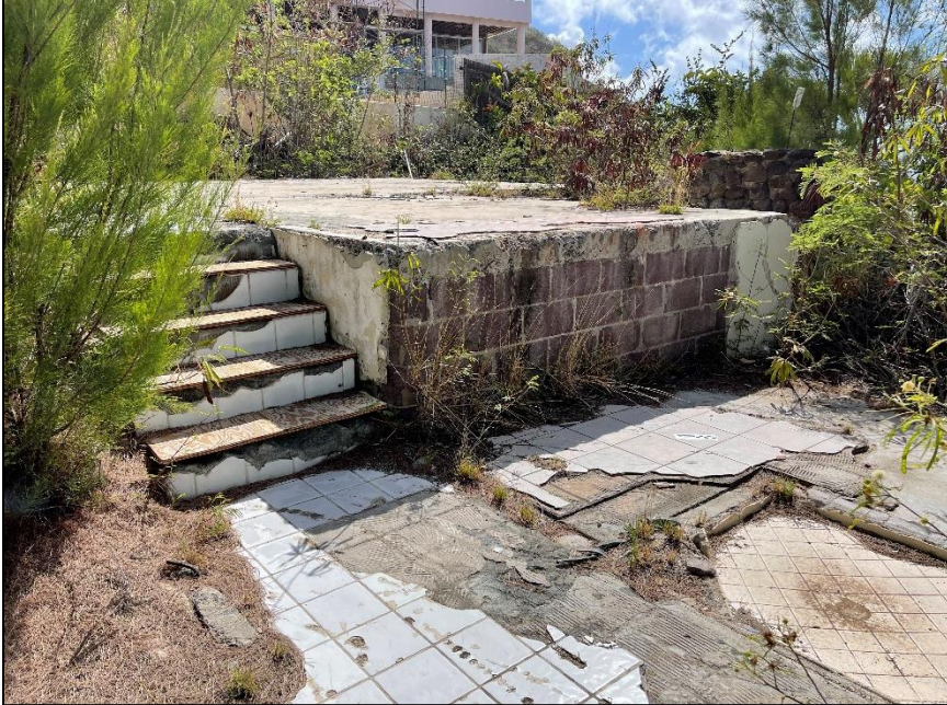
Figure 16. Steps connecting the two tiers of the property, facing east.
