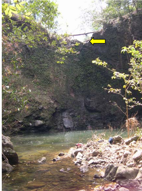
Upstream view of dry waterfall at site gh074r-030508. Note concrete diversion structure (yellow arrow) below fallen tree at the top of the cliff.
