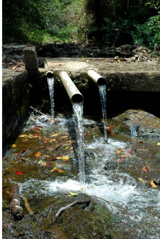
Close up of the three bypass pipes on Haiku diversion.
