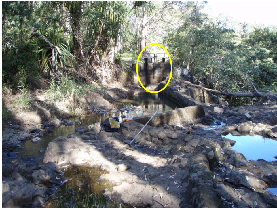
Downstream view of diversion just above the dry water valley in the previous photograph. Note the flume gate (yellow oval) in the middle.
