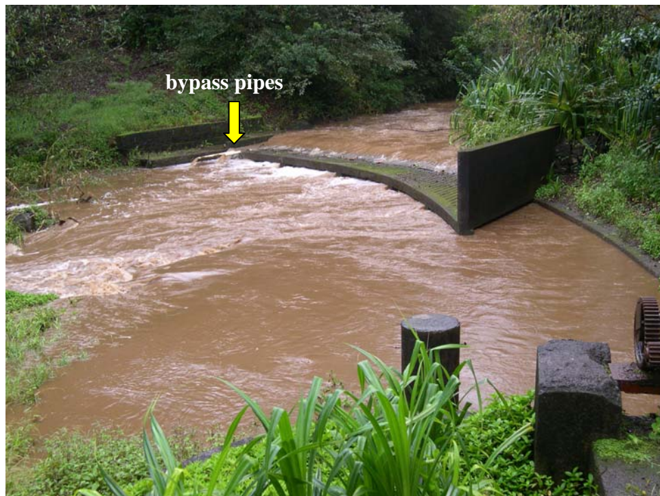
High flood waters over the irrigation ditch with the three bypass pipes. Note the lack of a simple passage way even at these high flows.
