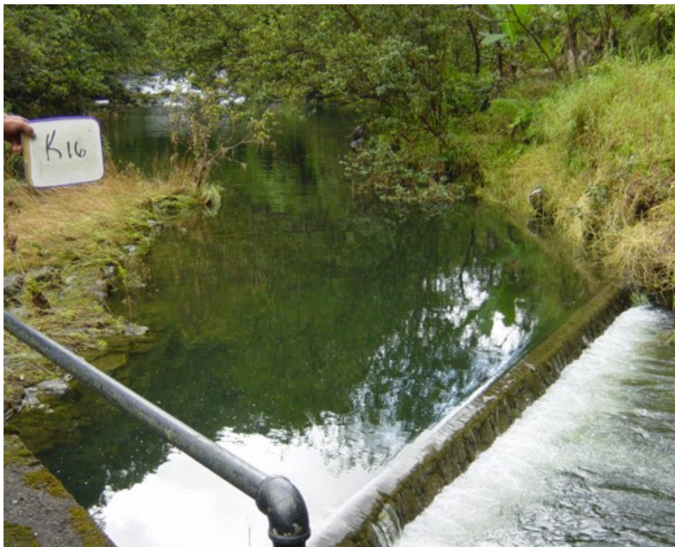
Figure 5-14. Diversion impoundment structure on the upper reach of Wailua Iki East Stream above Hāna Highway. (CWRM diversion photo 288.2).
