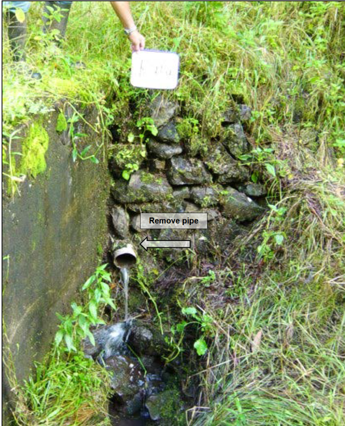
Photo 15a) Eight-inch pipe east of #9 intake at Ko'olau Ditch (K-21a) (2007).
