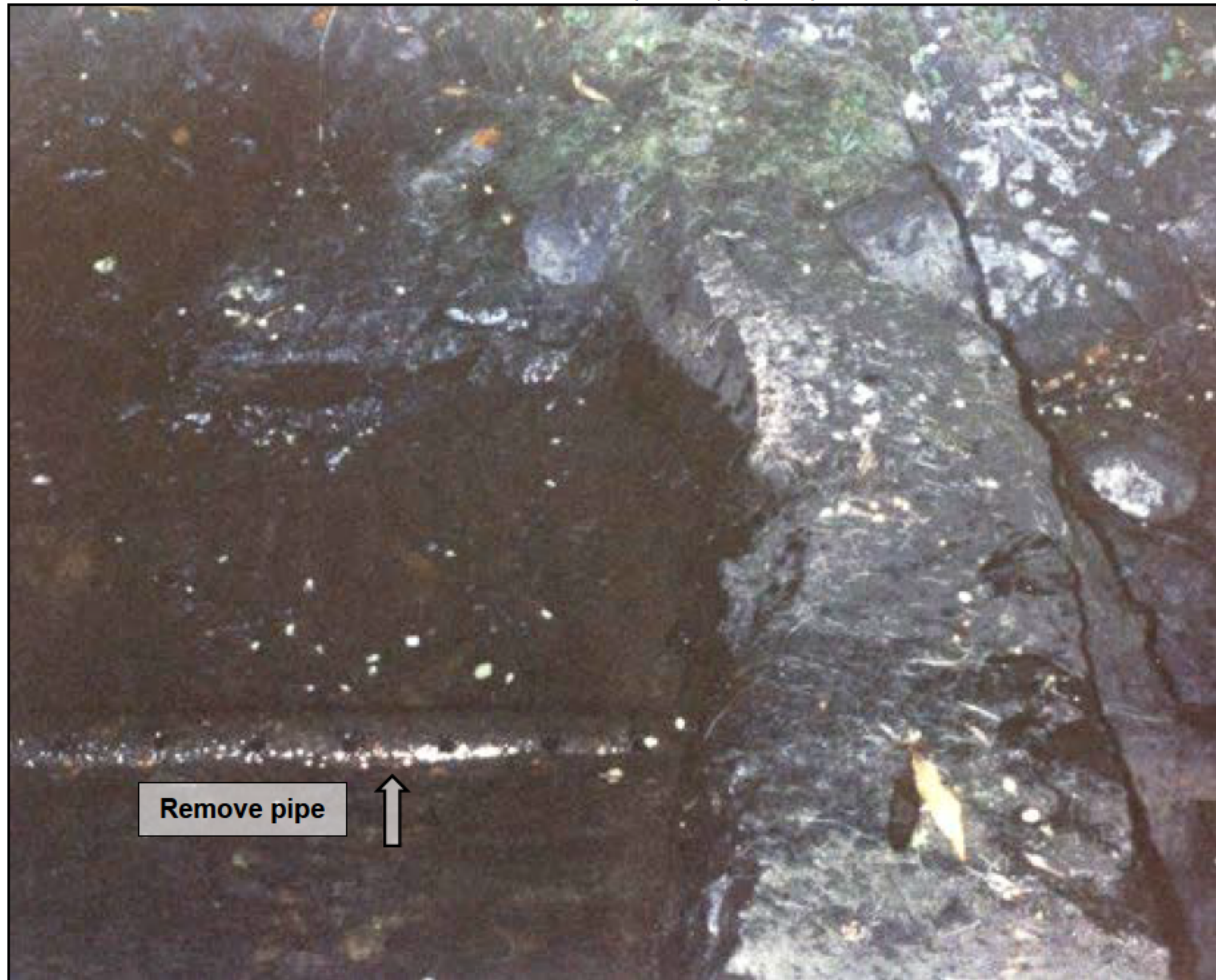
Photo 14. Wailuanui #8 intake at Ko'olau Ditch (K-20a) (1989).
