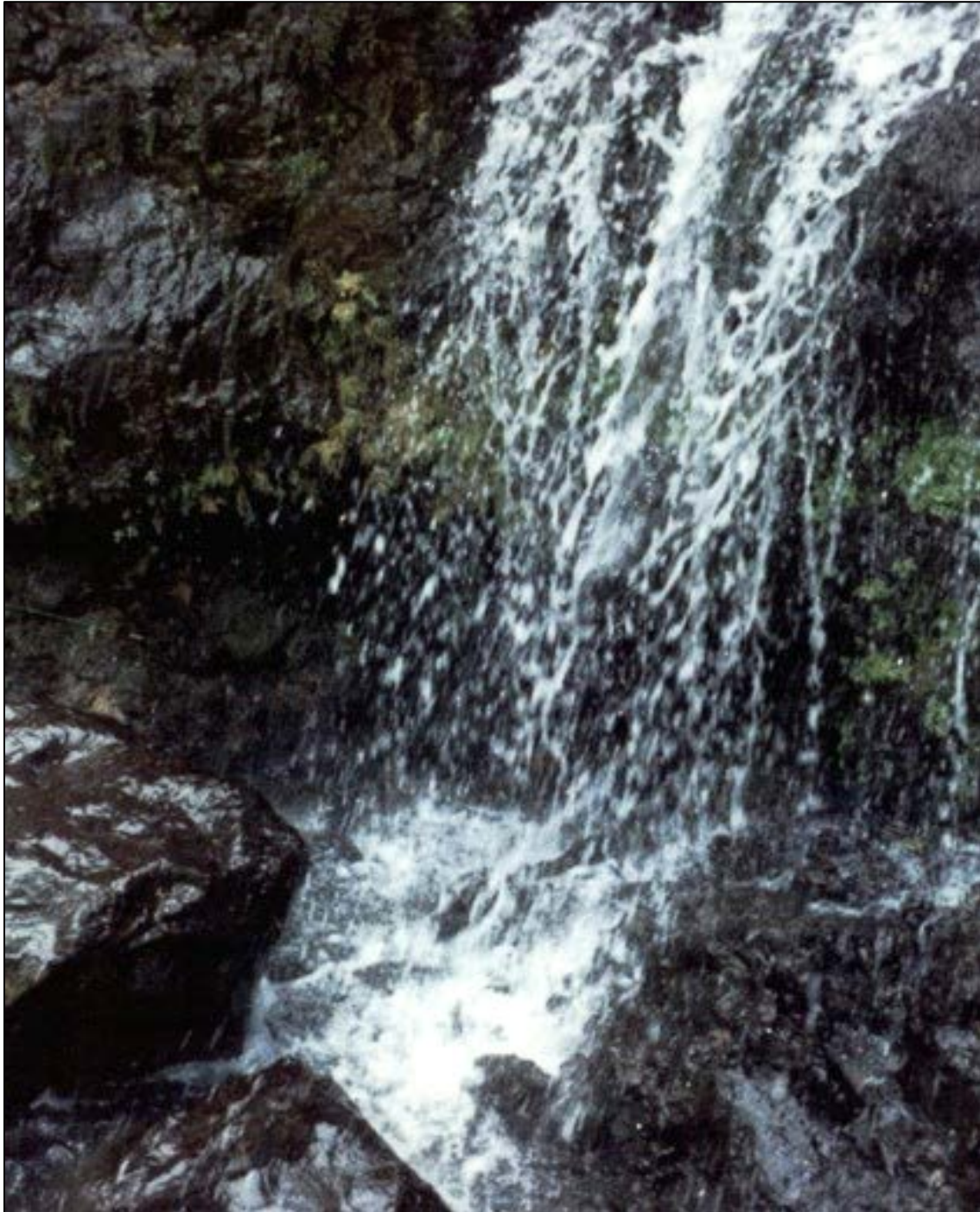
Photo 6. Lalapipi #2 intake at Hauoli Ditch (K-28) (1989).
