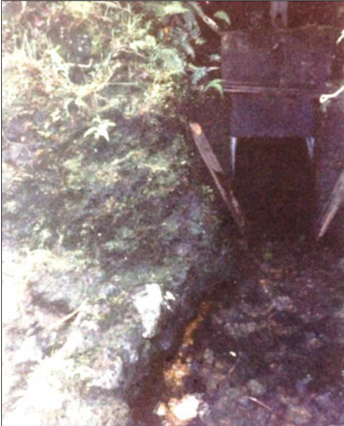
Photo 7. Ka'auau #1 intake at Hauoli Ditch (K-29) (1989).
