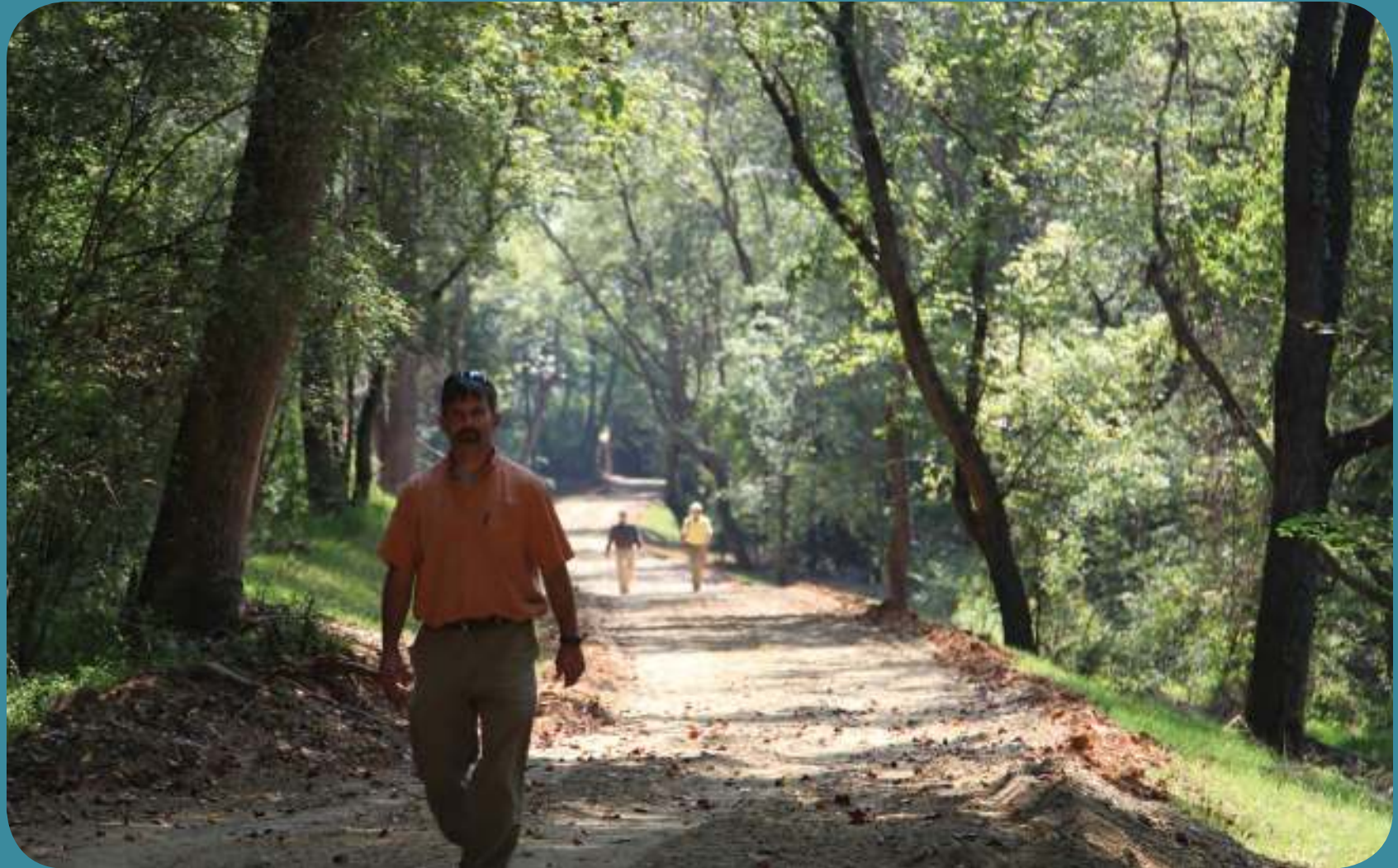
Tim Johnson, NCDPR's Western Regional Trails Specialist, tours newly constructed EVTA trails in Elkin, NC.
