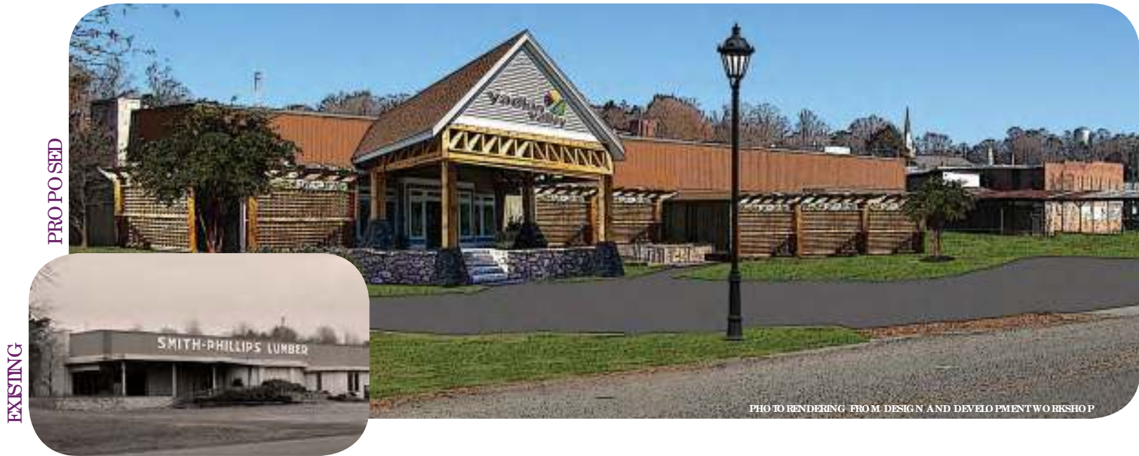
The Heritage and Trails Center will require an adaptive reuse of the old Smith-Phillips building.
