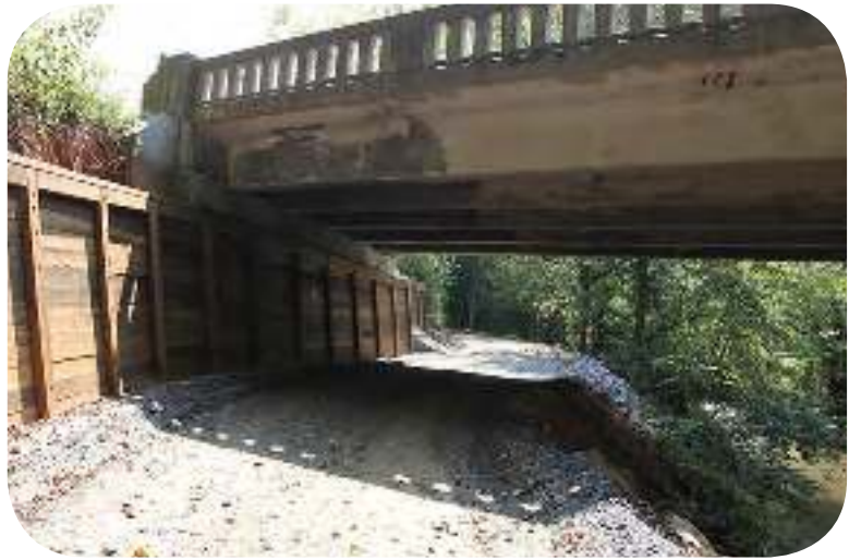
EVTA's work includes this Highway 268 trail underpass.
