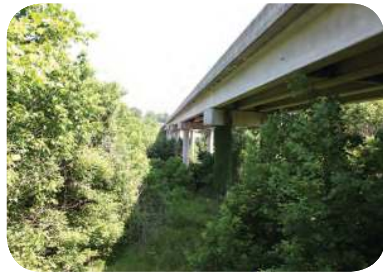
Trail construction is feasible underneath Highway 601.
