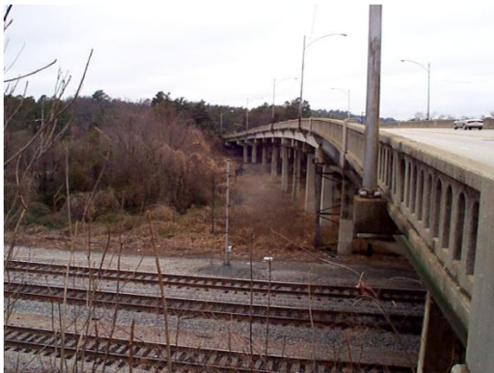
Property No. 49 – Bridge No. 116
