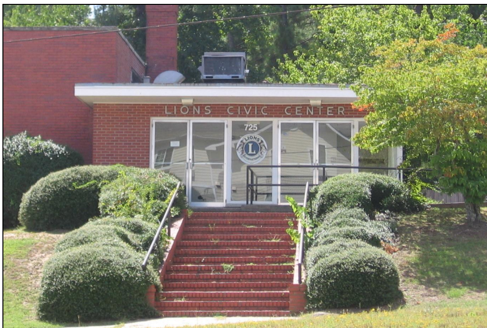
Figure 10. Lions Civic Center – detail of main entrance.
