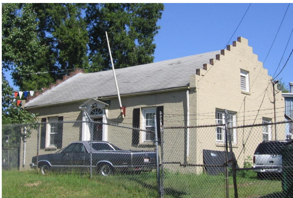
Figure 36. House at #460 West Rowan Street. Main (south) and east elevations.
