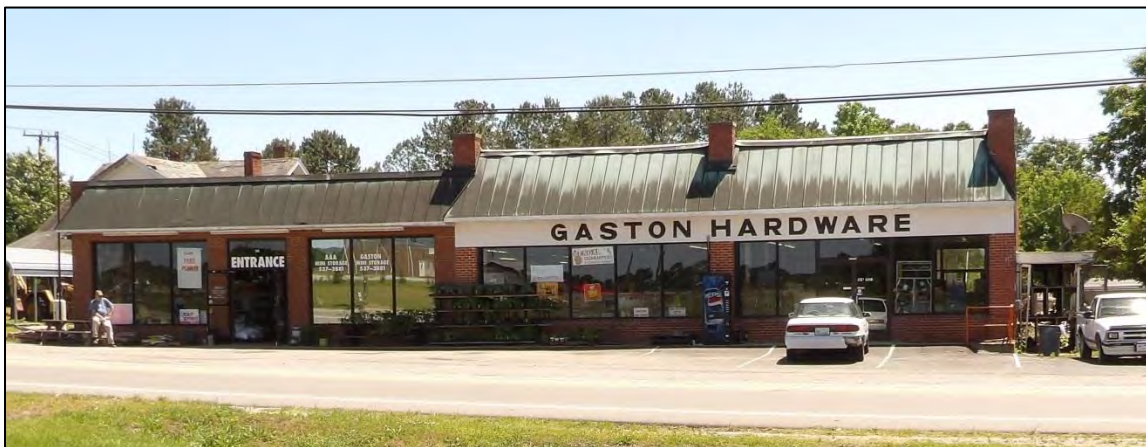
Photo 32: Gaston Hardware Store, North Elevation.
