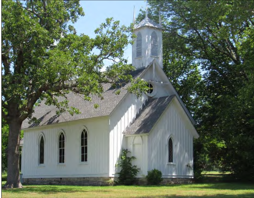
Photo 183: St. James Episcopal Church (VN0010), Southwest Oblique.
