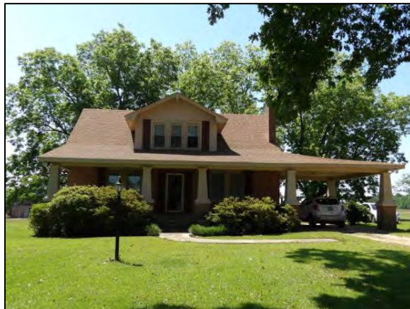
Photo 133: North Façade of the D.R. Allen Farm Dwelling, Looking South.
