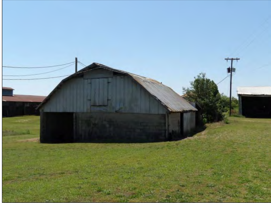
Photo 147: Dairy Barn, Looking South.
