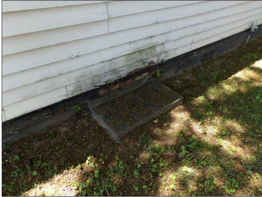
Photo 106: Detail of Foundation on West Elevation.
