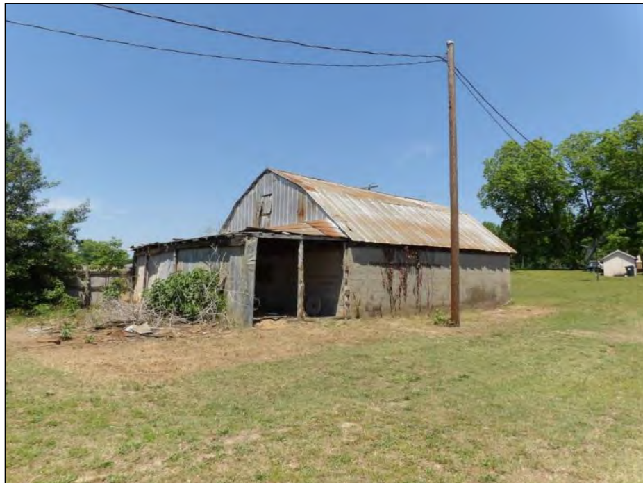
Photo 148: Dairy Barn, Southeast Oblique.
