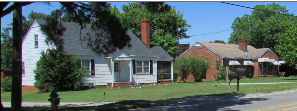
Photo 8: View of 307 and 305 Lawrenceville Road (N.C. Highway 46), Looking Northeast.
