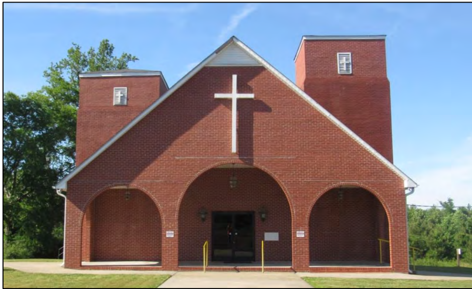
Photo 47: North Elevation Showing the Late 1990s Narthex, Brick Arcade, Recessed Entryway, and Tower Modifications.
