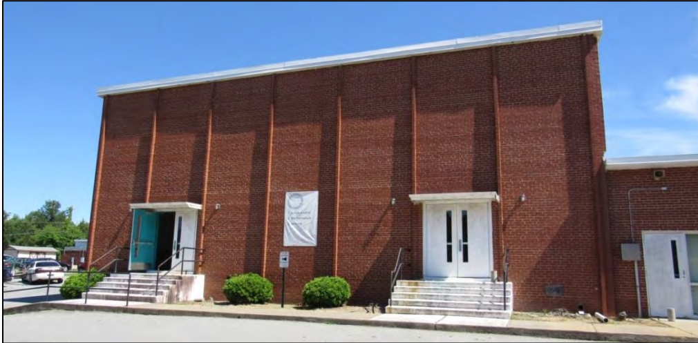
Photo 67: 1964 Gymnasium/Cafeteria Addition, South Elevation.
