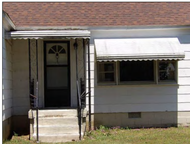
Photo 120: Detail of the Main Entry and Picture Window, Looking North.
