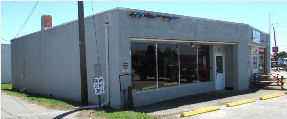
Photo 42: 105 Garysburg Road (N.C. Highway 46), Northeast Oblique.
