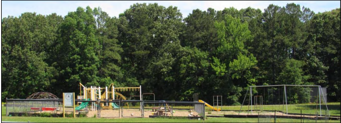
Photo 77: Playground (Circa-1990 and Circa-2005 Sections) Looking North.
