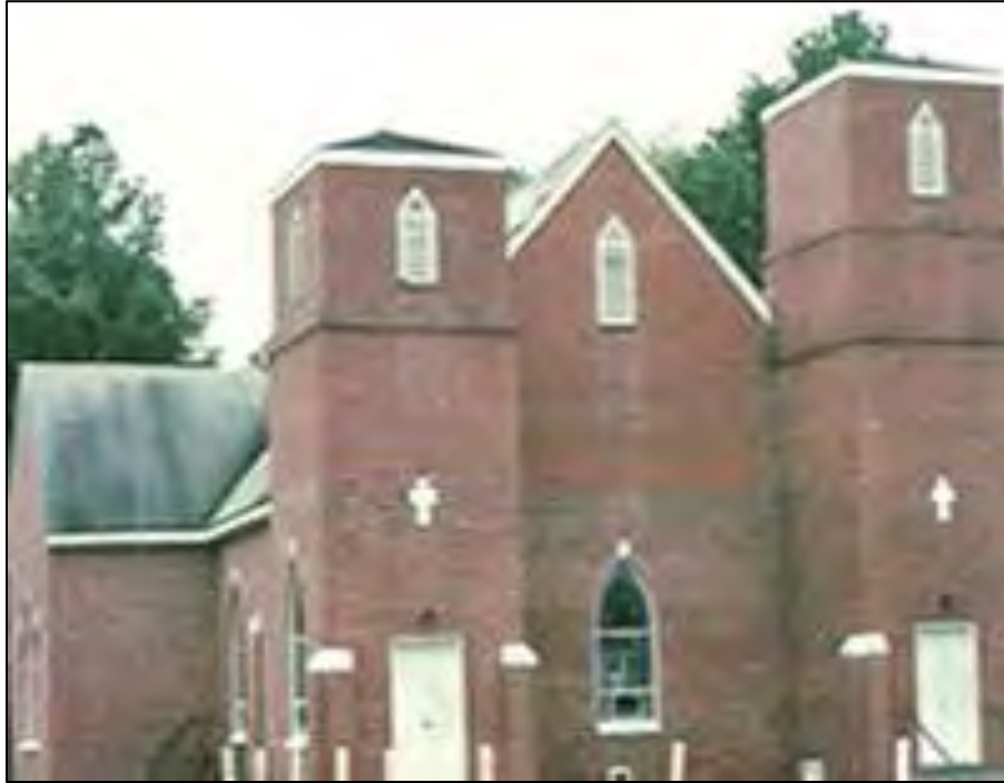
Photo 45: Northeast Oblique of the Cool Spring Baptist Church before the Late-1990s Narthex Addition. 102
