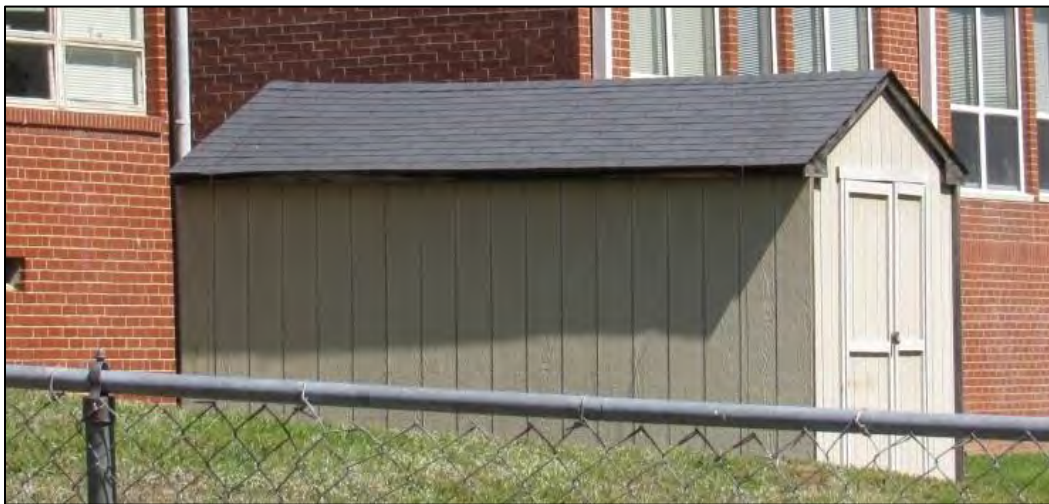
Photo 76: Southeast Oblique of the Circa-2005 Shed.
