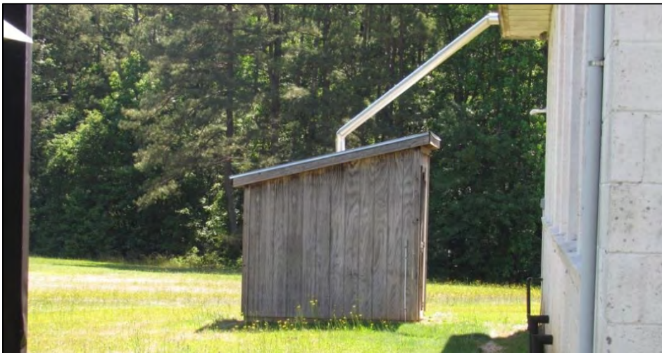
Photo 72: Cistern, West Elevation.
