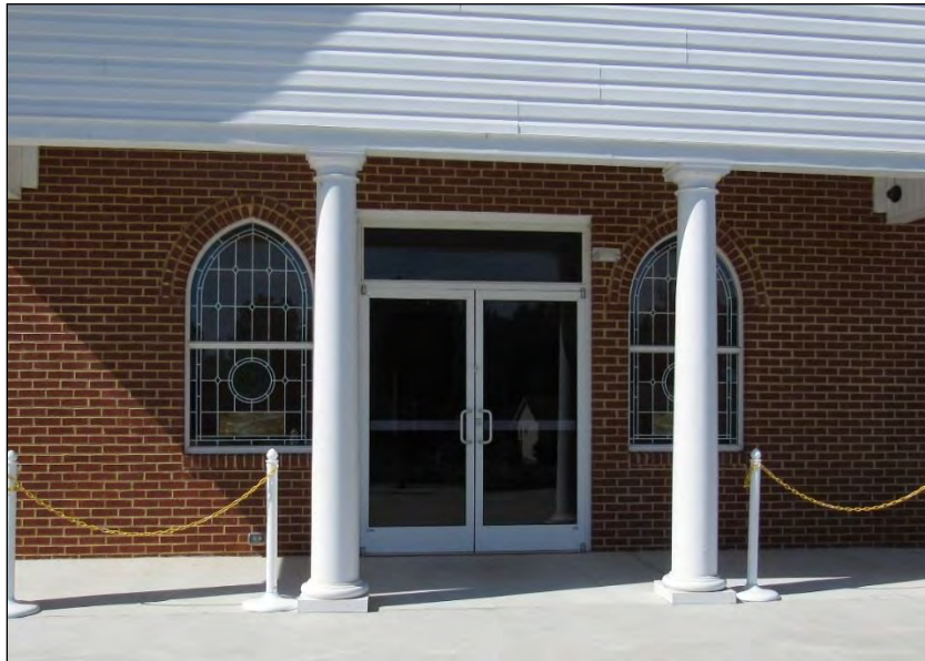
Photo 185: Gaston Baptist Church, Entry Detail.
