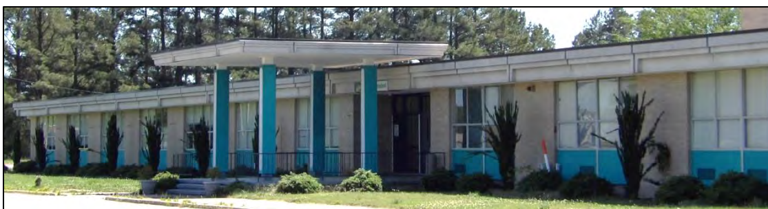
Photo 86: Northampton County (East) High School (NP1028) Entrance Detail, Looking South.
