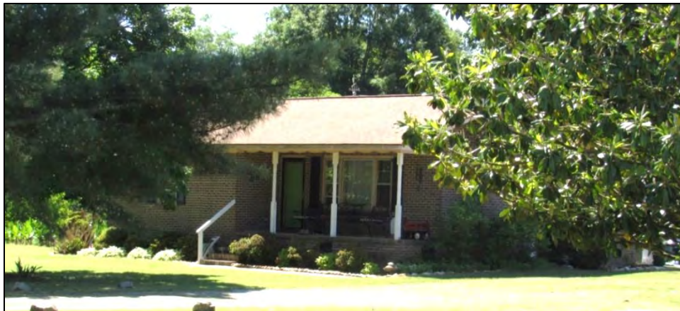
Photo 101: 4564 N.C. Highway 46, North Elevation.
