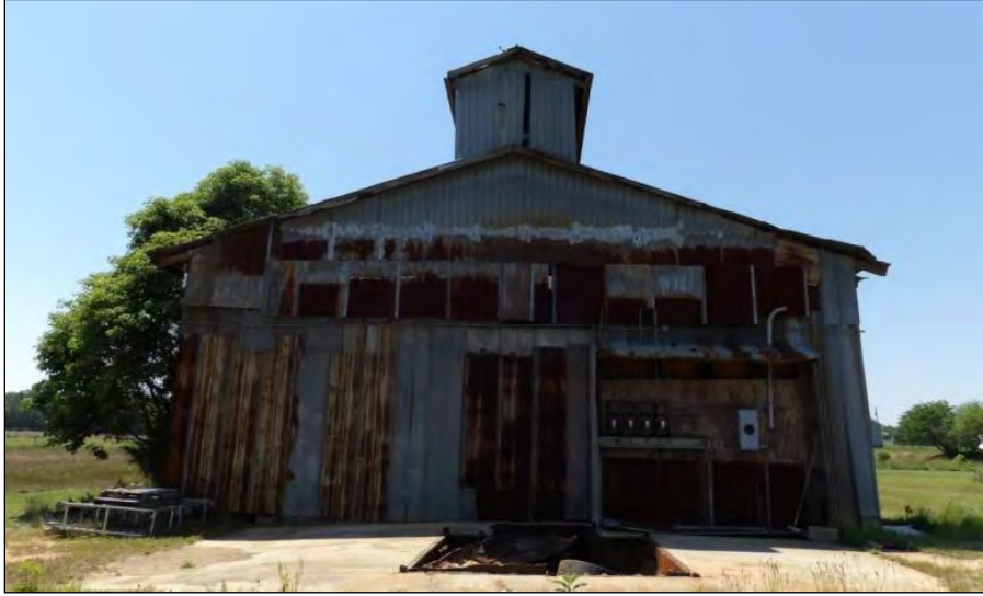
Photo 153: Peanut Warehouse, Looking South.
