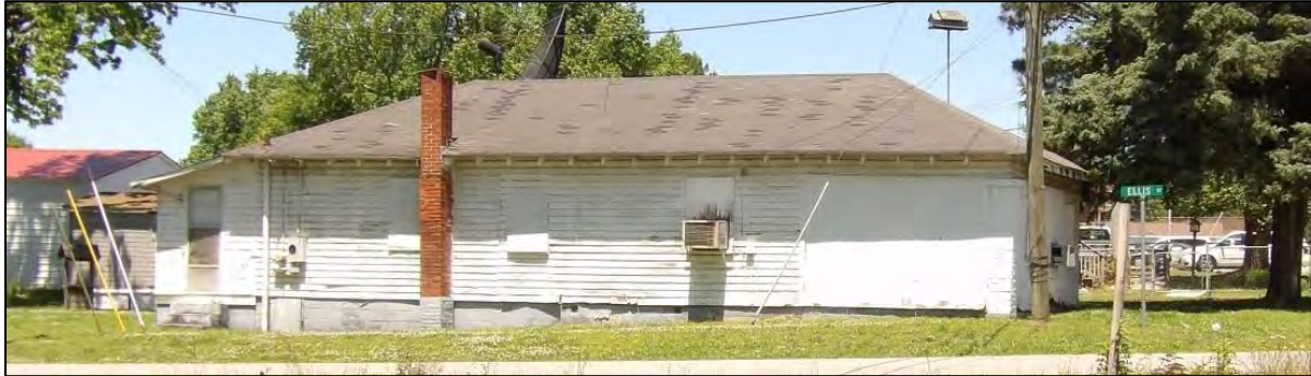
Photo 15: View of Probable Gas Station, 303 Craige Street, South Elevation.
