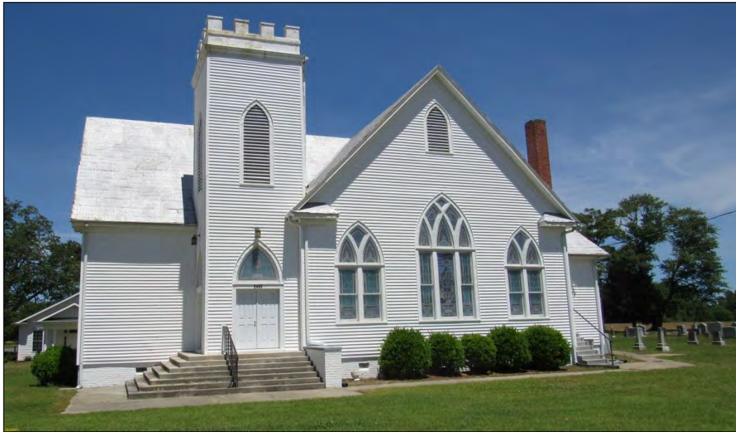
Photo 182: Pleasant Grove United Methodist Church (NP0246), South Elevation.
