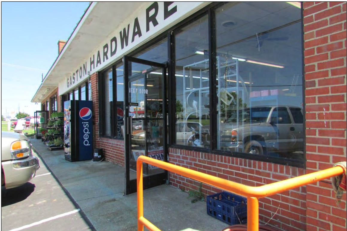
Photo 35: Detail of Storefront Windows at Gaston Hardware Store, Looking East.
