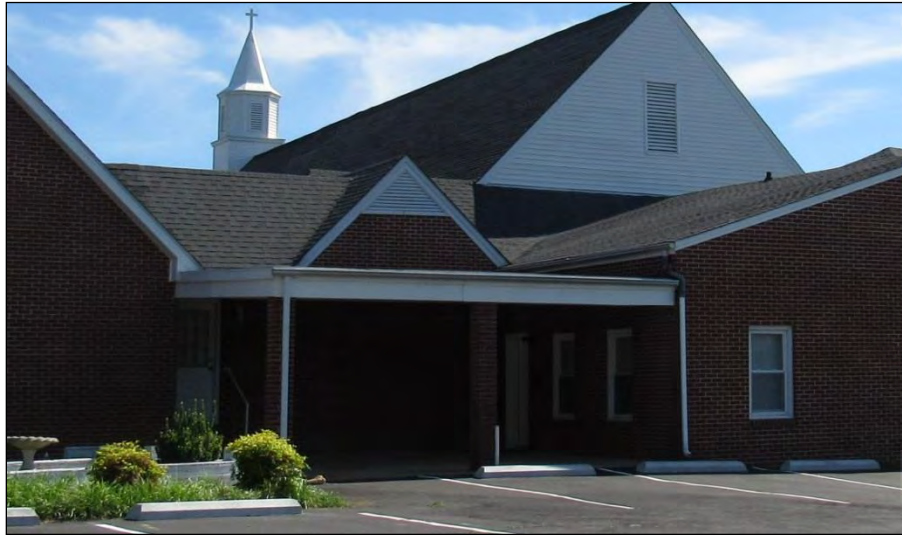
Photo 188: Circa-2010 Addition, Southwest Elevation.
