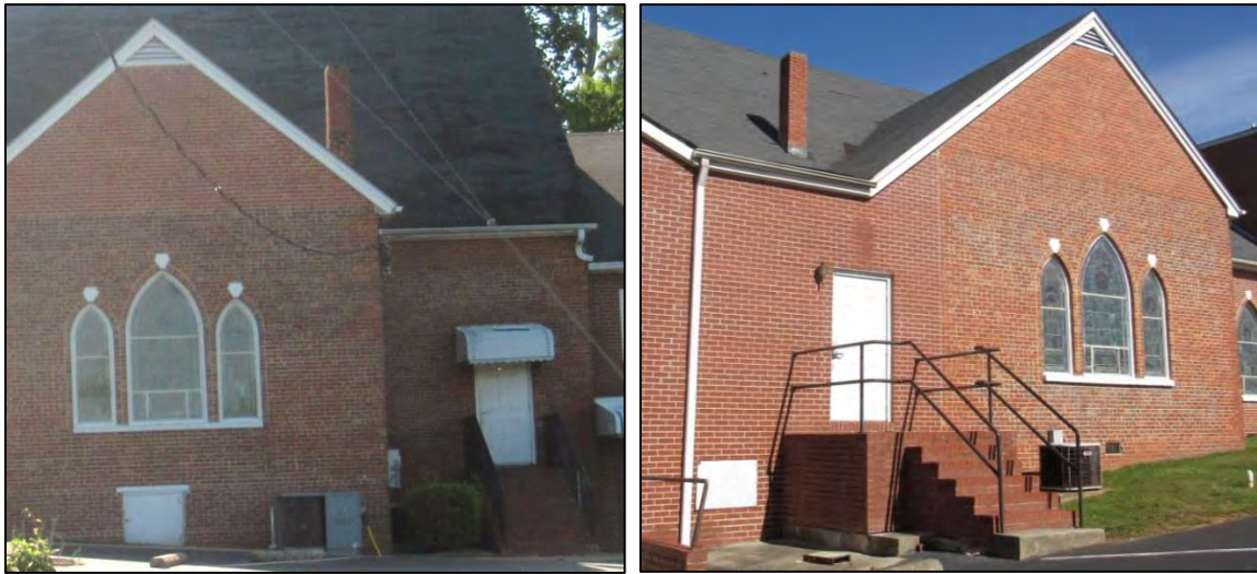
Photo 49: Secondary Entrances on the East (Left) and West (Right) Elevations.
