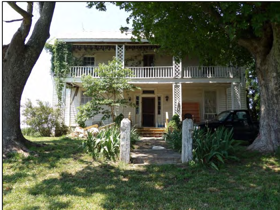
Photo 165: Dwelling, Southeast Elevation.
