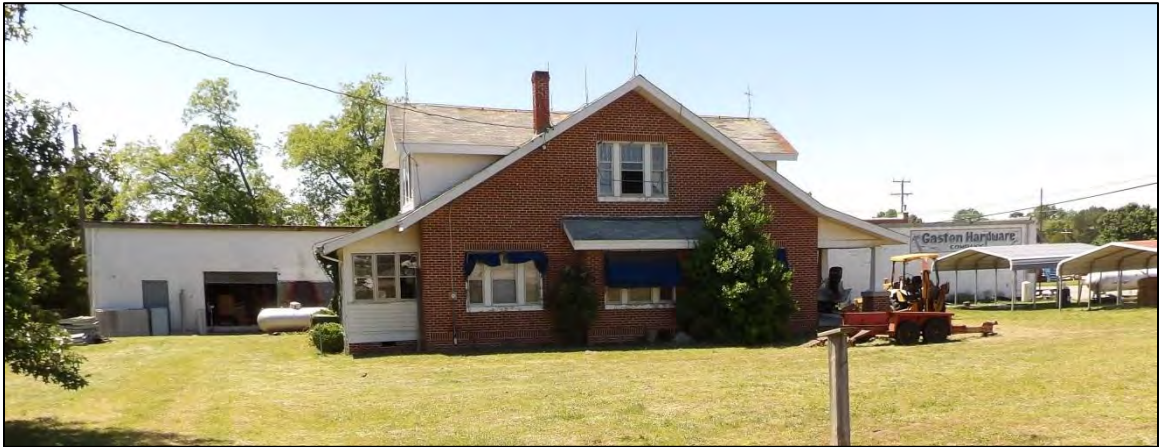
Photo 34: East Elevation of Store Showing Circa-1990 Addition Taken from Reid Street.
