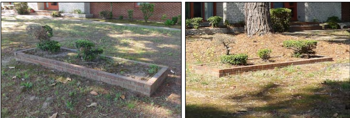
Photo 98: Two of the Brick Plant Boxes North of the House.
