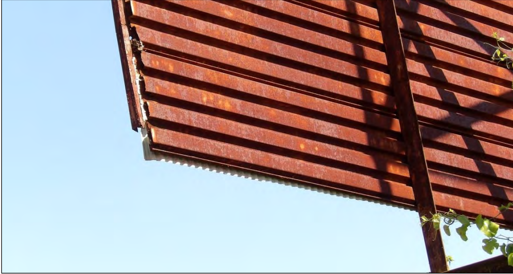
Photo 24: Detail of North Bottom Corner of Screen Showing Construction.
