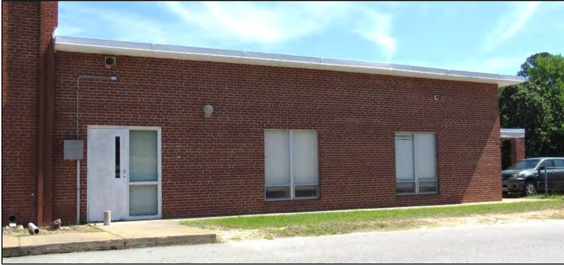
Photo 69: South Elevation of the Circa-1975 One-Story Addition.
