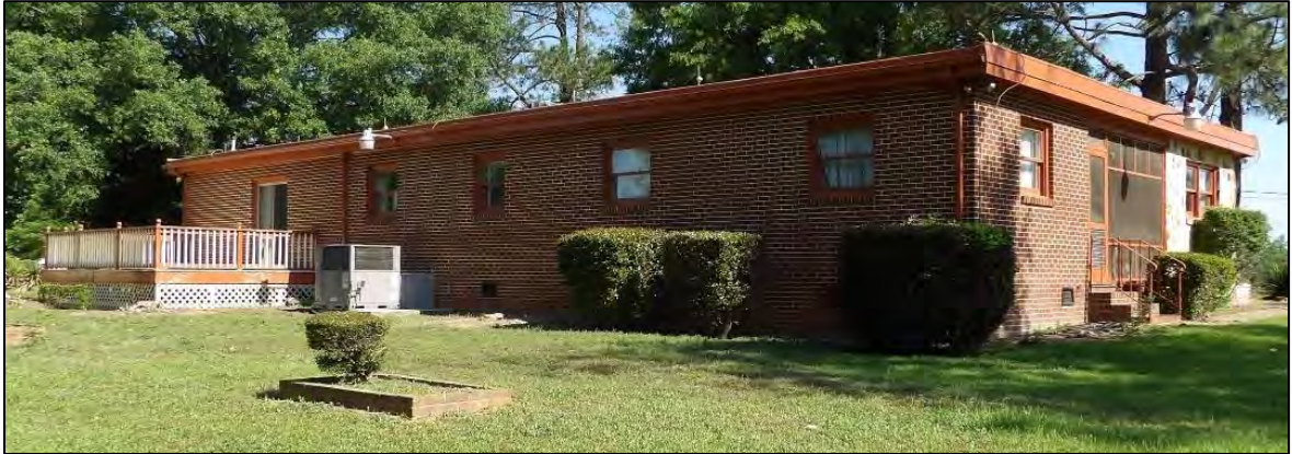
Photo 91: Southeast Oblique of the Jasper and Betty Jones House.
