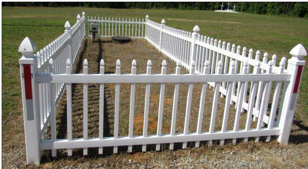
Photo 193: Utility Area, Looking South.
