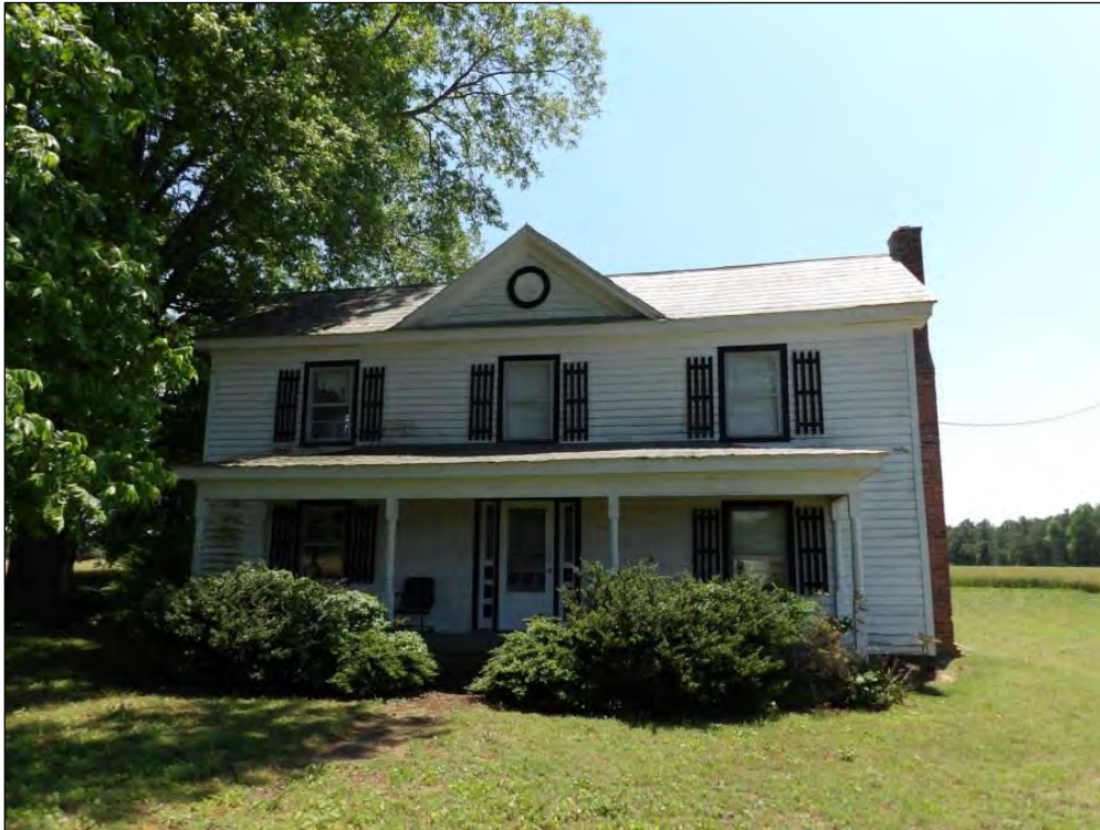
Photo 105: View of Façade of the I-House, Looking South.
