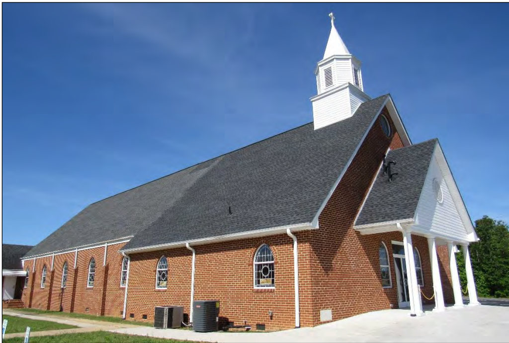
Photo 184: Gaston Baptist Church, North Oblique (Top) and East Oblique (Bottom).
