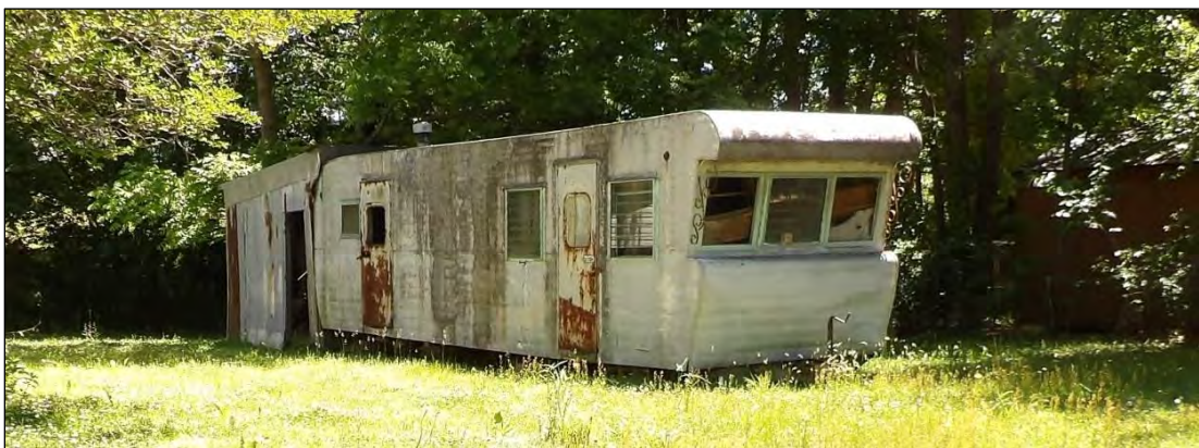
Photo 11: View of Circa-1955 Mobile Home on South Bay Street, Looking Southeast.
