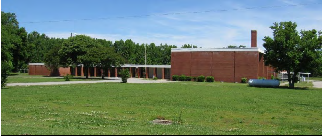
Photo 82: Garysburg Elementary School (NP1119), Southeast Oblique.
