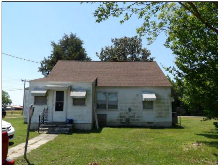
Photo 123: North Elevation, Looking South.
