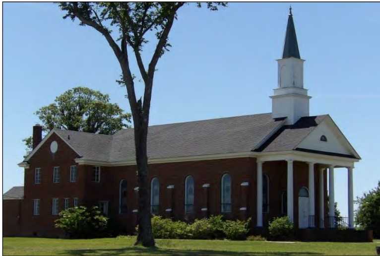
Photo 199: Sharon United Methodist Church (NP0828), East Oblique.
