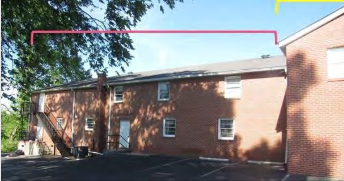
Photo 53: West Elevation of the Church. The circa-1970 addition is noted in yellow and the circa-1985 addition is noted in pink.
