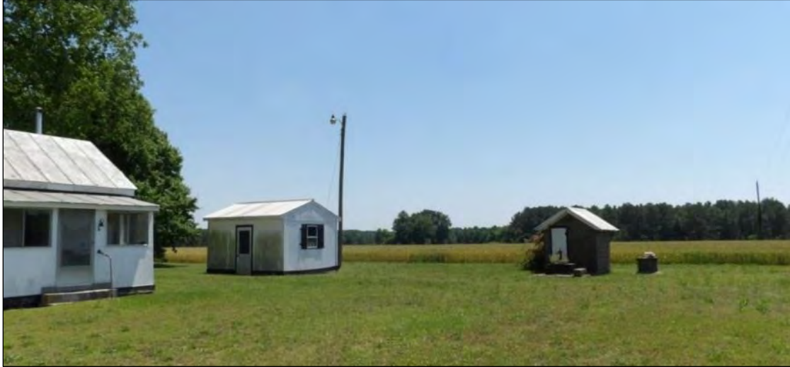
Photo 111: View of the Associated Outbuildings and Well, Looking Southeast.
