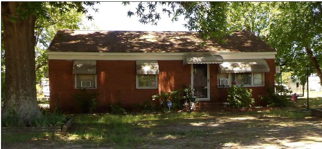
Photo 10: House at 206 Davie Street, South Elevation.
