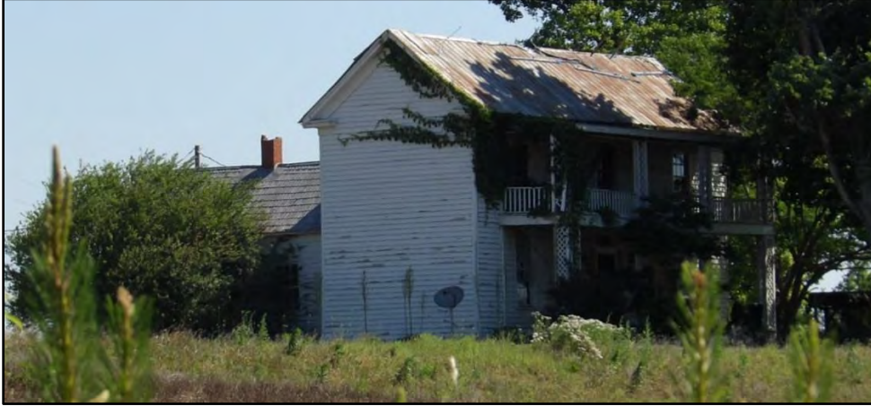
Photo 163: Dwelling, South Oblique Overview Featuring Rear Ell Addition.
