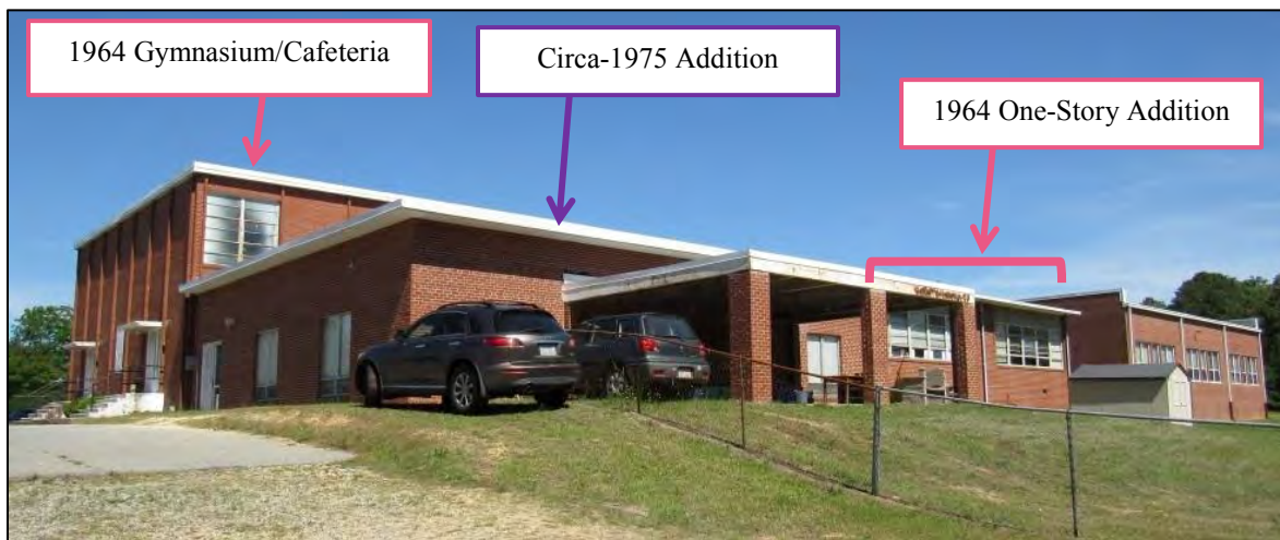
Photo 68: Southeast Oblique of the 1964 Gymnasium and One-Story Addition (Pink) and Circa-1975, One-Story Addition (Purple).
