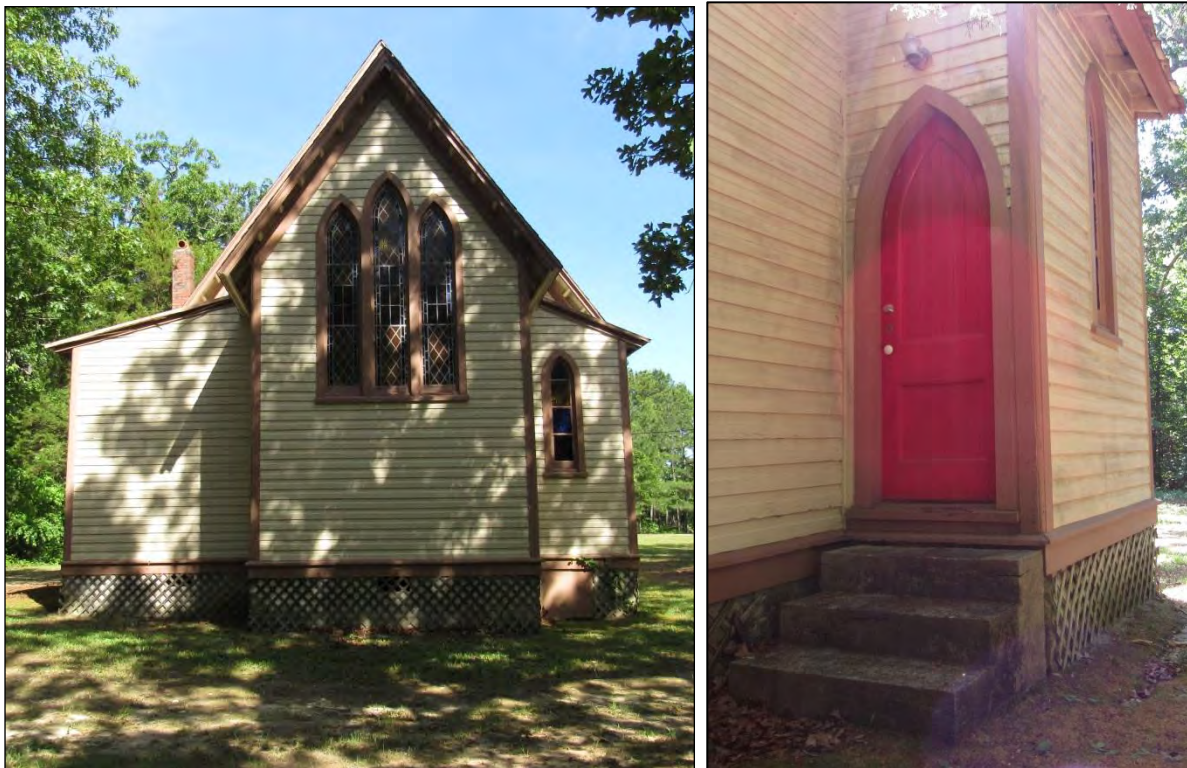
Photo 179 St. Luke's Church Southeast Elevation (Left) and Secondary Entry Detail (Right).
