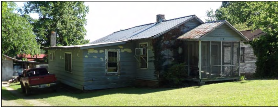
Photo 4: House at 103 East Hill Street, Northeast Oblique.
