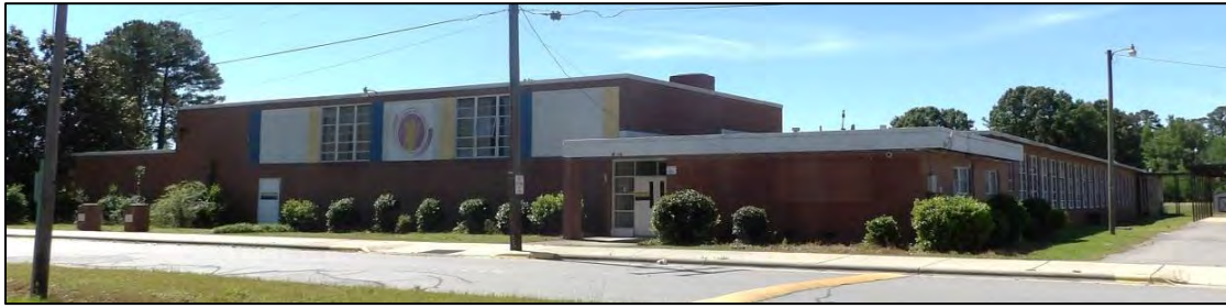
Photo 84: W.S. Creecy School (NP0959), Northwest Oblique.
