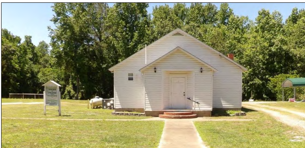
Photo 13: Doors of Praise and Worship Church on South Bay Street, East Elevation.
