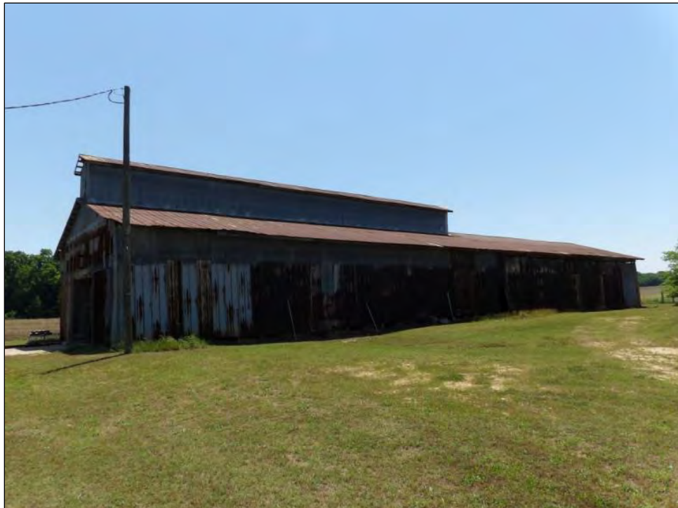
Photo 152: Peanut Warehouse, Looking Southeast.
