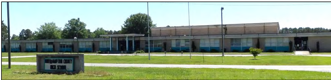
Photo 85: Northampton County (East) High School (NP1028), Northeast Elevation.
