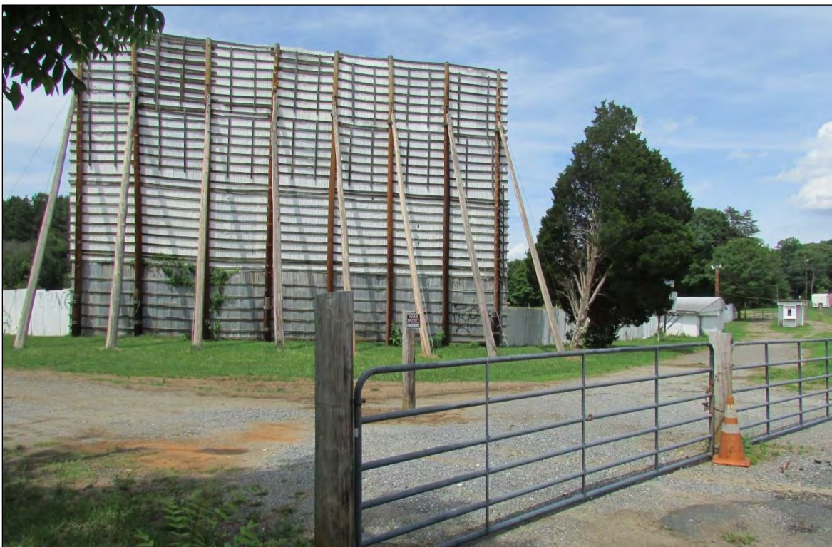
Photo 31: View of Screen and Ticket Booth at Belmont Drive-In Theatre, McAdenville Road, Belmont, North Carolina. Screen displays pole-type construction exhibited by a majority of drive-in screens throughout the state.
