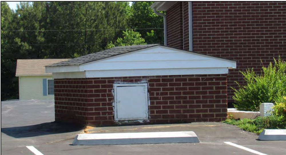
Photo 191: Well House, Southwest Oblique.
