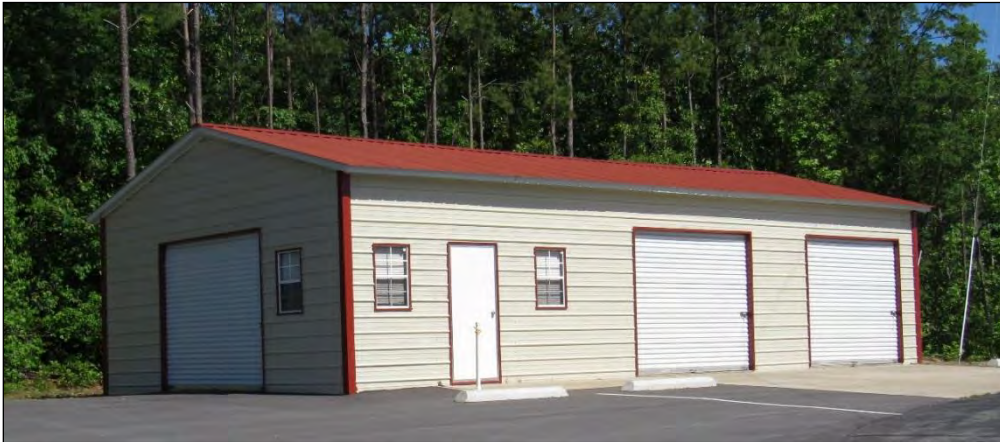
Photo 190: Garage, South Oblique.
