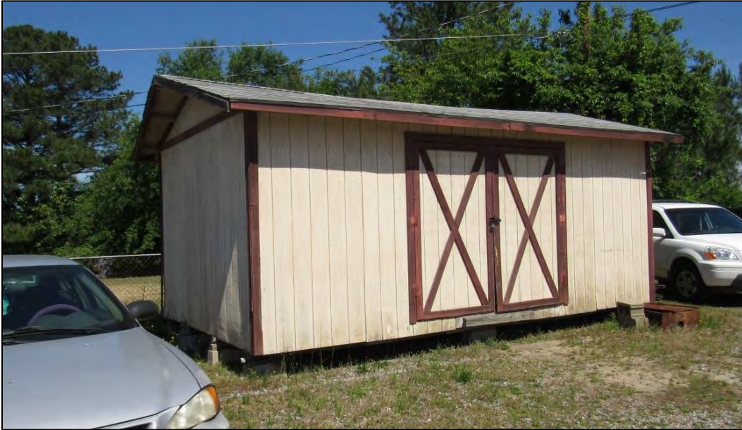
Photo 75: Southeast Oblique of the Circa-1995 Shed.
