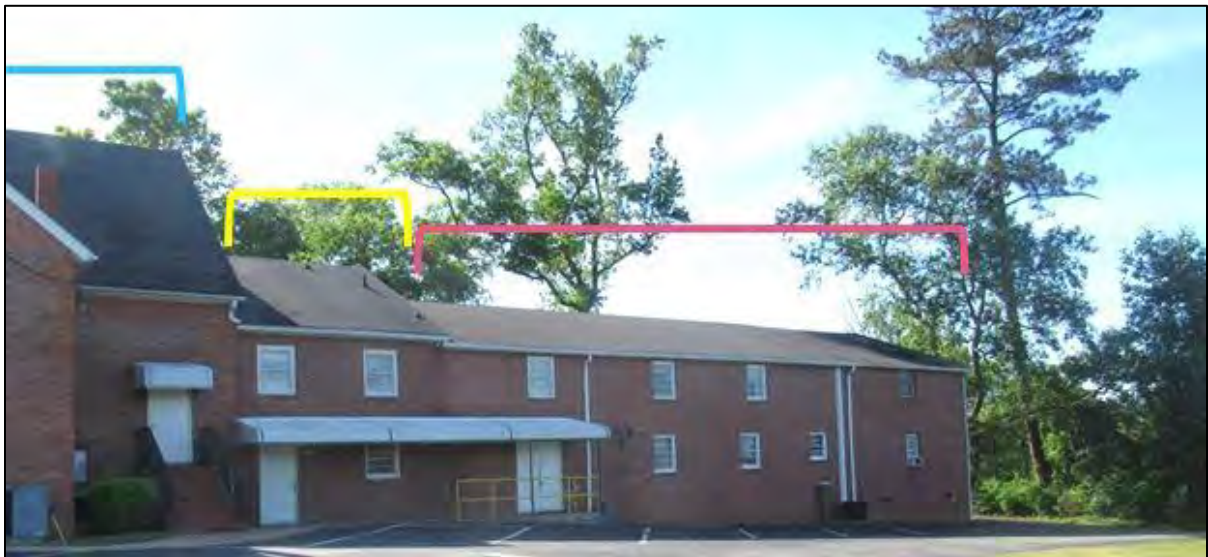
Photo 52: Cool Spring Baptist Church West Elevation Showing the Original Core (Blue), Circa-1970 Addition (Yellow), and Circa-1985 Addition (Pink).
