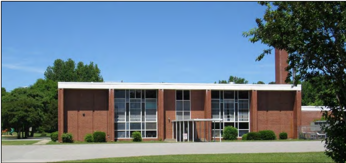
Photo 83: Garysburg Elementary School (NP1119), East Elevation.
