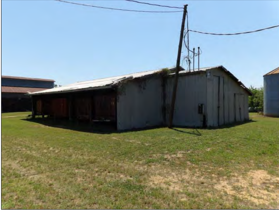
Photo 149: Six-Bay Equipment Shed, Northwest Oblique.
