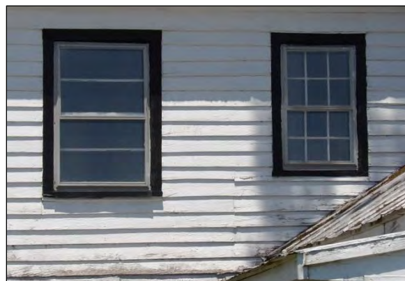
Photo 109: Window Detail on Rear Elevation.
