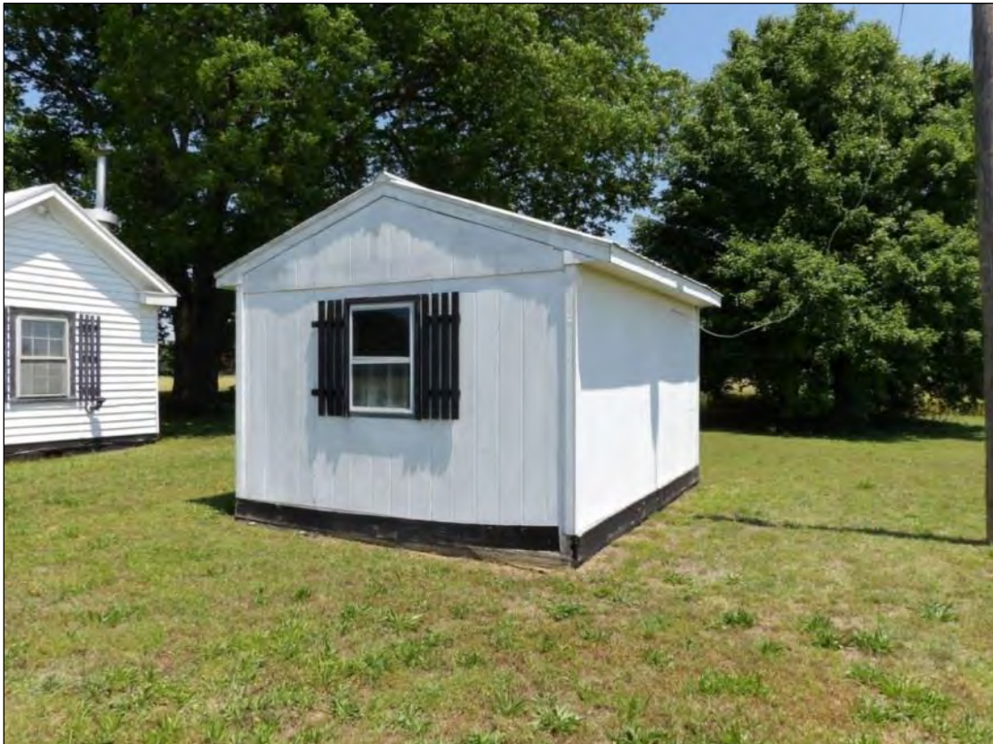
Photo 112: Shed, Southwest Oblique.
