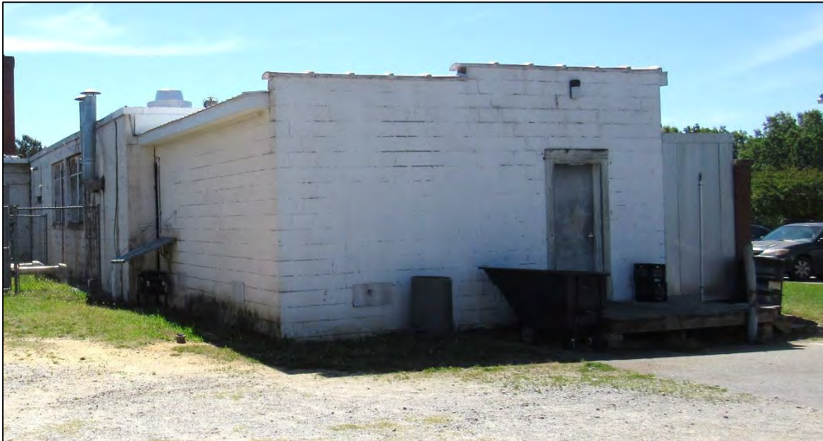
Photo 70: Northwest Oblique of the 1970s Concrete-Block Addition.
