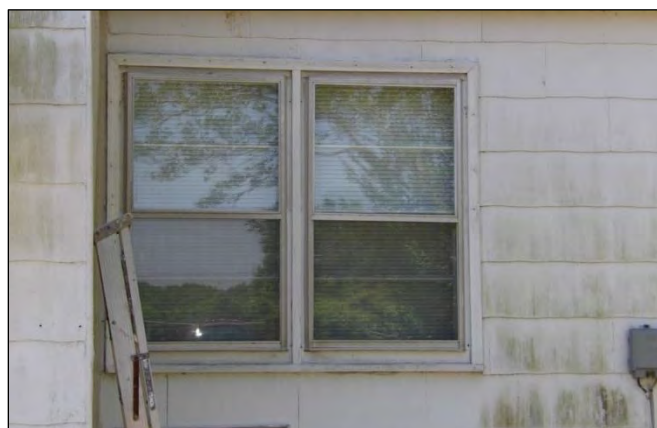
Photo 121: Window Detail on North Elevation, Looking South.
