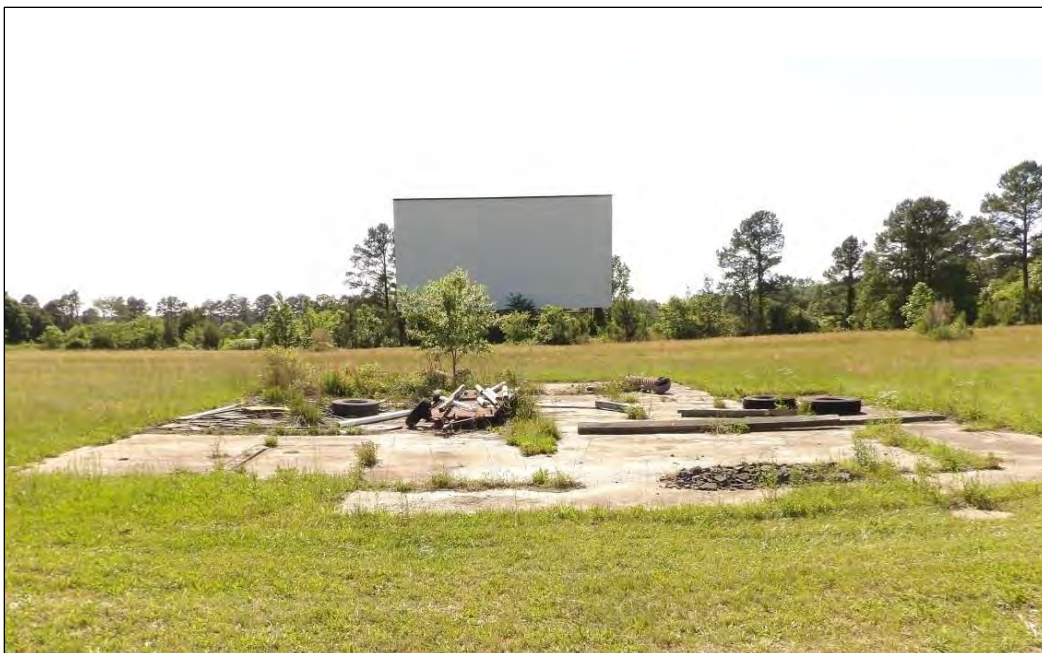
Photo 25: View of Projector House Foundation and Screen, Looking West.
