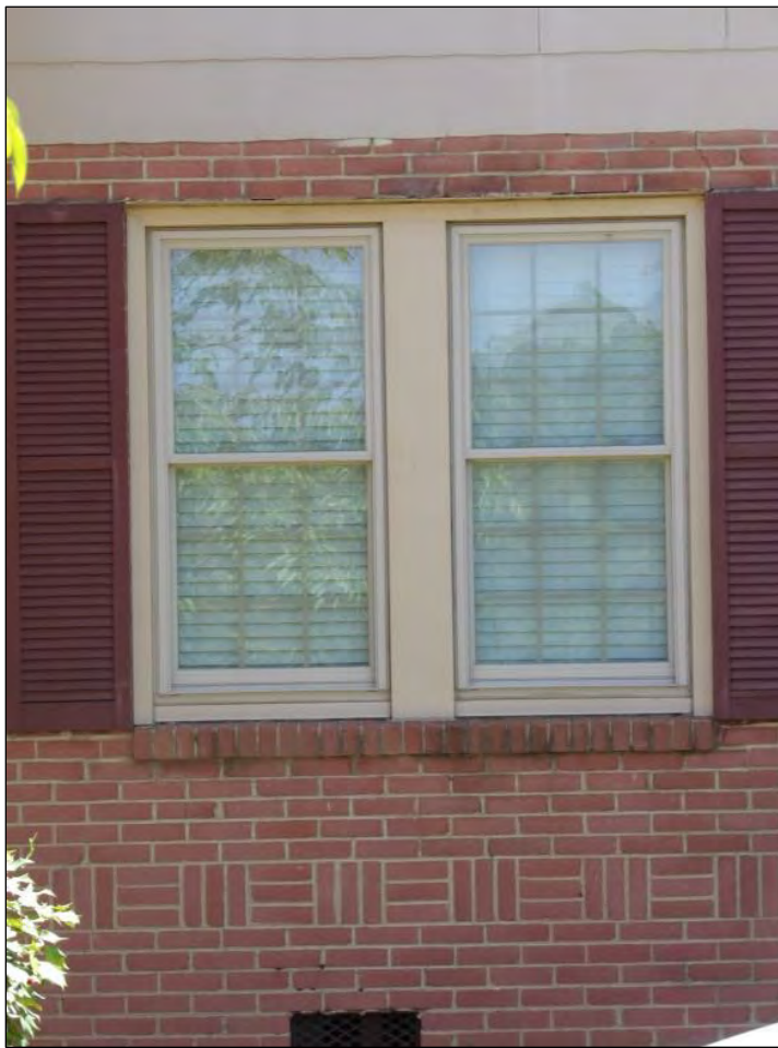
Photo 134: Window and Brick Details, Looking East.
