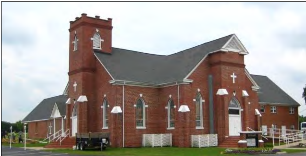
Photo 58: Early-2000s Photograph of the Roanoke Salem Baptist Church (NP0405) Showing the Original Tower Top. 129
