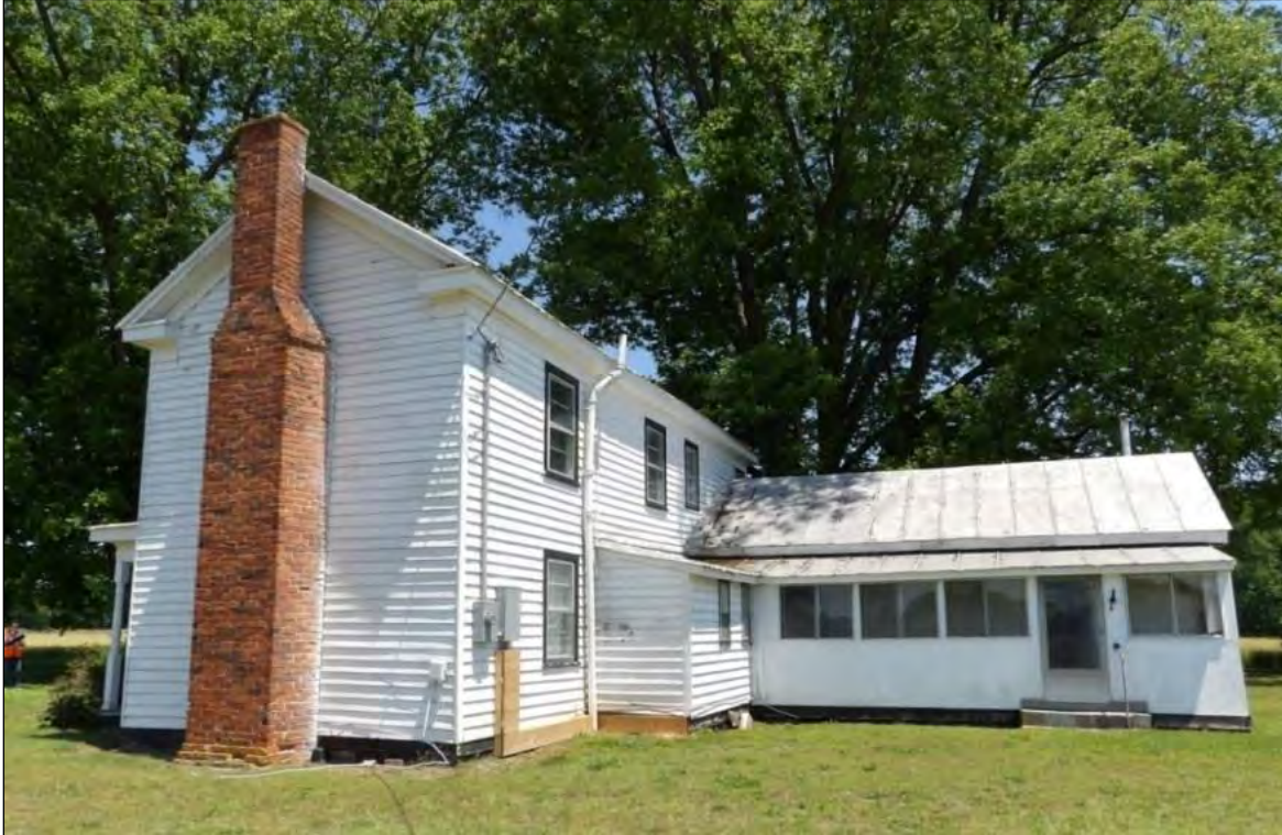
Photo 110: I-House, Southwest Oblique.
