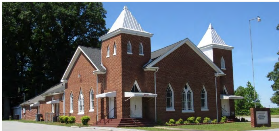
Photo 60: Oak Grove Baptist Church (NP0431), East Oblique.
