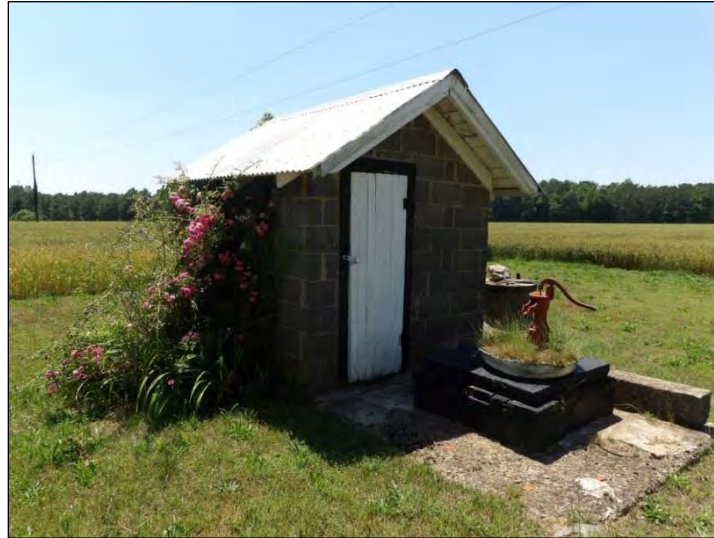
Photo 113: View of the Pumphouse in the Foreground and the Well in the Background, Looking Southwest.
