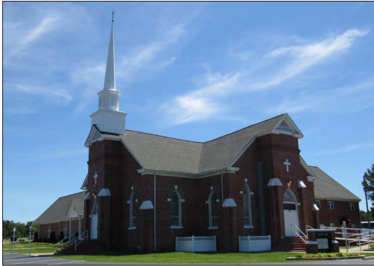
Photo 198: Roanoke Salem Baptist Church (NP0405), West Oblique.
