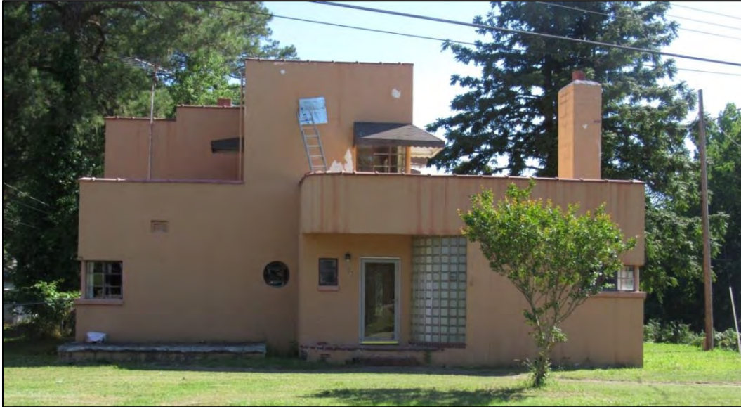
Photo 102: The Benjamin Mills, Jr. House (HX0912), North Elevation.
