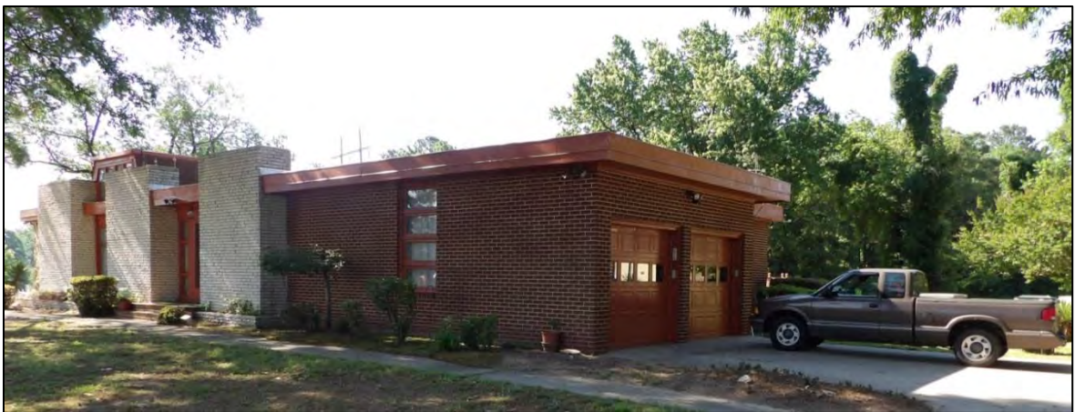
Photo 92: Northwest Oblique Showing the Garage Doors.
