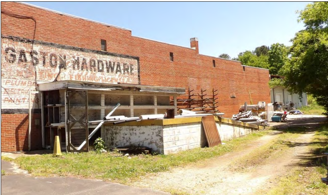
Photo 37: View of Loading Dock and Frame Shelving Unit, Looking Southeast.
