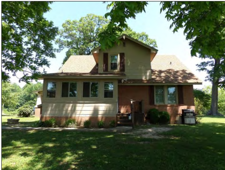
Photo 138: Rear Elevation Looking North.
