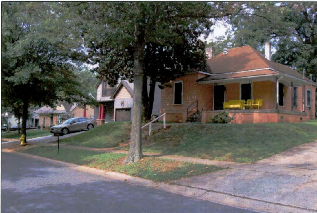
Looking south down North Summit Avenue with altered 325 North Summit (1926) at right and 317 through 301 North Summit (all 1987) to left
