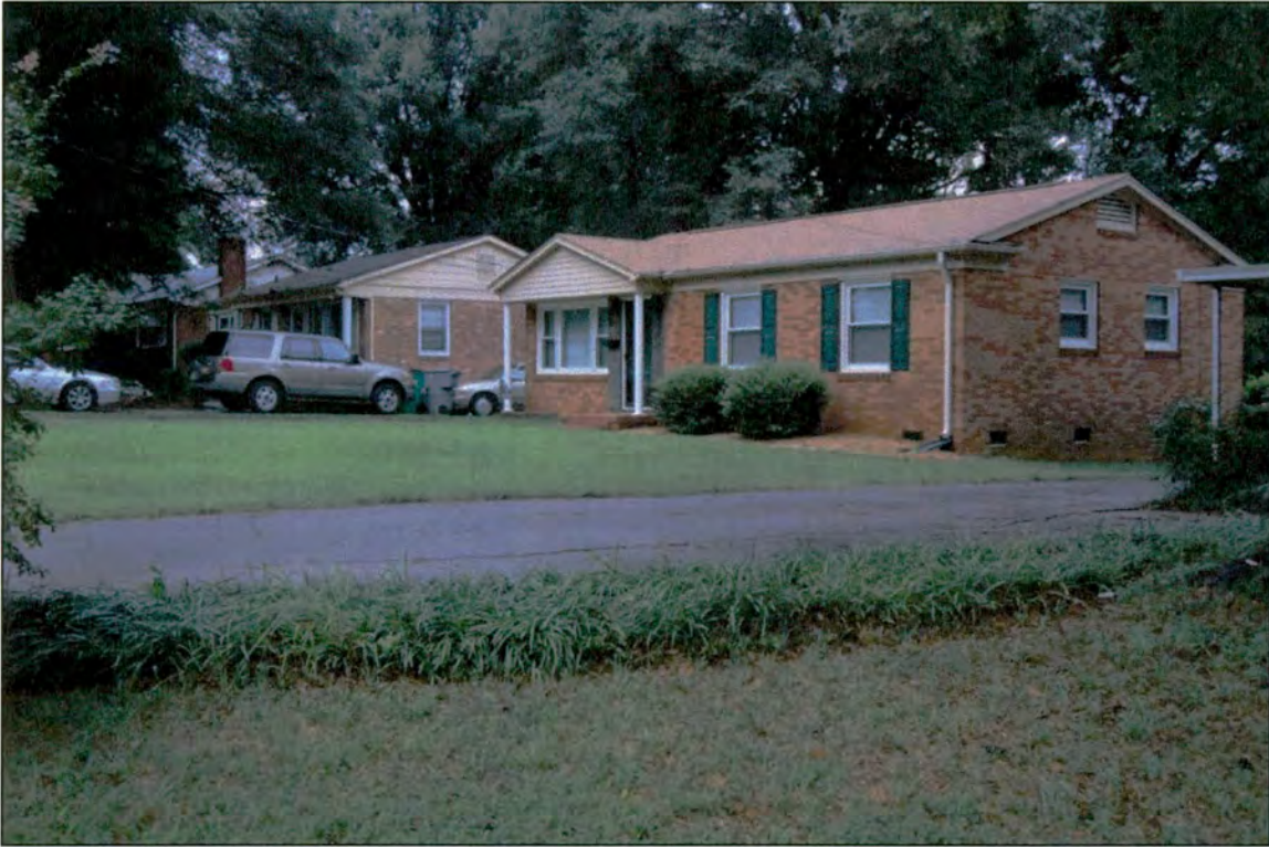
1422 Waddell Street (1957), at right, and 1426 Waddell (1957), at left, (within APE)
