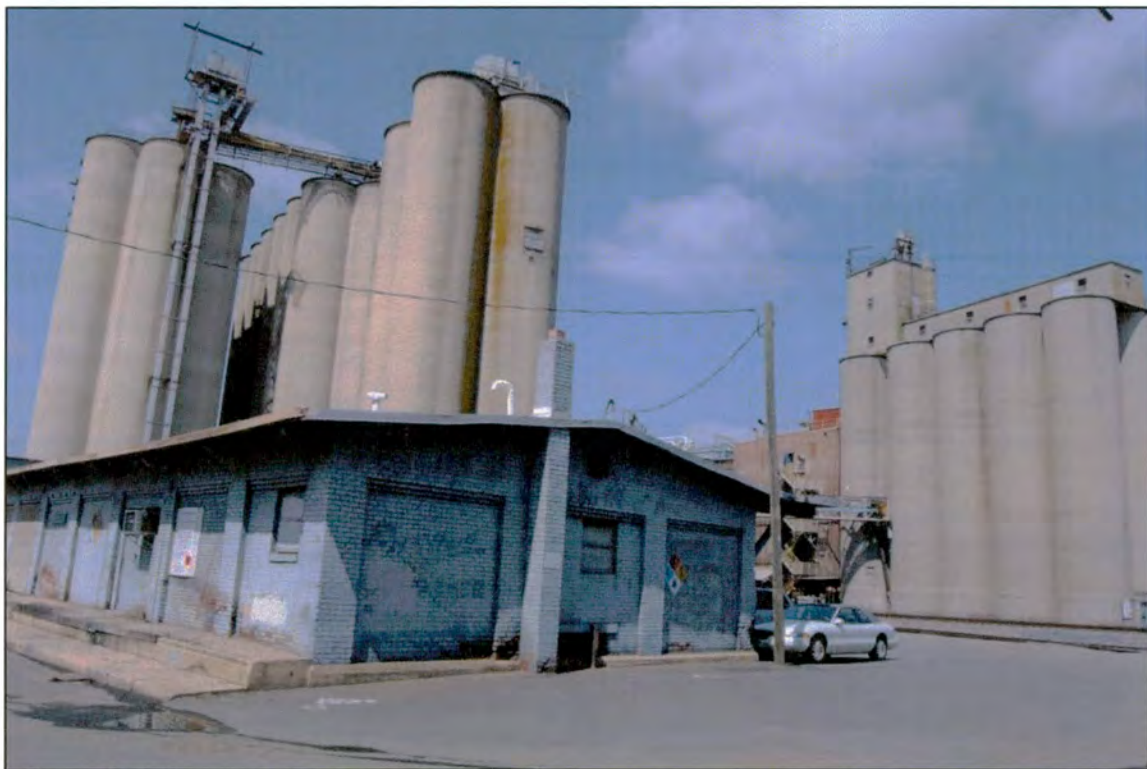
Interstate Mills complex from Smith Street
