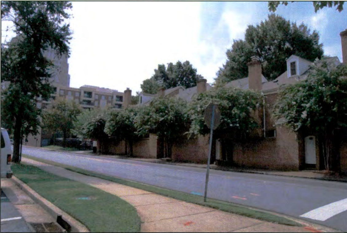
Fourth Ward Historic District—looking southeast on West 9th Street from North Poplar Street (southwest of APE)
