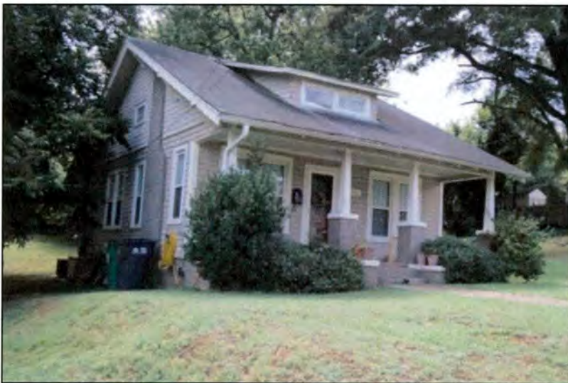
1325 W. 6th Street: East side and north front elevations
