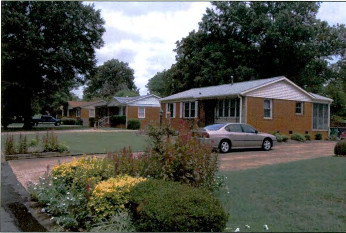
1236 Dean Street (1959), at right, (within APE)
