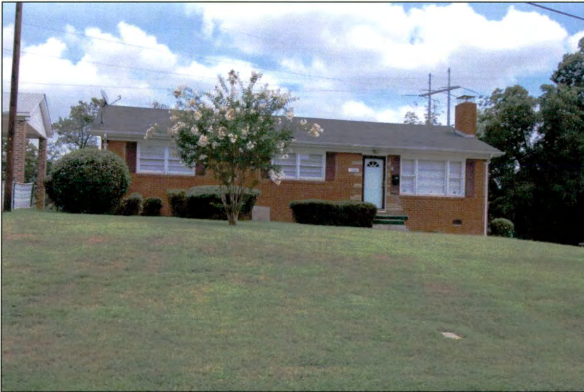
1500 Dean Street (1956) (within APE)
