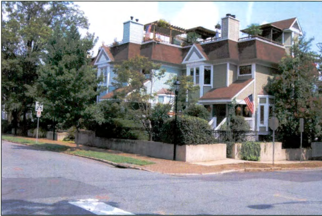
Fourth Ward Historic District—looking northwest on West 10th Street from North Poplar Street (toward APE)
