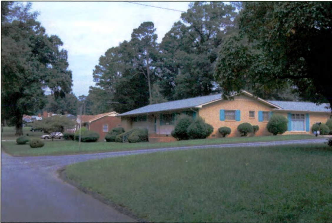
1624 Madison Avenue (1963) west of Creek Street (outside of APE within potential HD)
