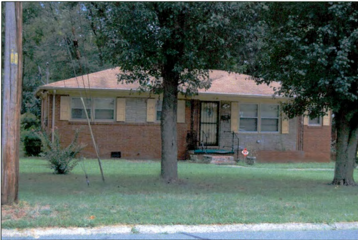
1330 Dean Street (1959) (within APE)
