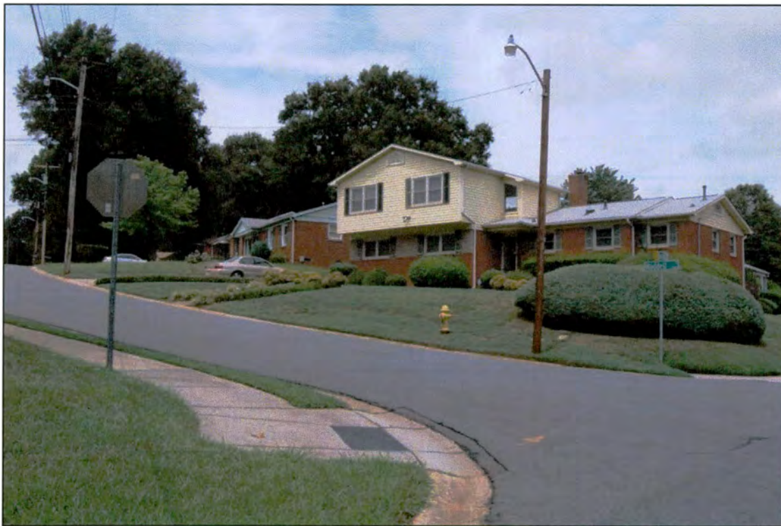
1400 Waddell Street (1958), at right, and 1410 Waddell (1957), at left, from Dean Street (within APE)
