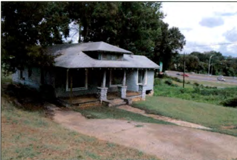
1322 W. 6th Street: West side and south front elevations; I-77 immediately to right
