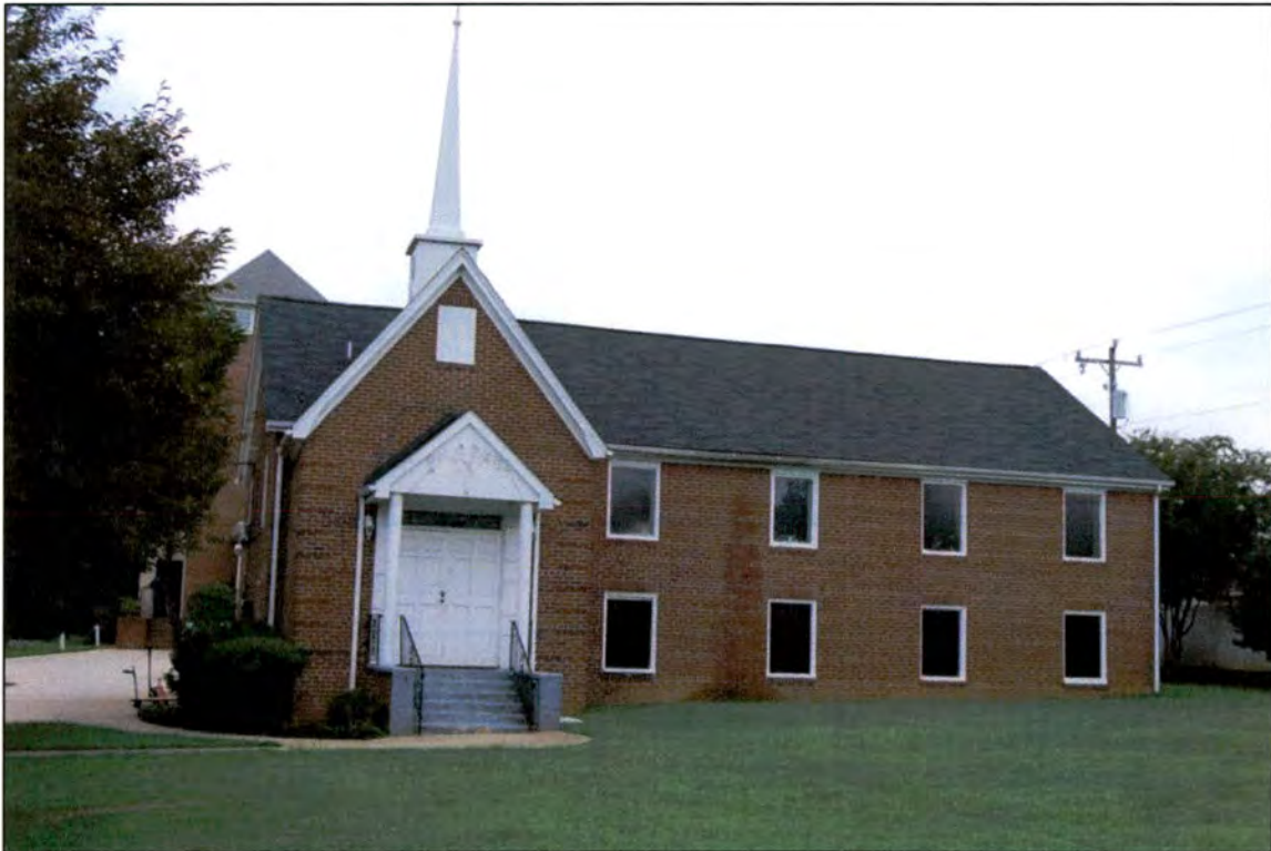
1800 Brewton Drive (1947) (within APE)
