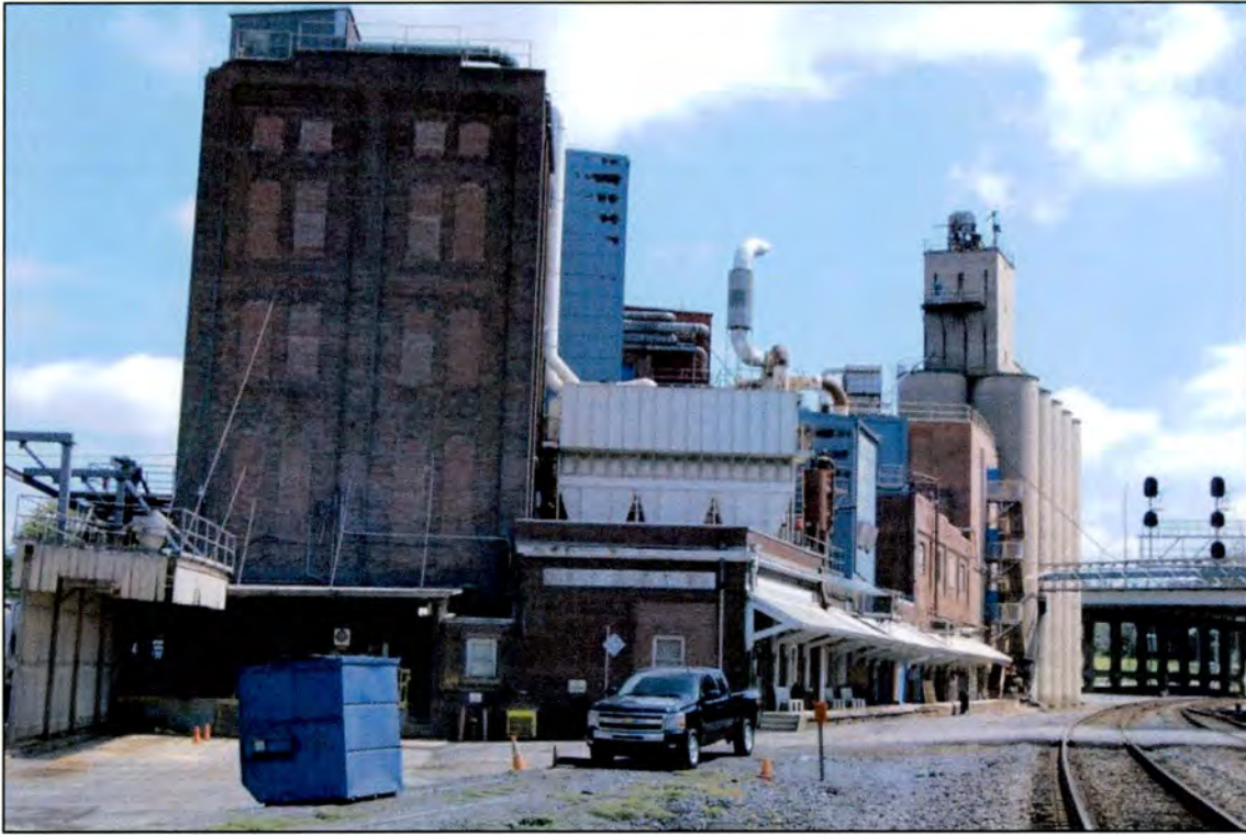
Interstate Mills complex on west side of tracks
