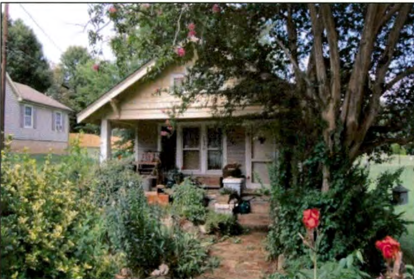
1330 W. 6th Street: South front elevations; modern 1334 W. 6th at left
