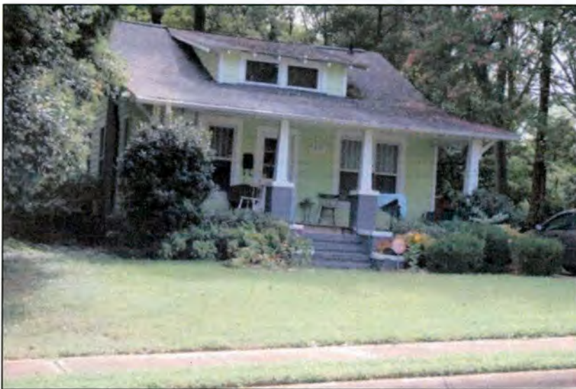
1315 W. 6th Street: East side and north front elevations
