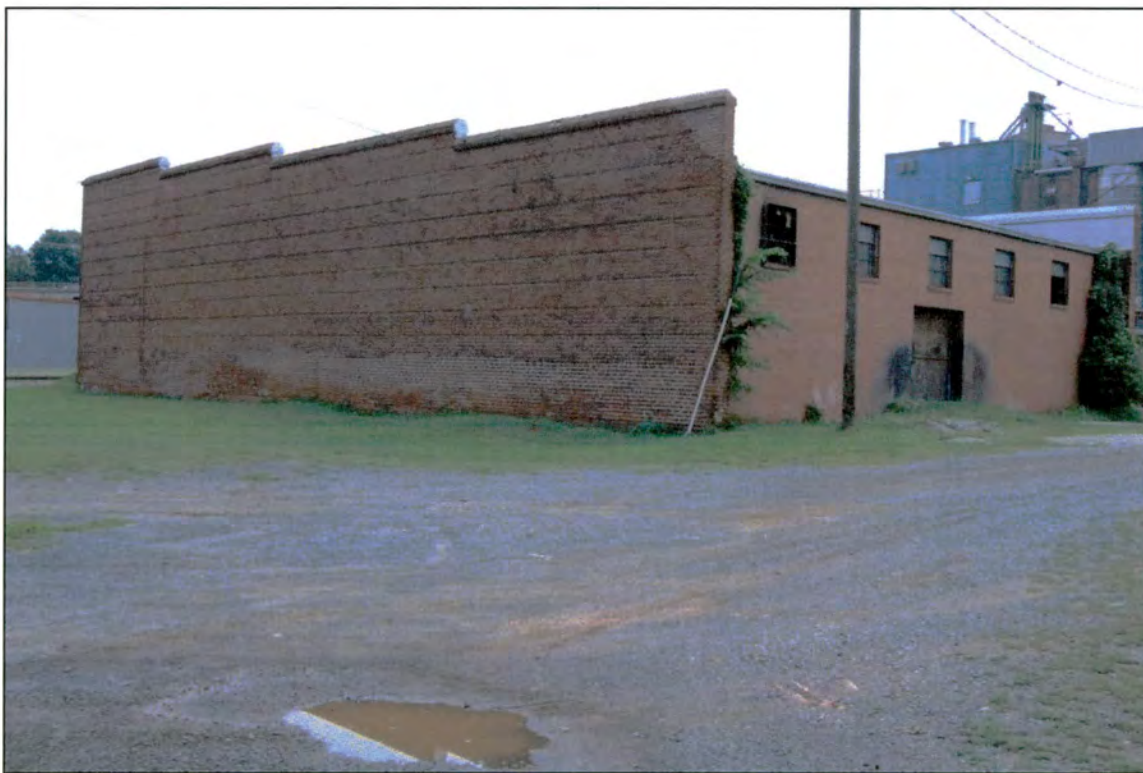
John B. Ross and Company Bag Warehouse
