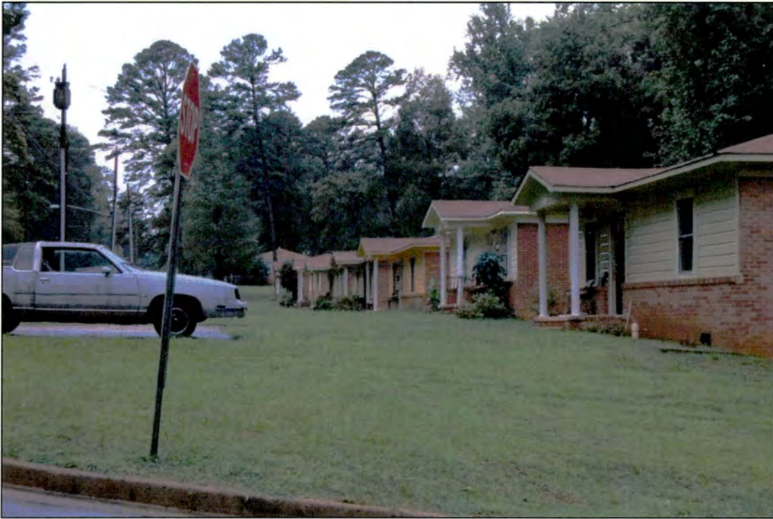
North side of Newland Road west of Lincoln Heights Court with 1704 Newland (1962) at right (outside of APE)
