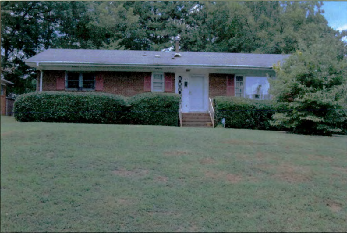
1600 Madison Avenue (1960) (within APE)
