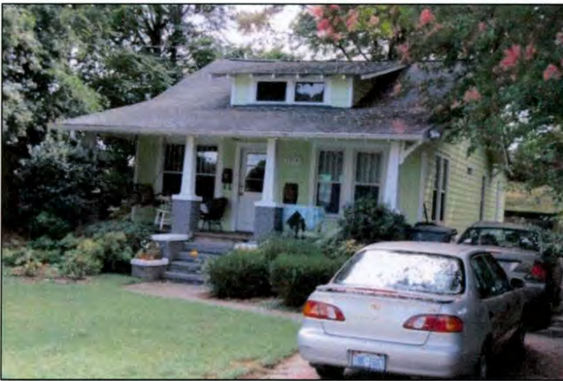
1315 W. 6th Street: West side and north front elevations
