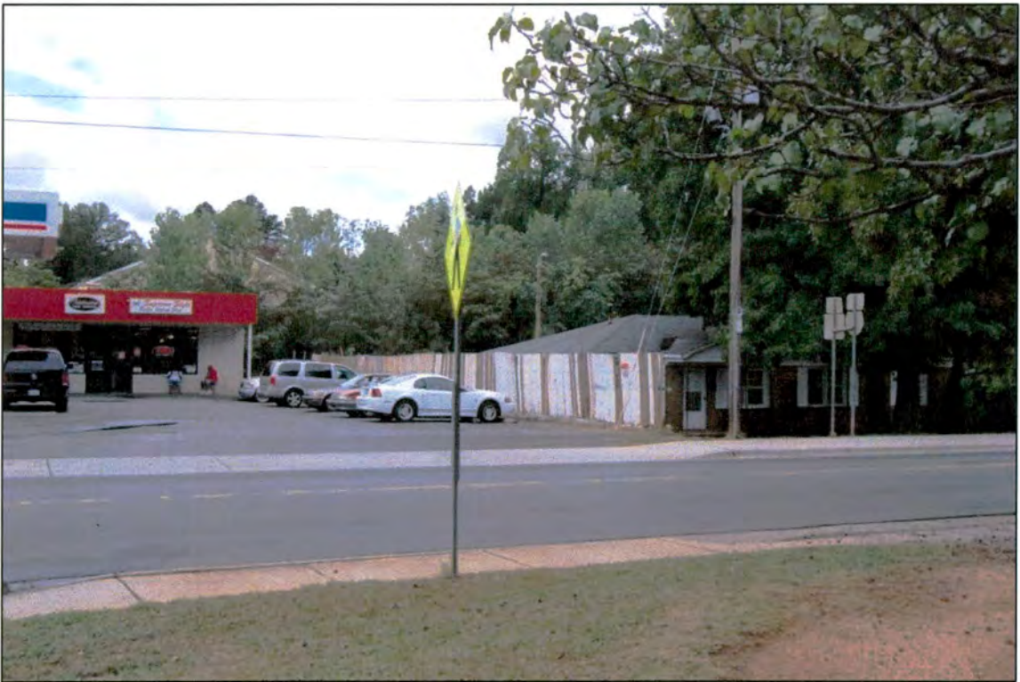
1327 Lasalle Street (1984, 1999), at left, and 1341 Lasalle Street (1963), at right (within APE)
